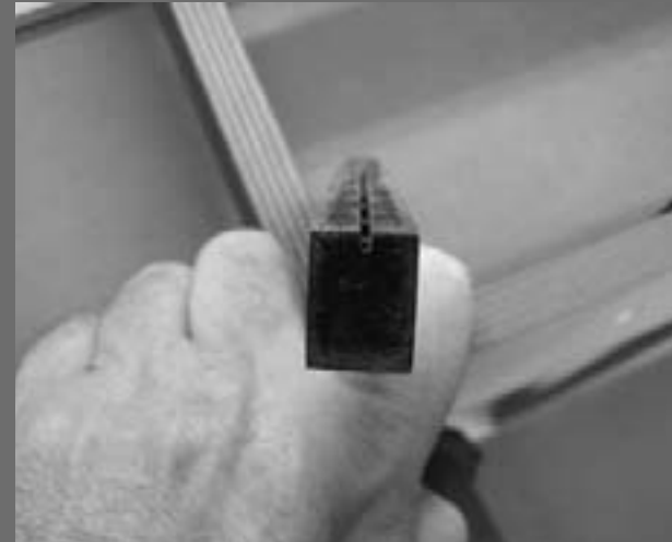
Figure 57: Slot cut 1/4" deep.
