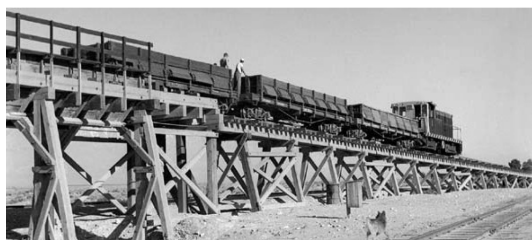
Figure 14: SP narrow gauge GE #1 works the ore trestle at Owneyo in 1955. The side-dump gondolas had an internal "A-frame" pitched floor to facilitate dumping into standard-gauge cars below. This view illustrates well the actual configuration of the high-line trestle. The layout compromises by having the standard gauge duck down because the narrow gauge can't climb enough in the space available. Looks like crews might have re-laid the narrow gauge track in the foreground (headed to Keeler) with some standard gauge ties. Courtesy, Joe Dale Morris Collection.
