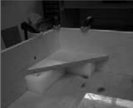
Figure 14: Gussets glued and screwed.
