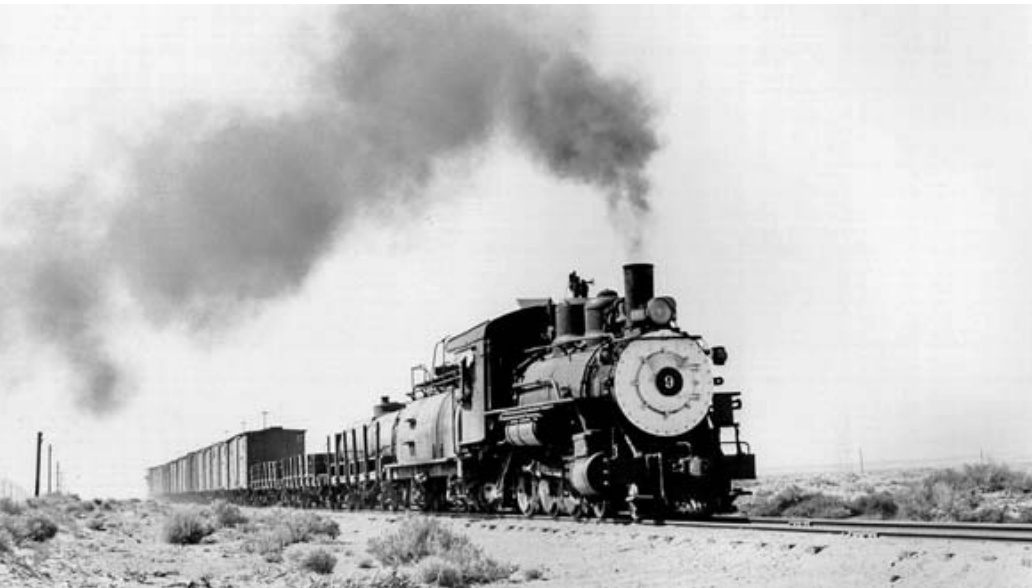
Figure 6: Number 9 has a long train rolling at speed across the high desert. Note the auxiliary water tender behind the regular tender, necessary for operation across the long, dry line. Courtesy, Joe Dale Morris Collection.
