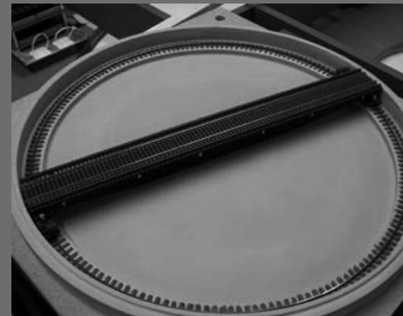
Figure 42: Completed pit with rail and turntable bridge.
