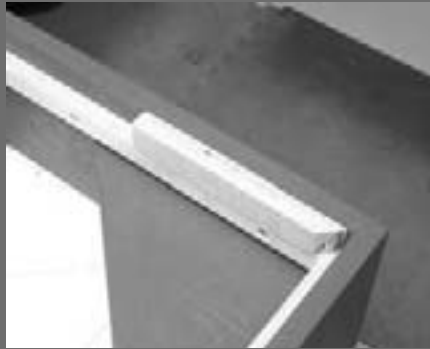
Figure 27: Sideframe cleats installed.
