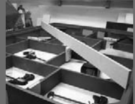
Figure 29: Installing and levelling the risers.
