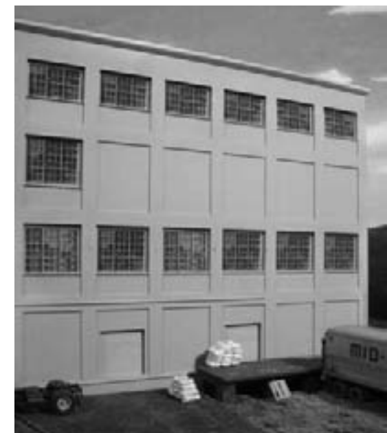
Figure 4: This photo shows some grey window frames that I think lack contrast and are not as realistic as some of the others, especially from a distance.
