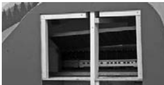
Figure 5: The side of the tunnel liner removed, giving access to the track and train inside the tunnel.
