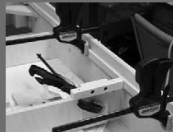
Figure 26: Cleats installed around the inside perimeter of the module.
