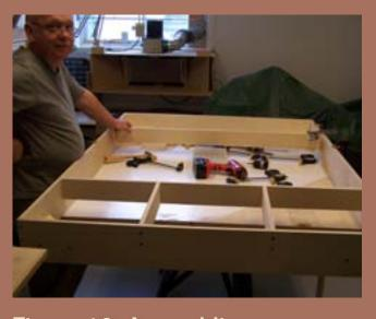
Figure 16: Assembling sideframe and gusset. I couldn't have assembled the module without Ray's help.
