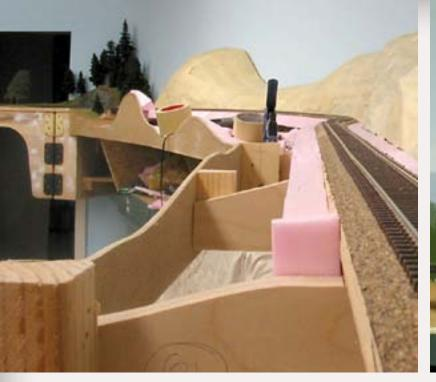
Figure 3: Charlie Comstock attaches his 3/16" masonite fascia to cleats at the end of the benchwork joists.
