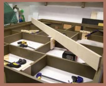
Figure 29: Installing and levelling the risers.
