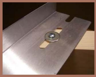
Figure 79: Securing mounting bracket.
