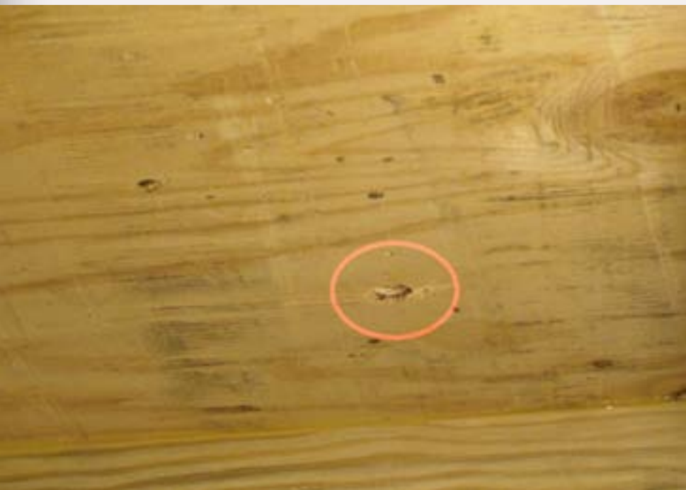
Figure 2: 1/2" hole drilled through plywood and foam for the control wire.
