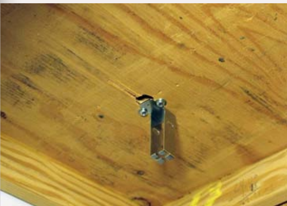
Figure 3: Servo bracket installed.
