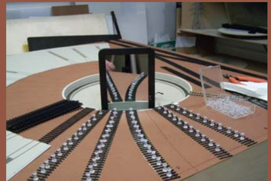
Figure 51: For curved tie strips, sight down using a mirror and adjust if necessary. Once completed let everything dry for several hours.
