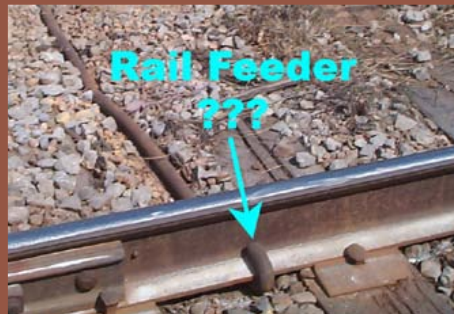
Figure 85: Prototype photo – gee this looks a lot like one of my rail feeders!
