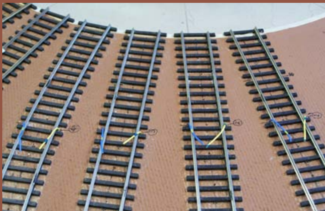
Figure 77: I left about 2 inches of feeder above the roadbed and stripped each wire,
