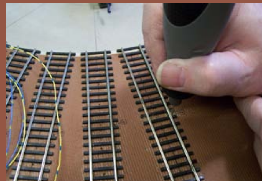
Figure 76: I drilled a hole close to each rail so the feeder would rest snug against the rail.
