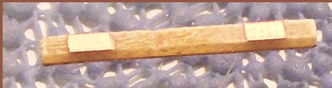
Figure 55: All that's left are the tie plates.
