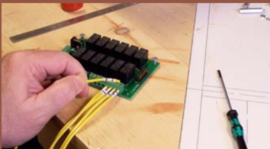
Figure 87: I had 21 wires going to the APR's, so I took the APR board and fastened it temporarily to my workbench. I routed, measured, numbered and cut each wire, then screwed it to the appropriate APR terminal.
