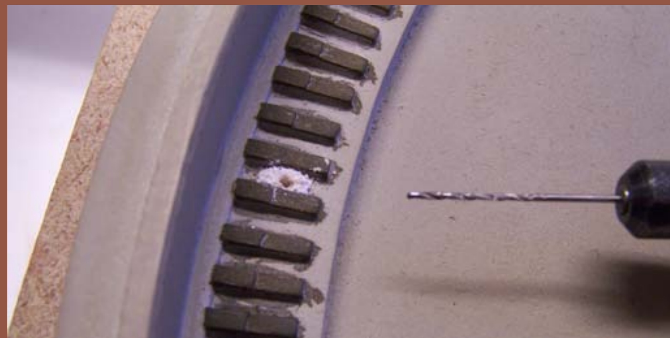
Figure 28: Tie recess for rail installation and hole drilled for feeder wire.
