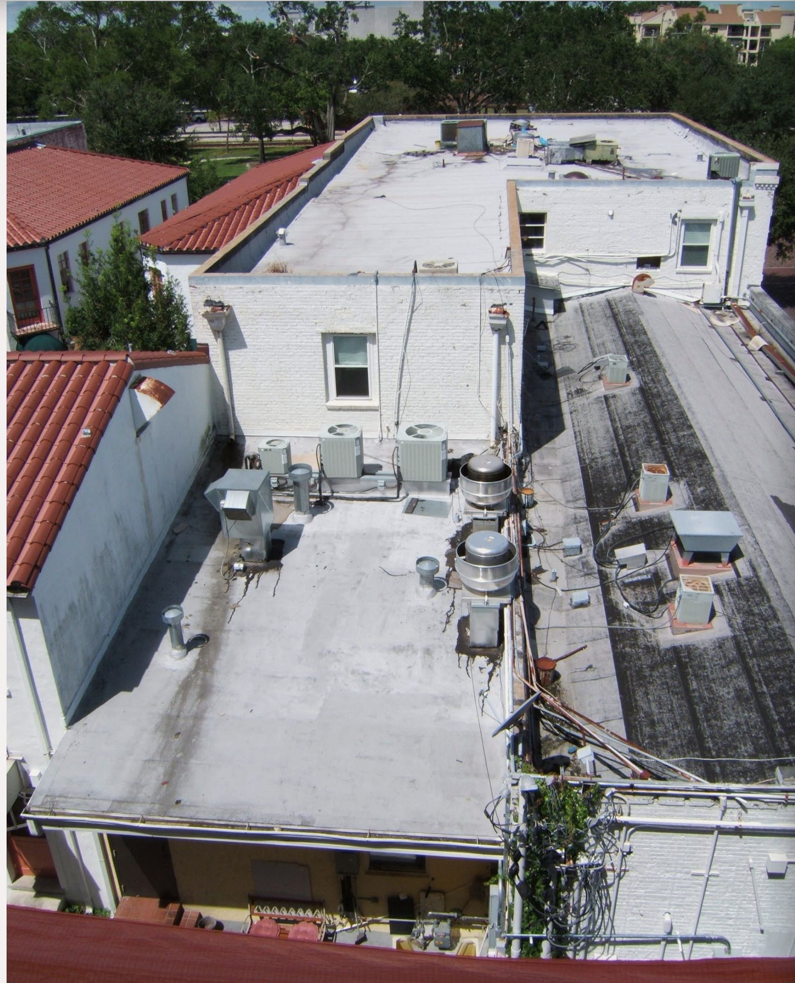
Figure 2: Typical commercial buildings. Each of these buildings exhibits a different roof type like tile and roll-down roofing. The roof on the right is a gable roof within a parapet wall on the end. From the ground, the roof looks flat.
