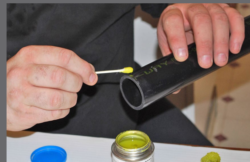
Figure 1.19: With a liberal coating of glue on the end of the pipe I prepared to install the cap. ABS glue sets fast, so positioning is a quick one-time procedure. No second chances here.
