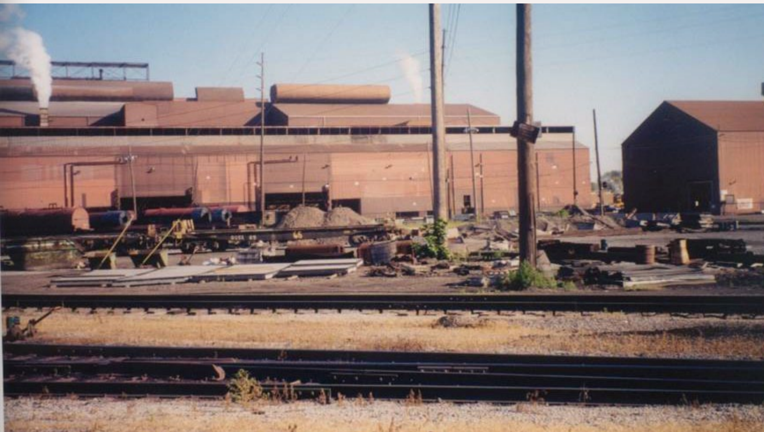
Figure 1: Typical industrial buildings. Notice the large ventilators that let out the heat from processes located inside the buildings.
