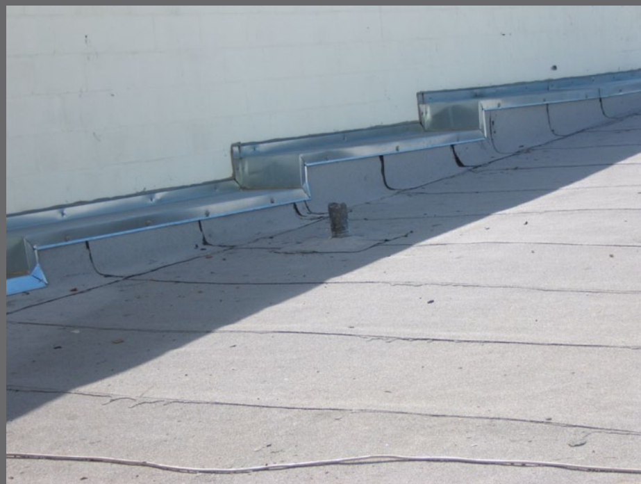
Figure 47: Prototype picture showing step flashing installed. Notice that the tar from the built up roof is not neat.
