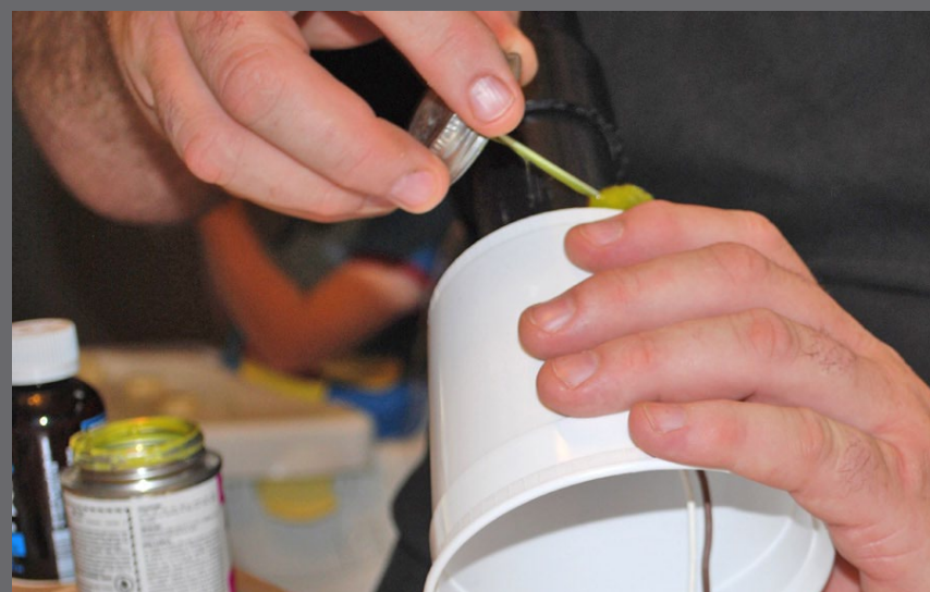
Figure 1.29: I swabbed glue onto the pipe where the coupler would sit.
