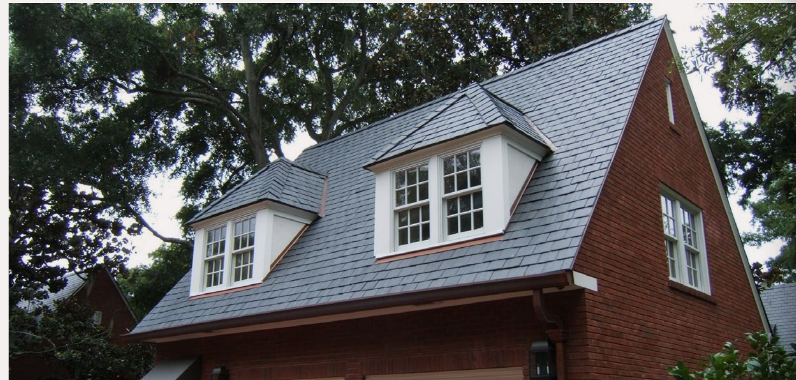
Figure 6: You won't find a slate roof used much in modern construction due to cost. A slate roof will last 50 years or more – this brand-new slate roof was installed to match the original house.
