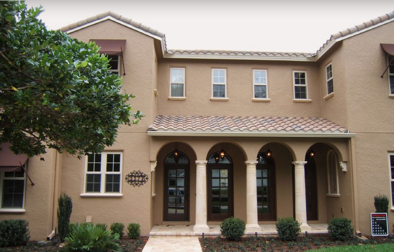
Figure 3: Typical residential building – a modern house with a tile roof.
