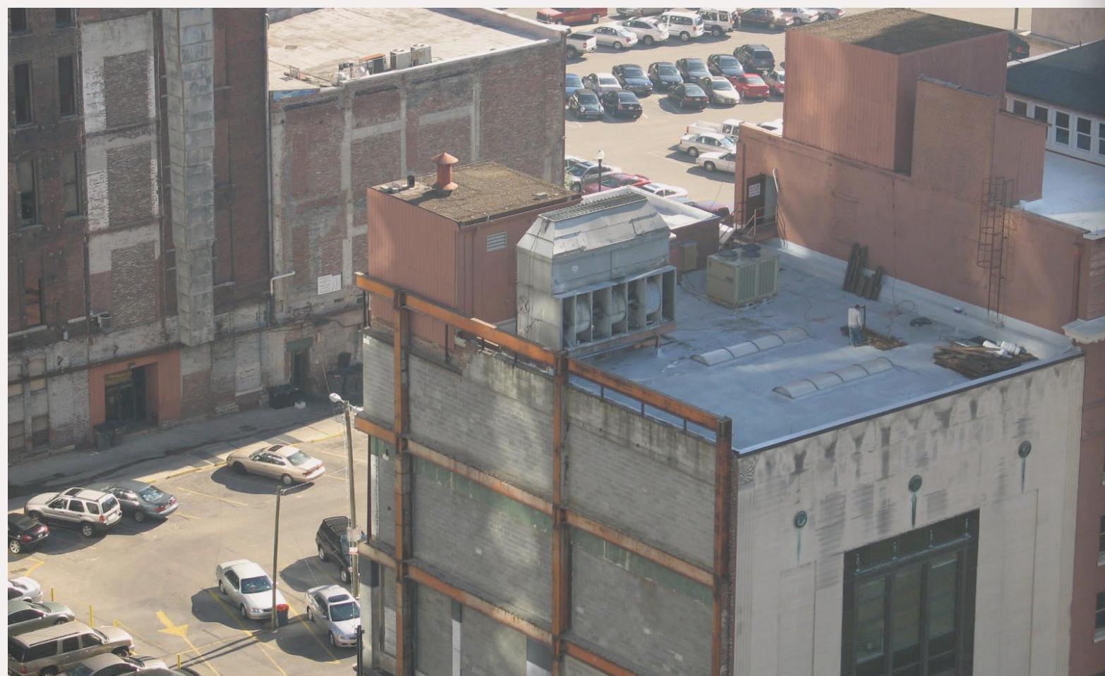
Figure 26: Another style of cooling tower.
