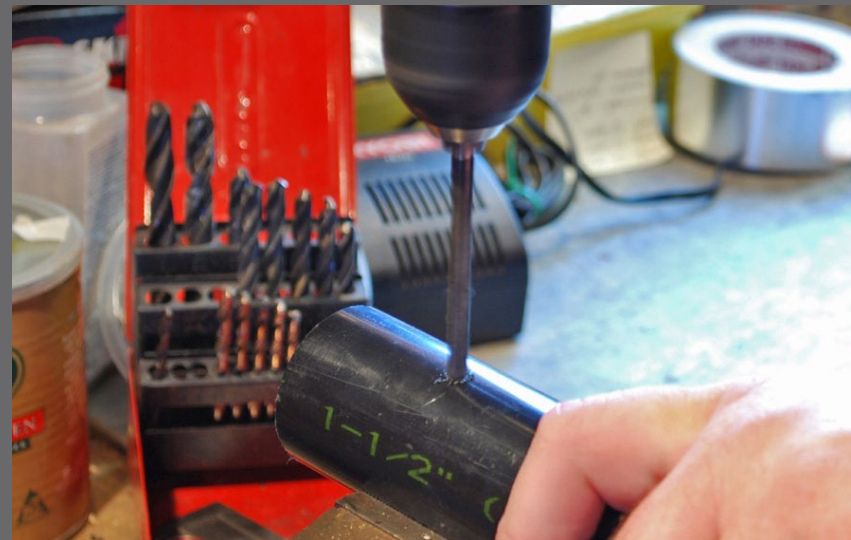
Figure 1.3: Using my cordless drill along with 1/8", 1/4" and a 1/2" bits, I drilled all the holes needed in the pipe.
