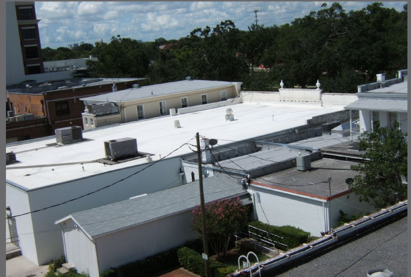
Figure 59: Notice the different roofing types and different elevations of the buildings.
