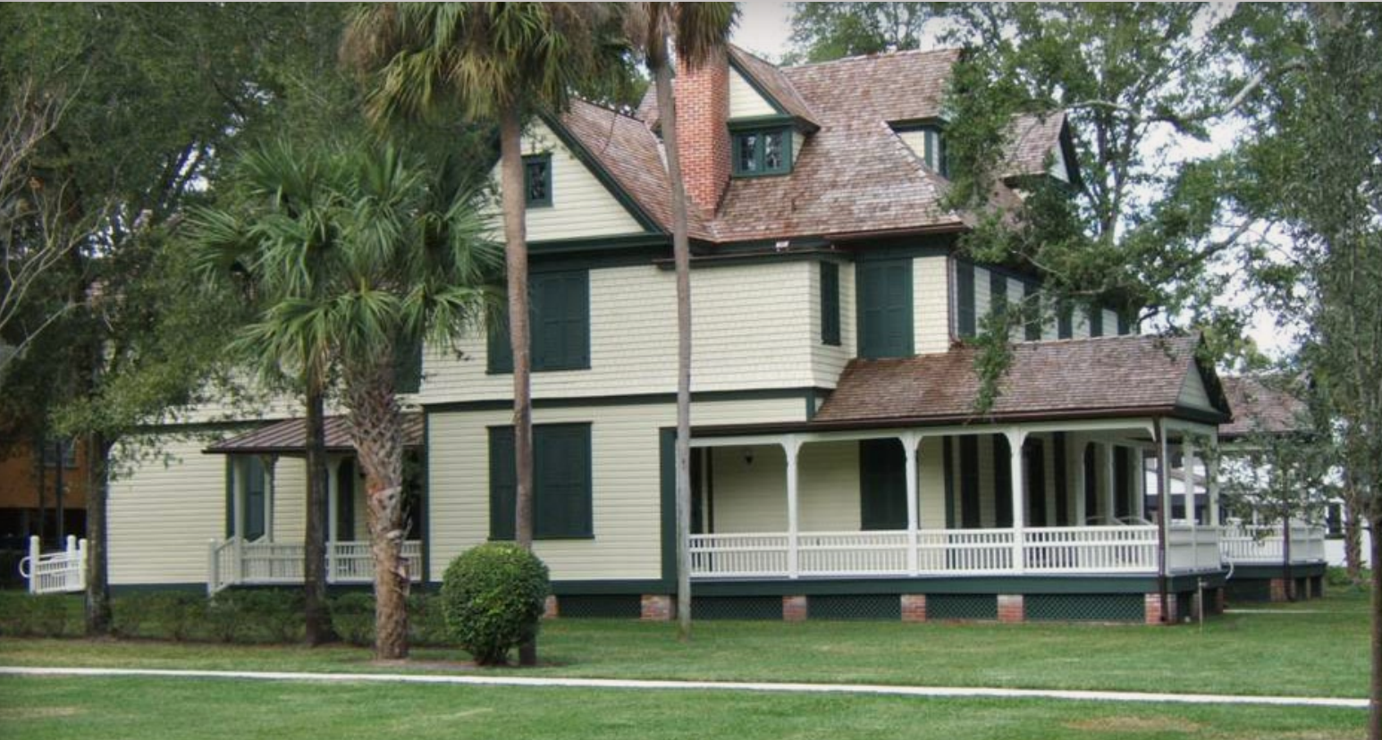
Figure 7: Wood shake roofing is not used much any more. This is a historic house that was restored within the last few years. The new wood shake roof was installed for historic reasons.
