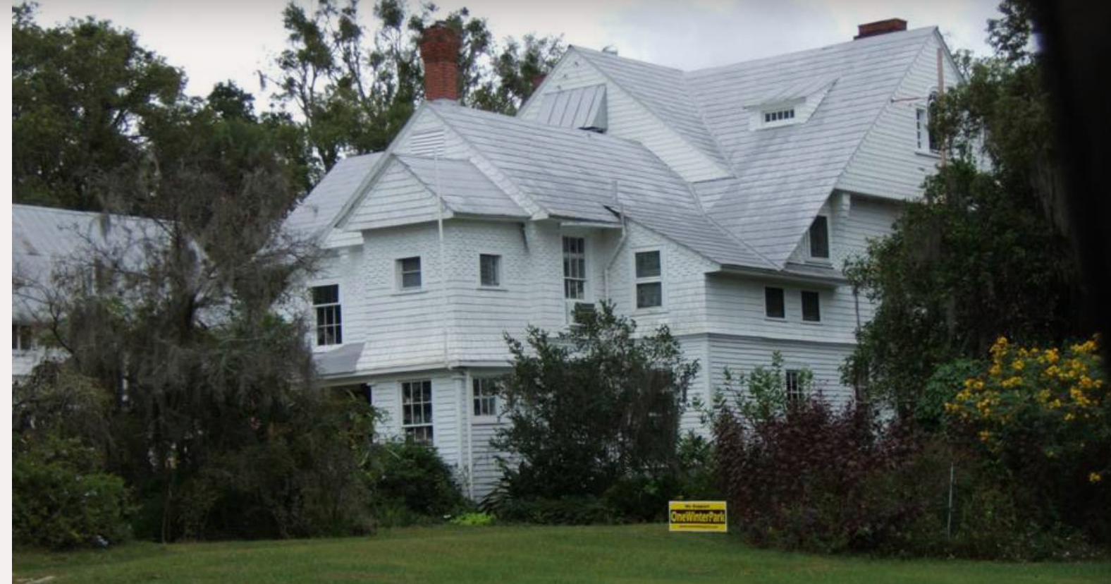
Figure 8: This house has a metal-stamped roof . Normally you will see the corrugated type or the standing-seam type. This style was made to look like shingles, but being metal gives better fire protection than shingles.
