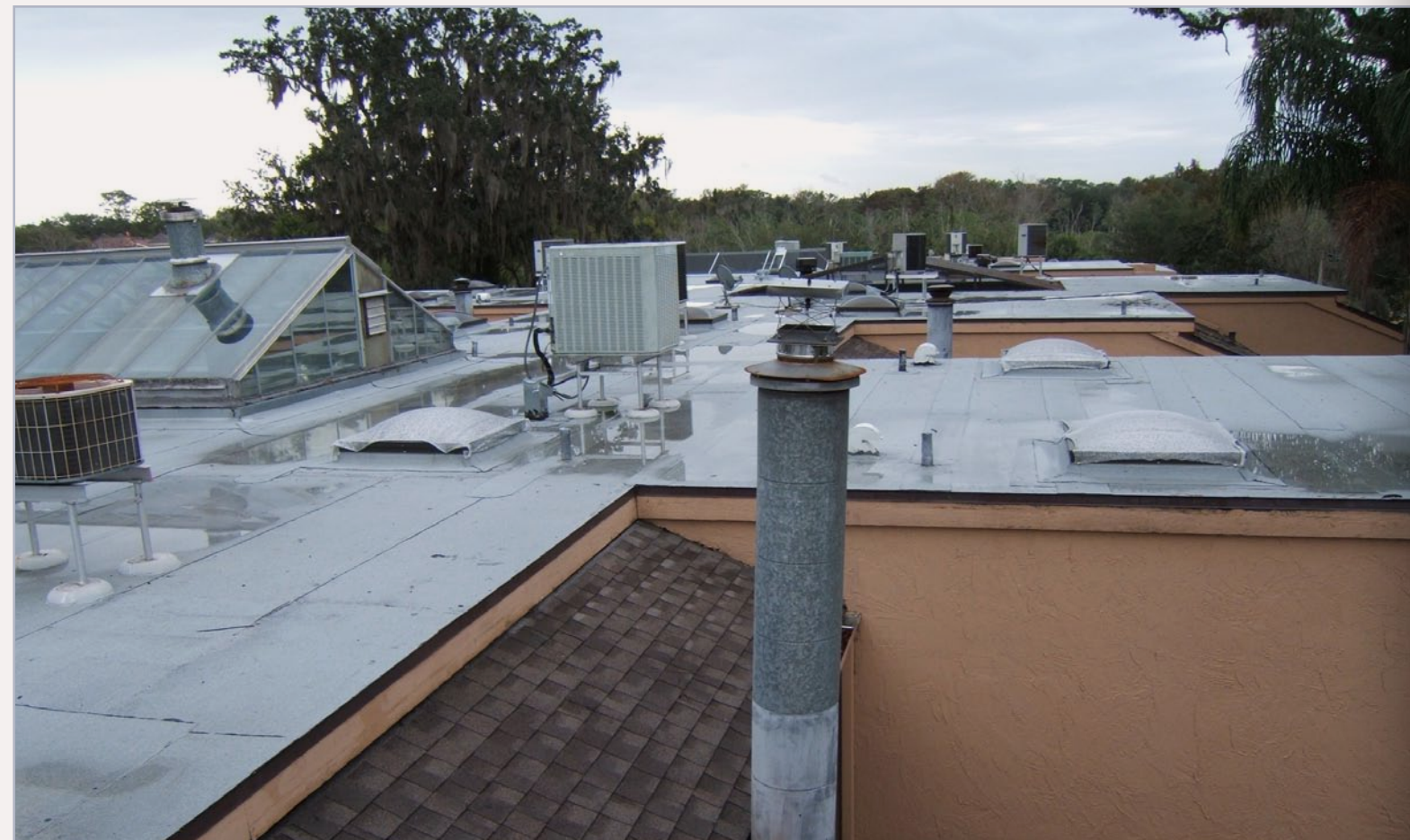
Figure 23: This house roof has a greenhouse. That big gray pipe in the foreground is a vent from a wood-burning fireplace.
