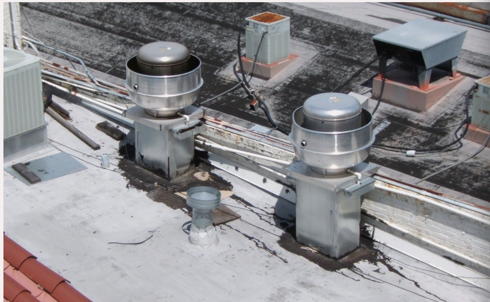
Figure 19: These two cooking-pot like vents are up blast grease exhaust fans. These units tilt so they can be cleaned. They stand 40" from the roof surface to the top of the fan.
