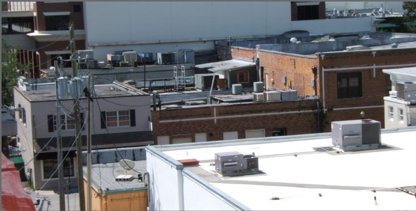
Figure 58: Typical main street blocks of stores that were built in the 1920s and modified to meet today's standards. The different roof heights, materials, and equipment makes it very appealing to try to model this – instead of just having nothing much on your roofs.
