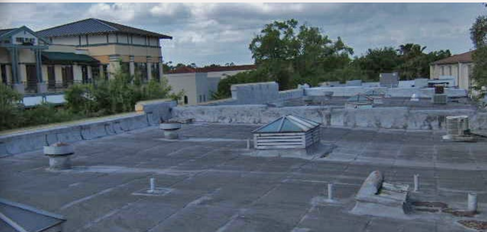
Figure 22: Typical roof details as seen from 1920 through today. This roof has old-style skylights installed (Campbell Scale Models and Grandt Line make this style of skylights). This roof also has old-style roof ventilators with very noticeable weathered streaking. The galvanizing on the smaller pipe ventilators keeps them from exhibiting such strong streaking.
