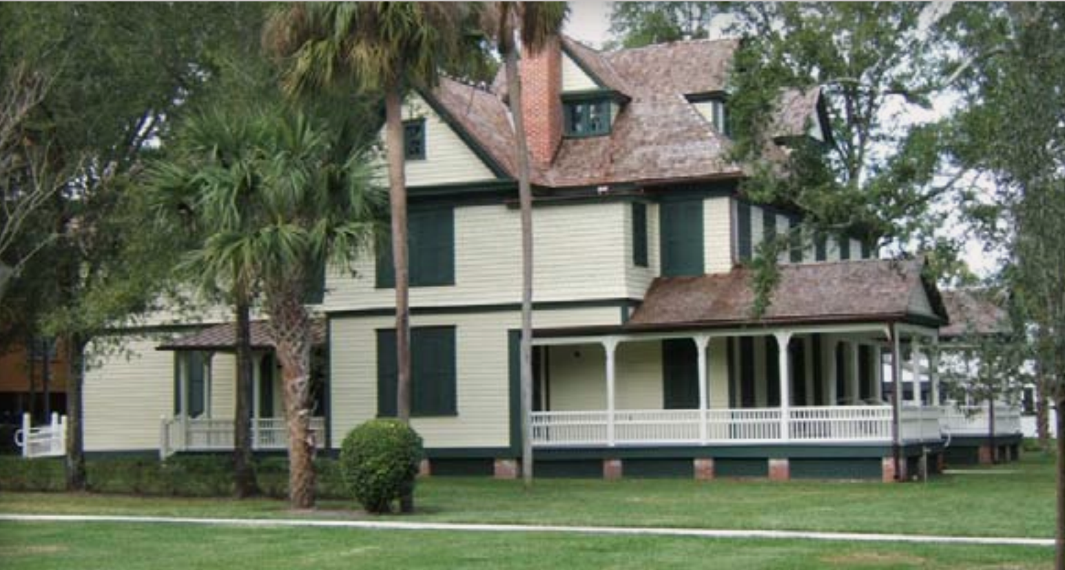
Figure 7: Wood shake roofing is not used much any more. This is a historic house that was restored within the last few years. The new wood shake roof was installed for historic reasons.
