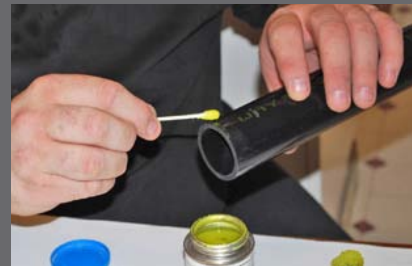
Figure 1.19: With a liberal coating of glue on the end of the pipe I prepared to install the cap. ABS glue sets fast, so positioning is a quick one-time procedure. No second chances here.
