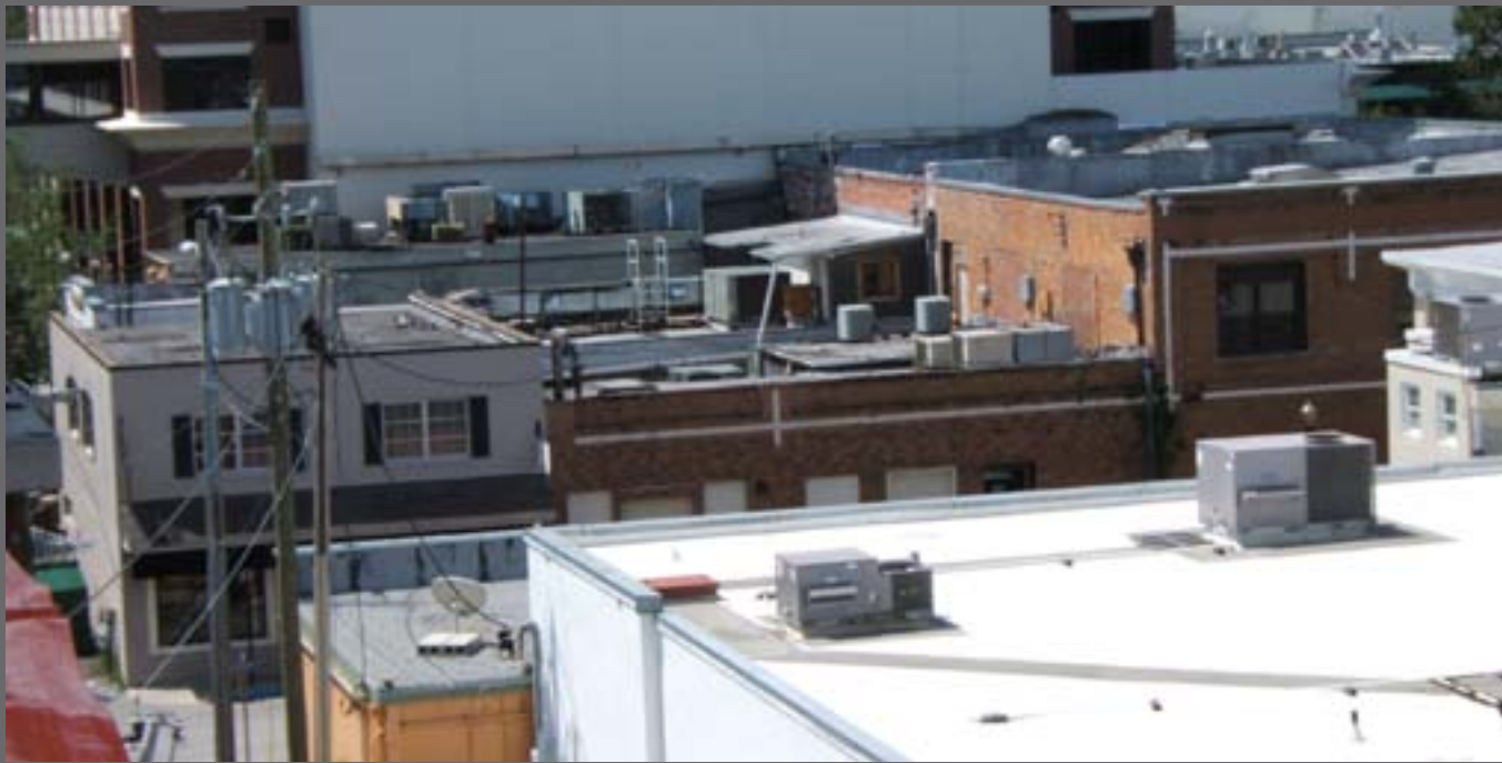
Figure 58: Typical main street blocks of stores that were built in the 1920s and modified to meet today's standards. The different roof heights, materials, and equipment makes it very appealing to try to model this – instead of just having nothing much on your roofs.
