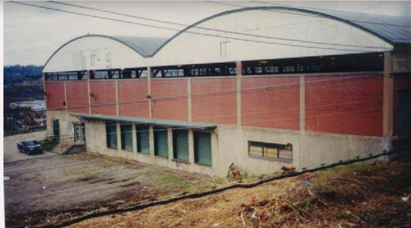
Figure 4: This barrel type roof is not as commonly seen, and can be something of a challenge to model. This building is next to Rook Yard of the Wheeling and Lake Erie RR in Pittsburgh.
