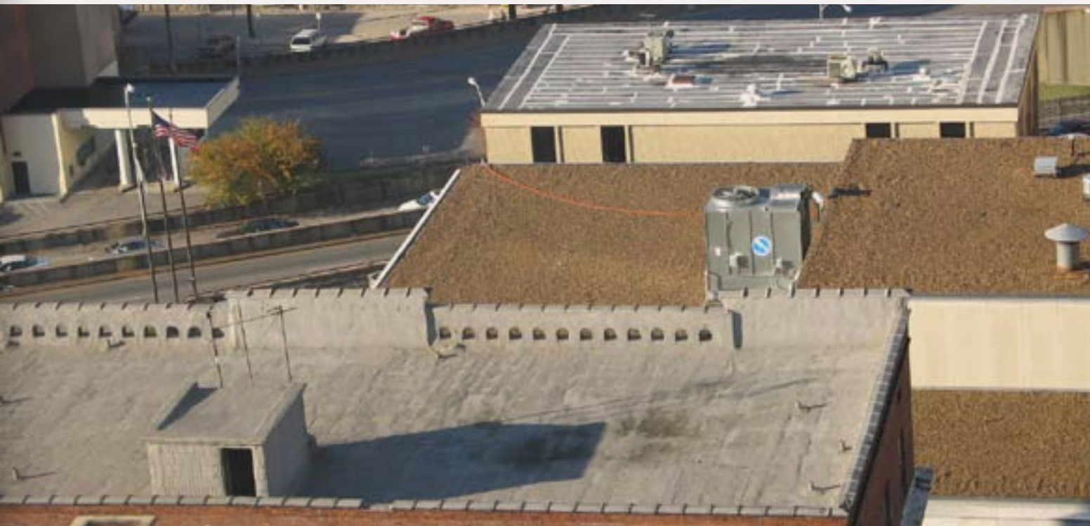
Figure 5: Here's a combination of different roof types from front to back: roll-down and tar-and-gravel. On the front building, notice the antenna on the roof access and the tile caps on the roof edge. A new cooling tower has been added to the second building's roof. On the rear building, repairs have been made to the roof.
