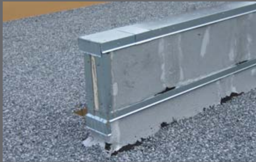
Figure 46: Prototype picture of straight wall section with flashing installed.
