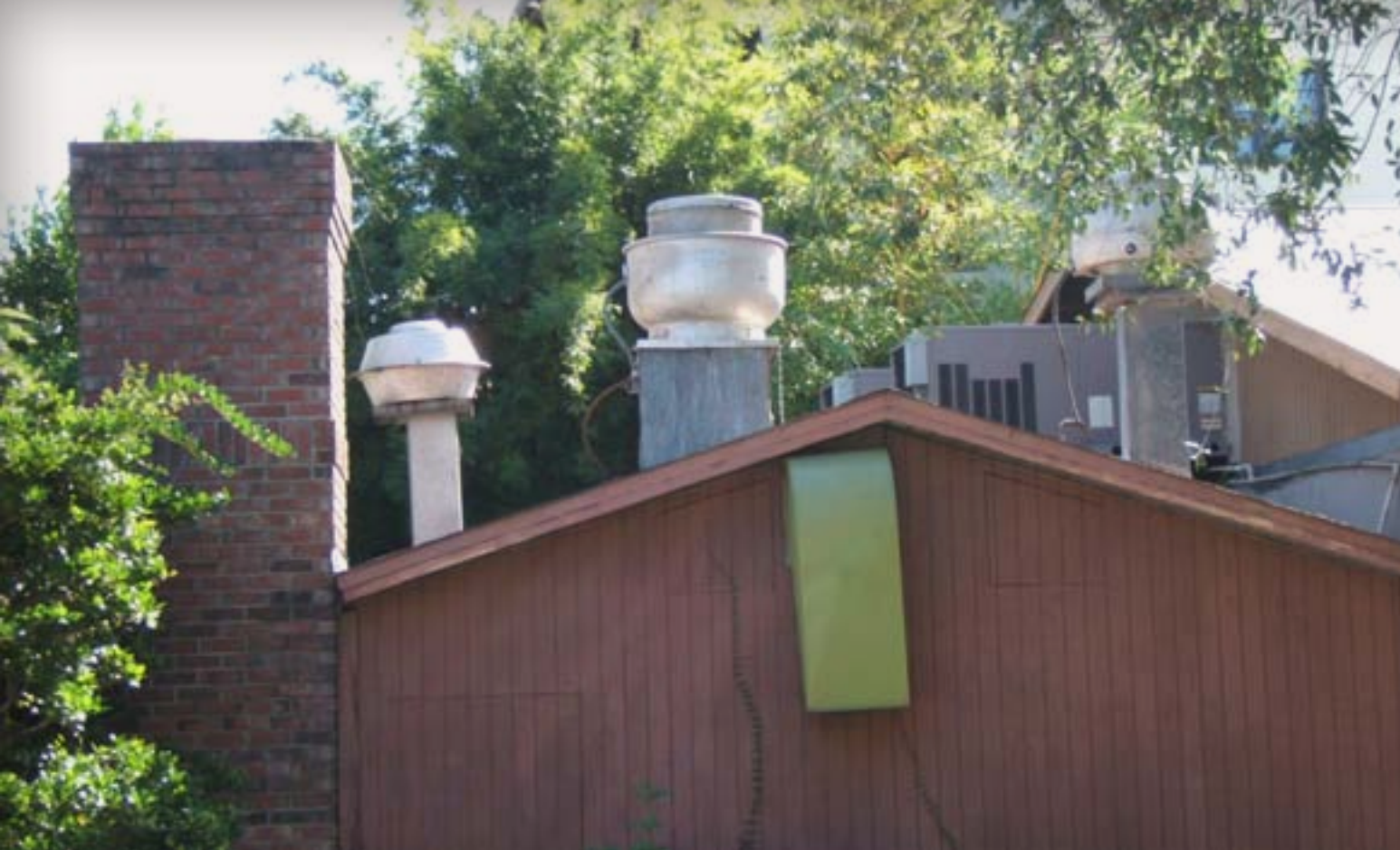
Figure 20: Multiple grease exhaust fans on the roof, with a makeup air duct on the wall (green ductwork).
