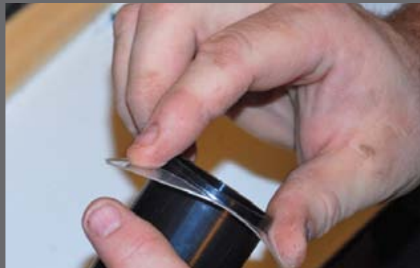
Figure 1.24: I test-fit the plastic washer on the pipe end.
