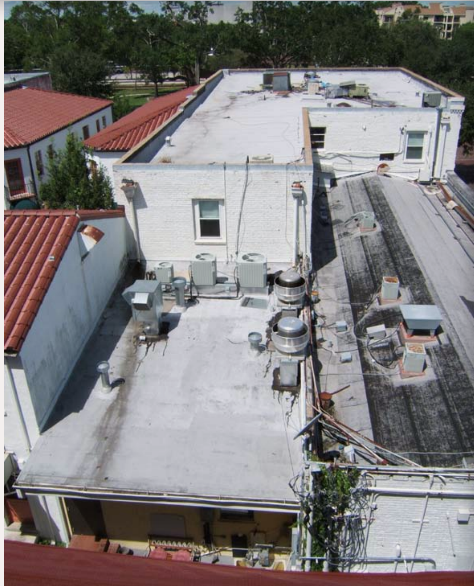
Figure 2: Typical commercial buildings. Each of these buildings exhibits a different roof type like tile and roll-down roofing. The roof on the right is a gable roof within a parapet wall on the end. From the ground, the roof looks flat.
