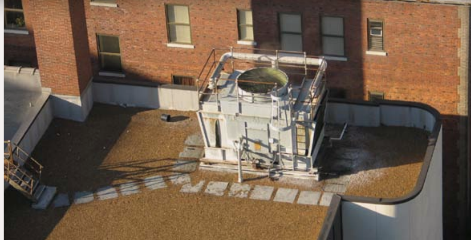
Figure 25: This a picture of a cooling tower. Piping coming out of the front goes to the chiller located in the building. Electrical disconnect switches are for the fan. The walkway pads protect the roof and the walkway stairs make it easy to access the unit for servicing.
