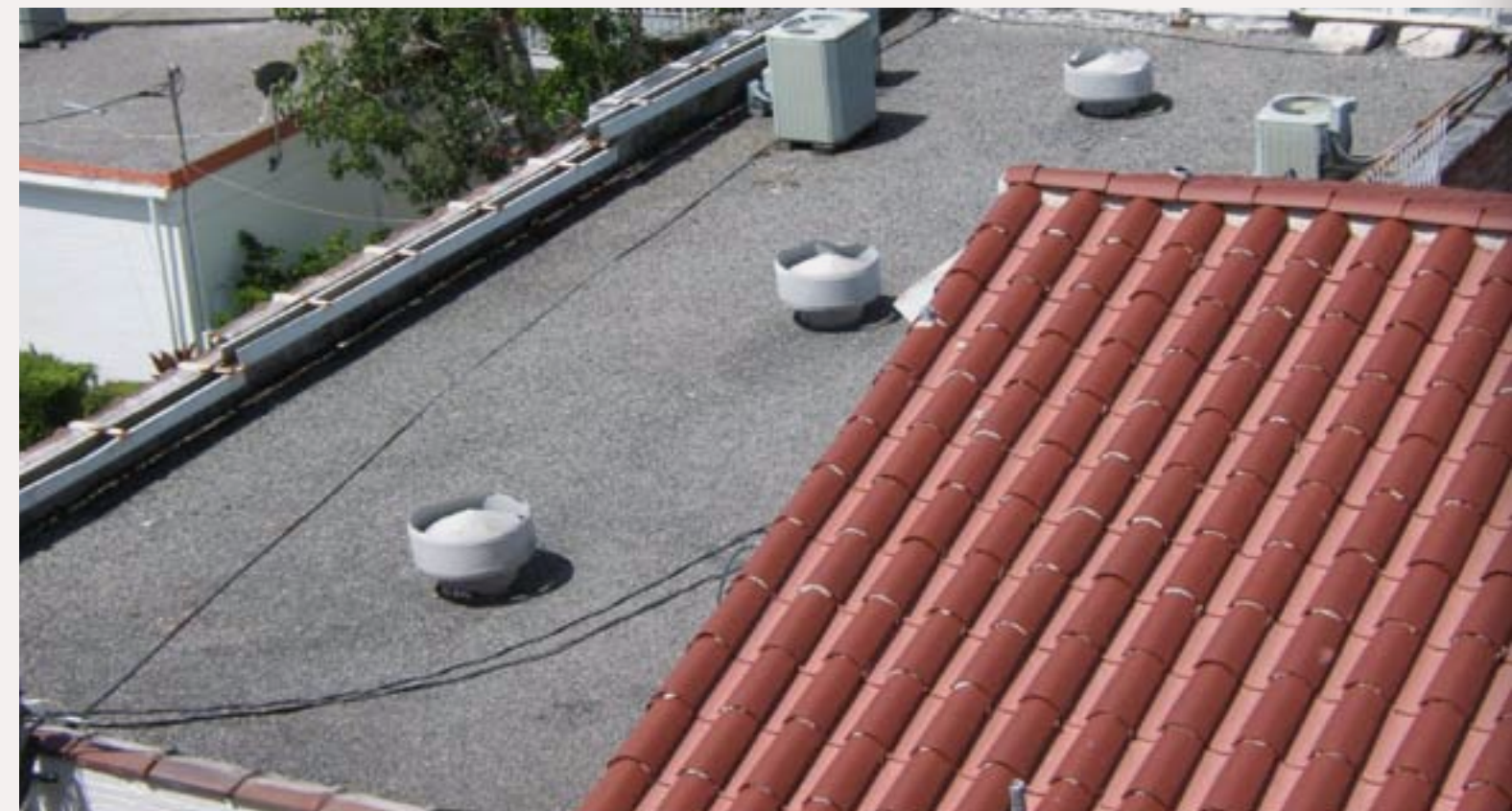
Figure 10: These are typical roof ventilators for a commercial flat roof. They let the heat escape from the attic. Notice the roof heights and types of roofing, and even the tree growing between buildings. Modeling these details from photos will enhance the scenes on your model railroad.
