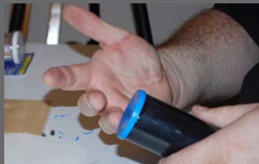
Figure 1.20: Firm downward pressure and a small twisting motion are all it took to firmly seat the cap in place, flush against the end of the pipe.
