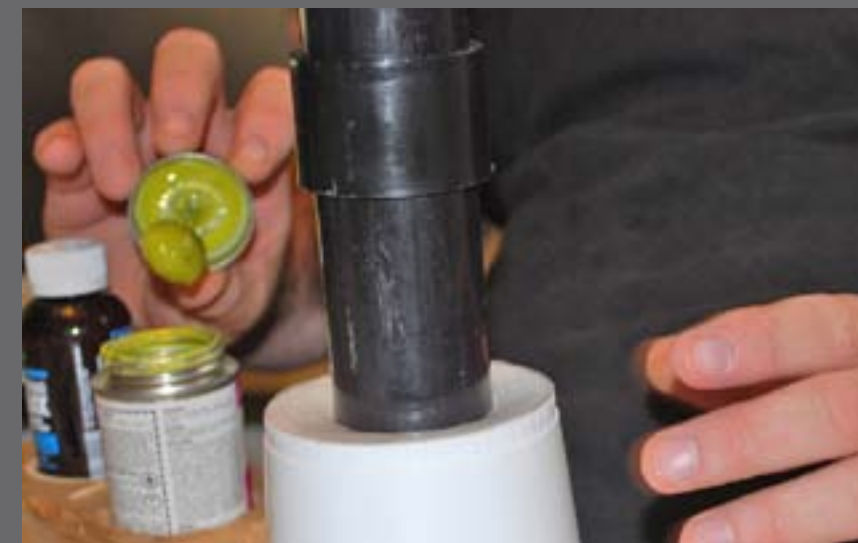
Figure 1.28: I slid the coupler over the pipe in preparation for gluing.
