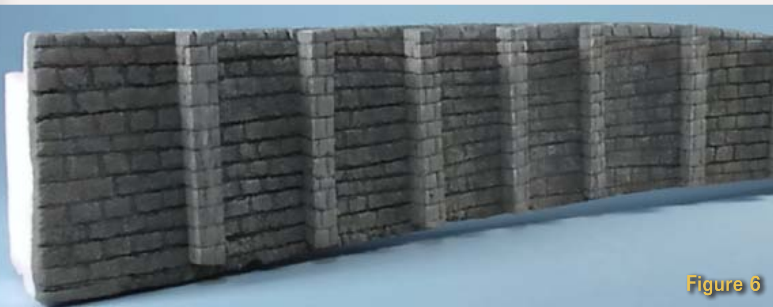
Figures 6 and 7: The retaining wall ready for the top cap and after top cap installation with dry-brushed highlights.
