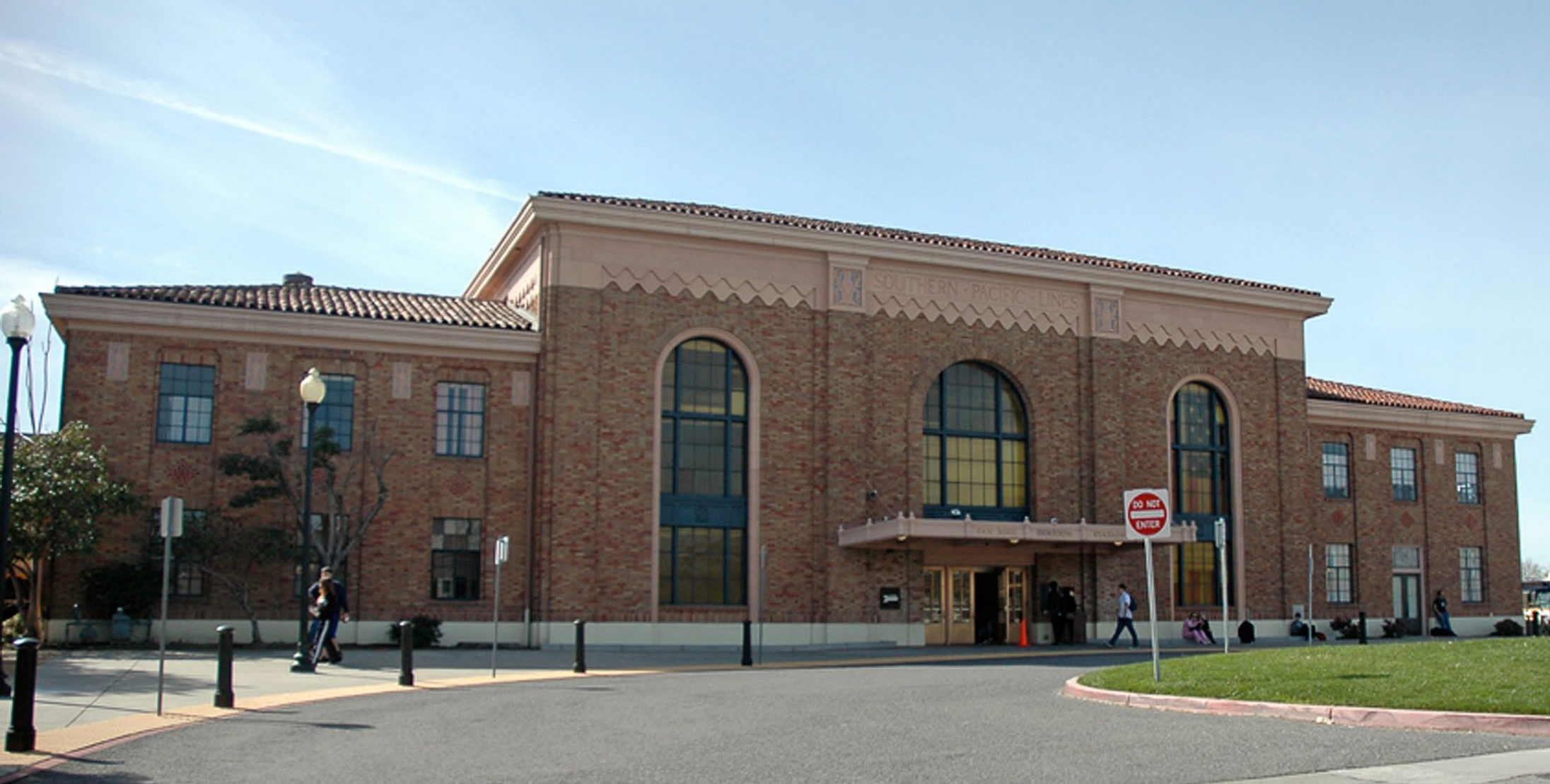
Figure 36: The current San Jose station. The SP opened it in 1935 after a massive relocation of railroad tracks from the middle of 4th Street. SP architect John Christie designed the building in the Italian Renaissance Revival style. It's similar to the Sacramento station with its large arched windows. The 40 x 80 main building is steel framed, and wings are framed with wood, all clad with variegated blonde brick laid in English Bond pattern. Its total length including the mail and express wing on the left is 390 feet - Craig Walker photo .
