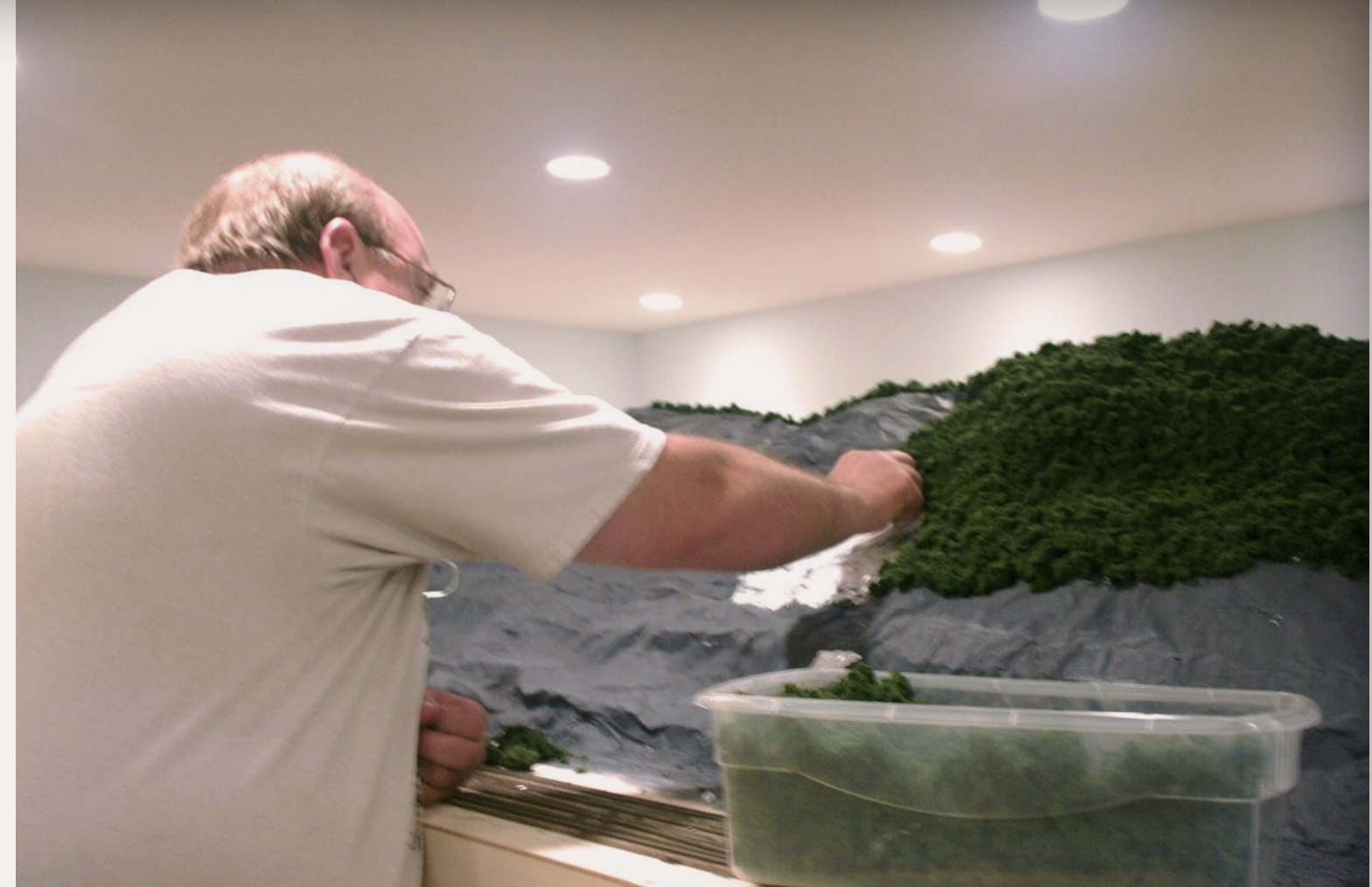
FIGURE 7: Here, Mark Andersen, one of the construction crew, plants a few acres above MG Tower. The adhesive caulk is still white in this picture, but will turn clear when it dries.
