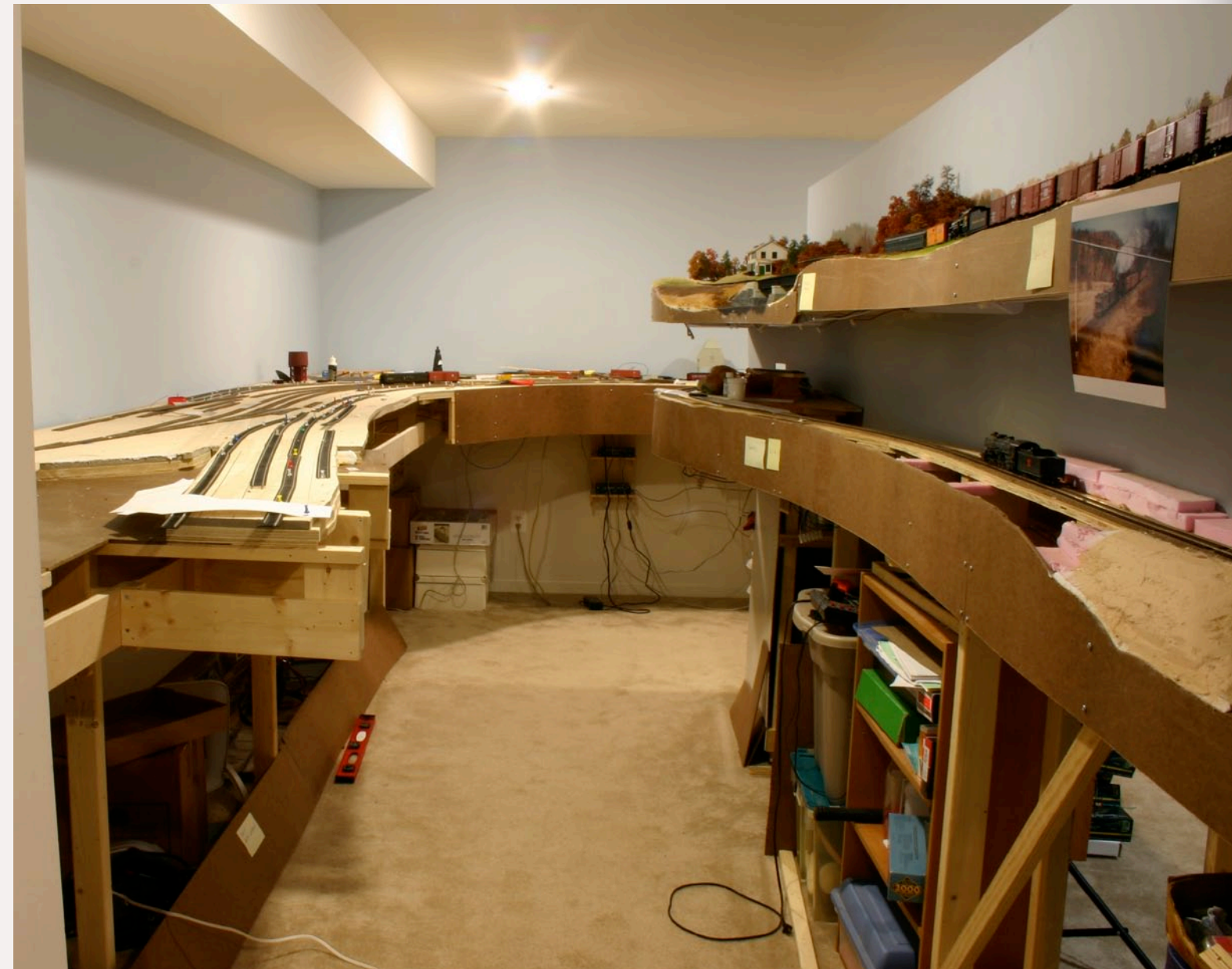
FIGURE 1: During test operating sessions (see Sea Trials for the SNE in the May/June 2010 MRH ) the Thames Street pier area protruded into the aisle and proved a bottleneck for operators entering the layout area. So Marty decided to rework the pier area – again.
