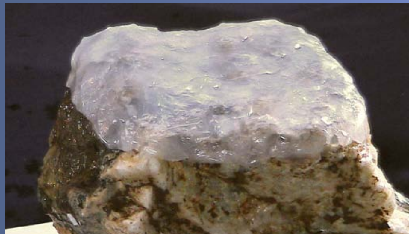
Figure 5. First layer of silicone smoothed out.
