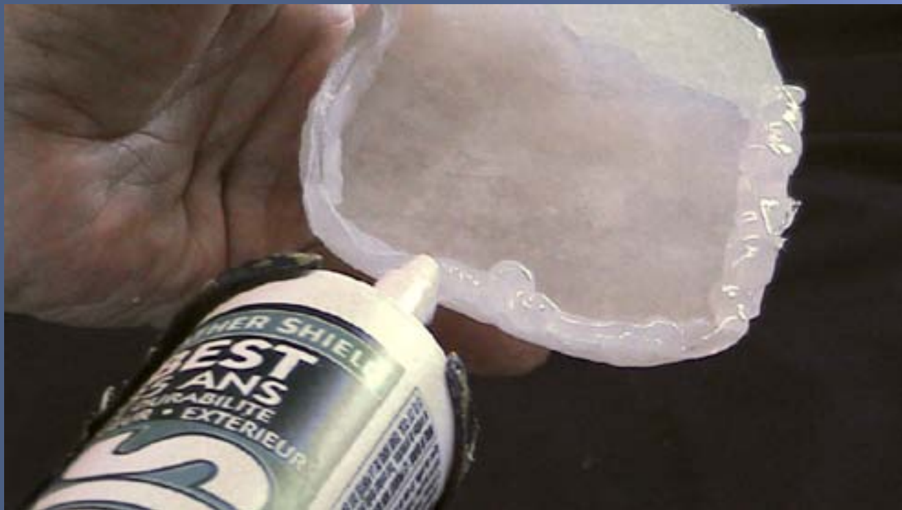
Figure 9. Applying the edge bead.
