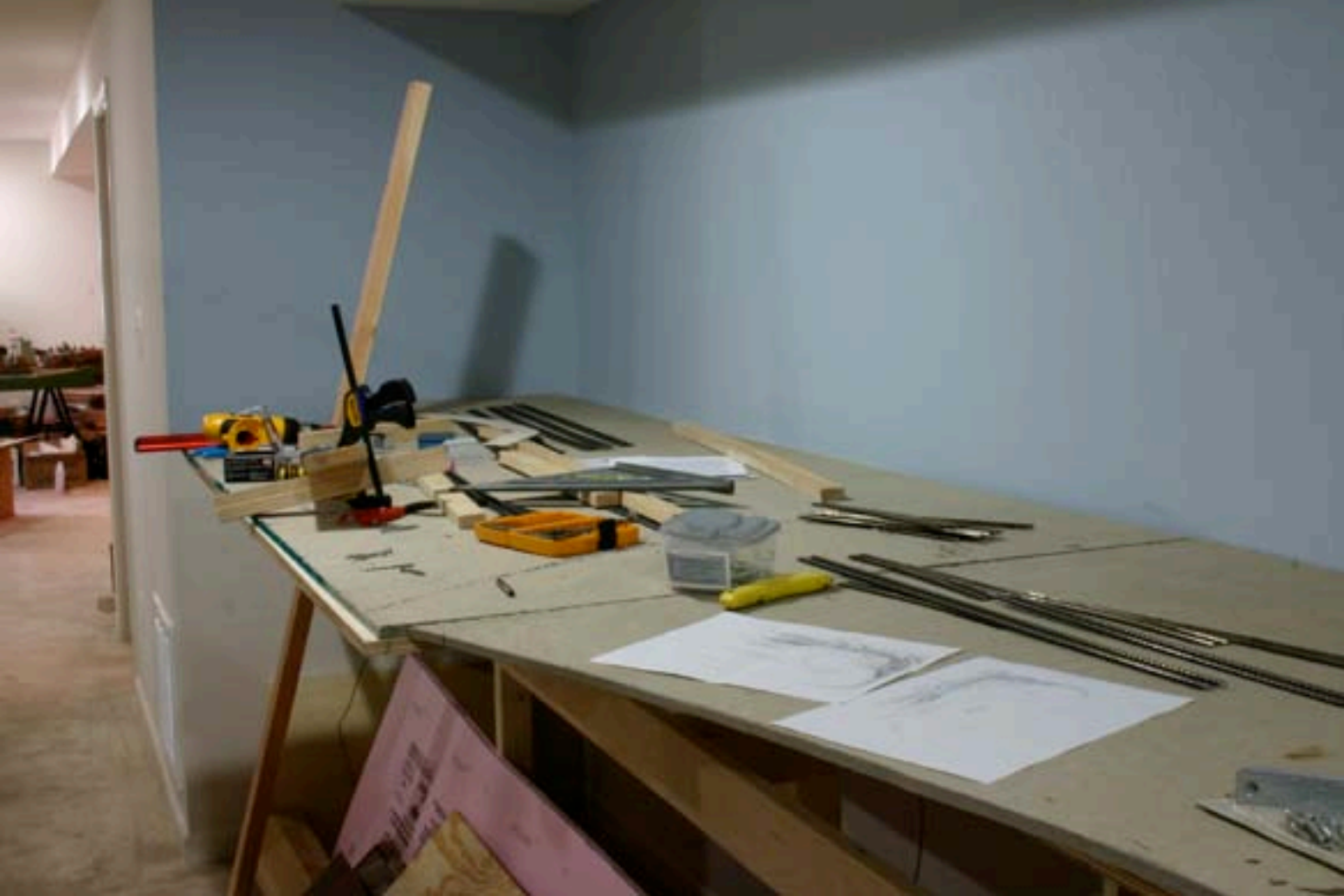
FIGURE 2: This photo shows the pier area in the early benchwork stages. The narrow aisle to the left of the short wall is visible. It was impractical to penetrate that short wall because the HVAC is on the other side.
