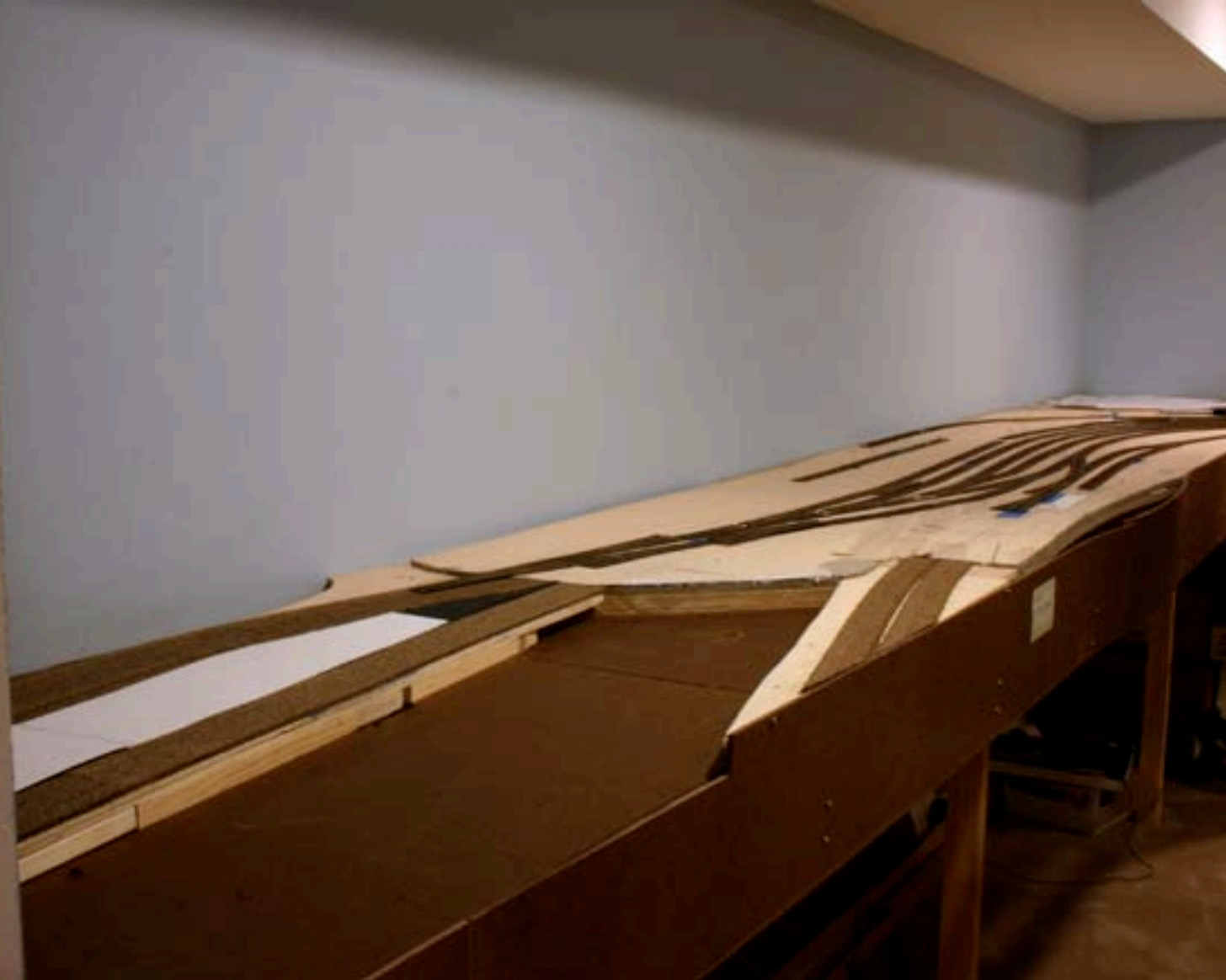
FIGURE 6a: These two views of the reworked pier area can be seen here (trackwork is still under way). The State Pier ends at the benchwork, an “aisle side” industry. The railroad pier is behind it on the left.
