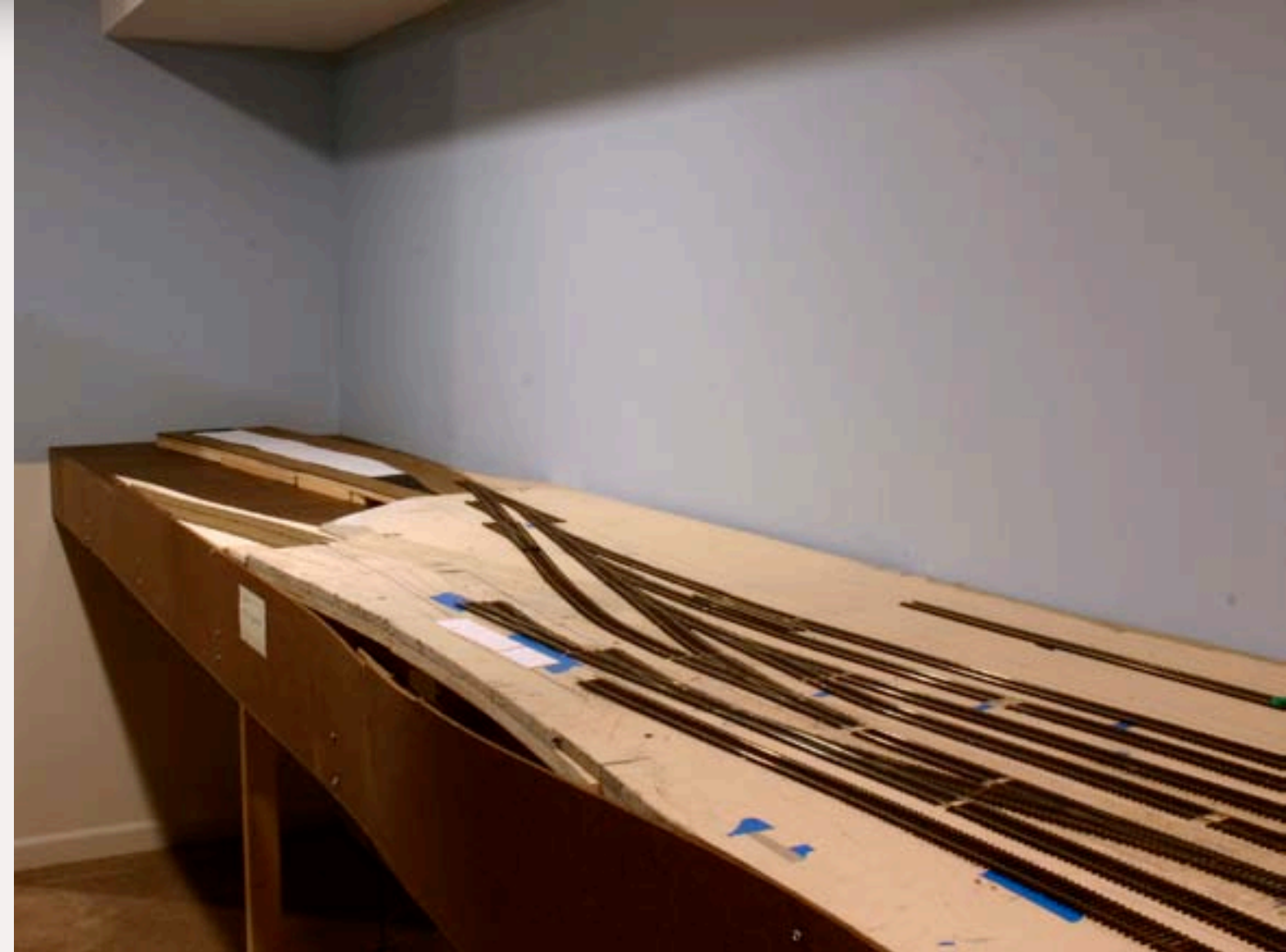
FIGURE 6b: The white posterboard footprint marks the approximate outline of the freight platform and shed. At last, all is right with the world in the Thames Street yard.
