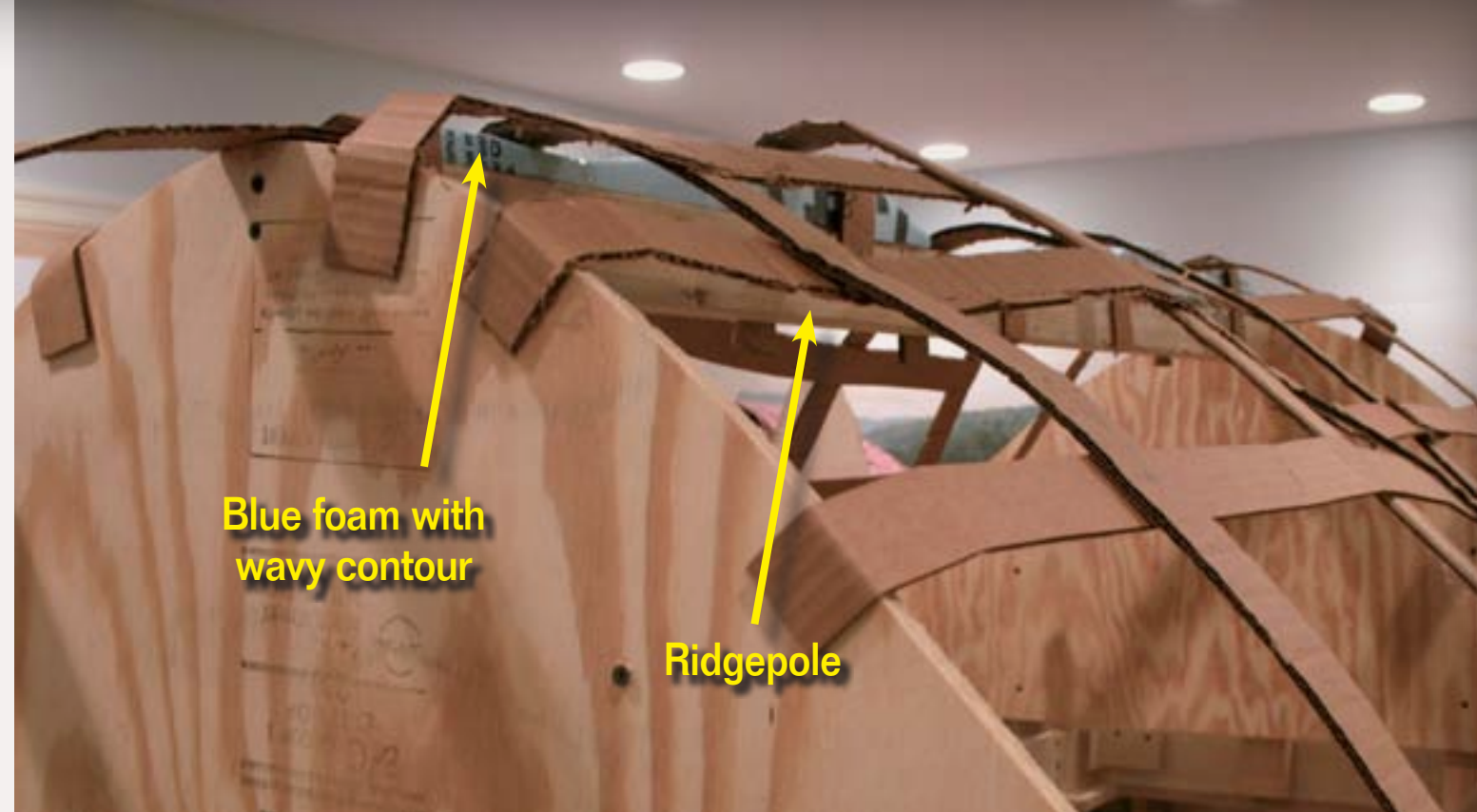
FIGURE 3: Cardboard grid glued over plywood forms shows the terrain contours taking shape. Note the blue foam on top of the ridge pole.
