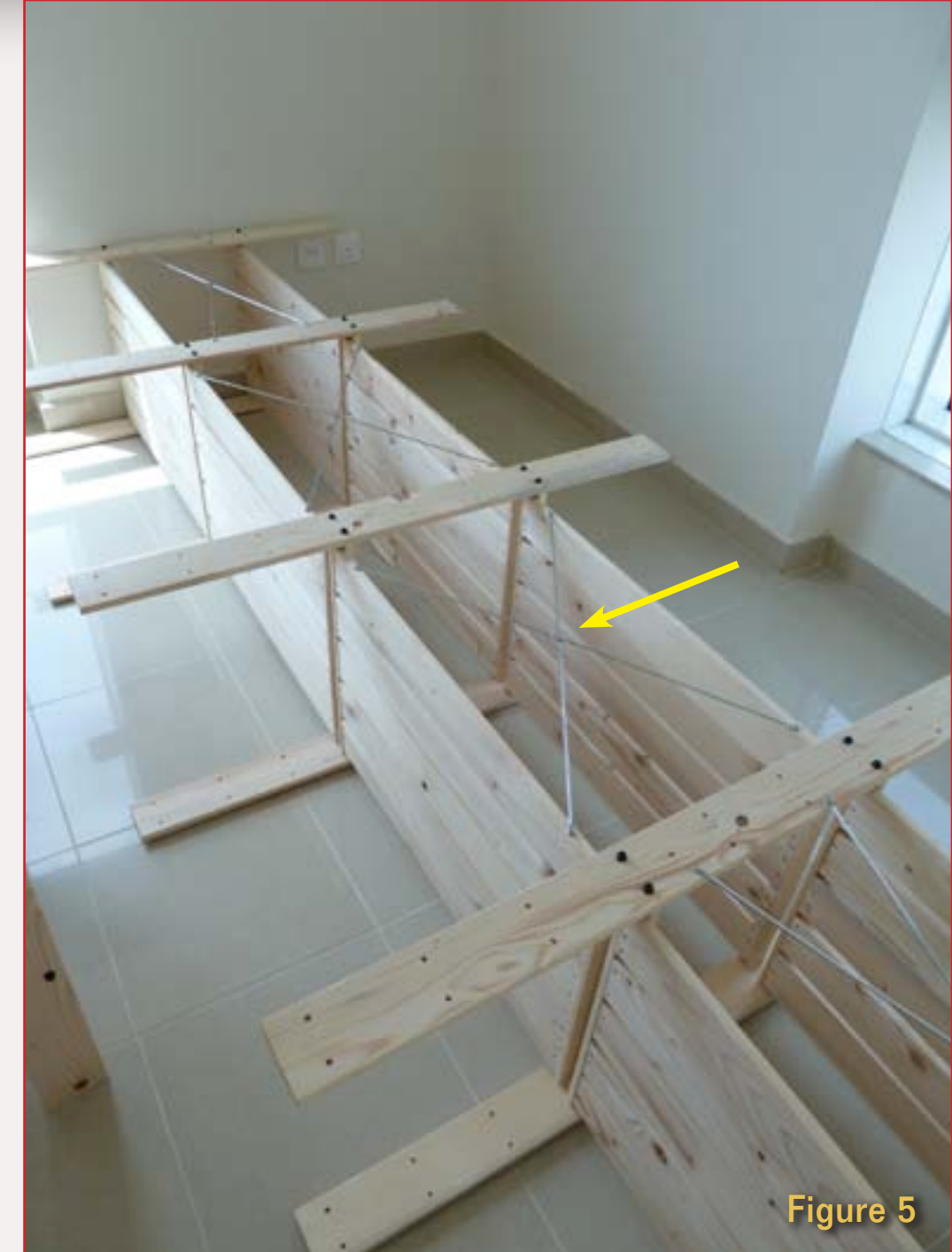
Figure 6: The metal cross braces didn't reach across every section, so I tied them into the shelves themselves. The one on the left is on the post, the one on the right, the shelf.
