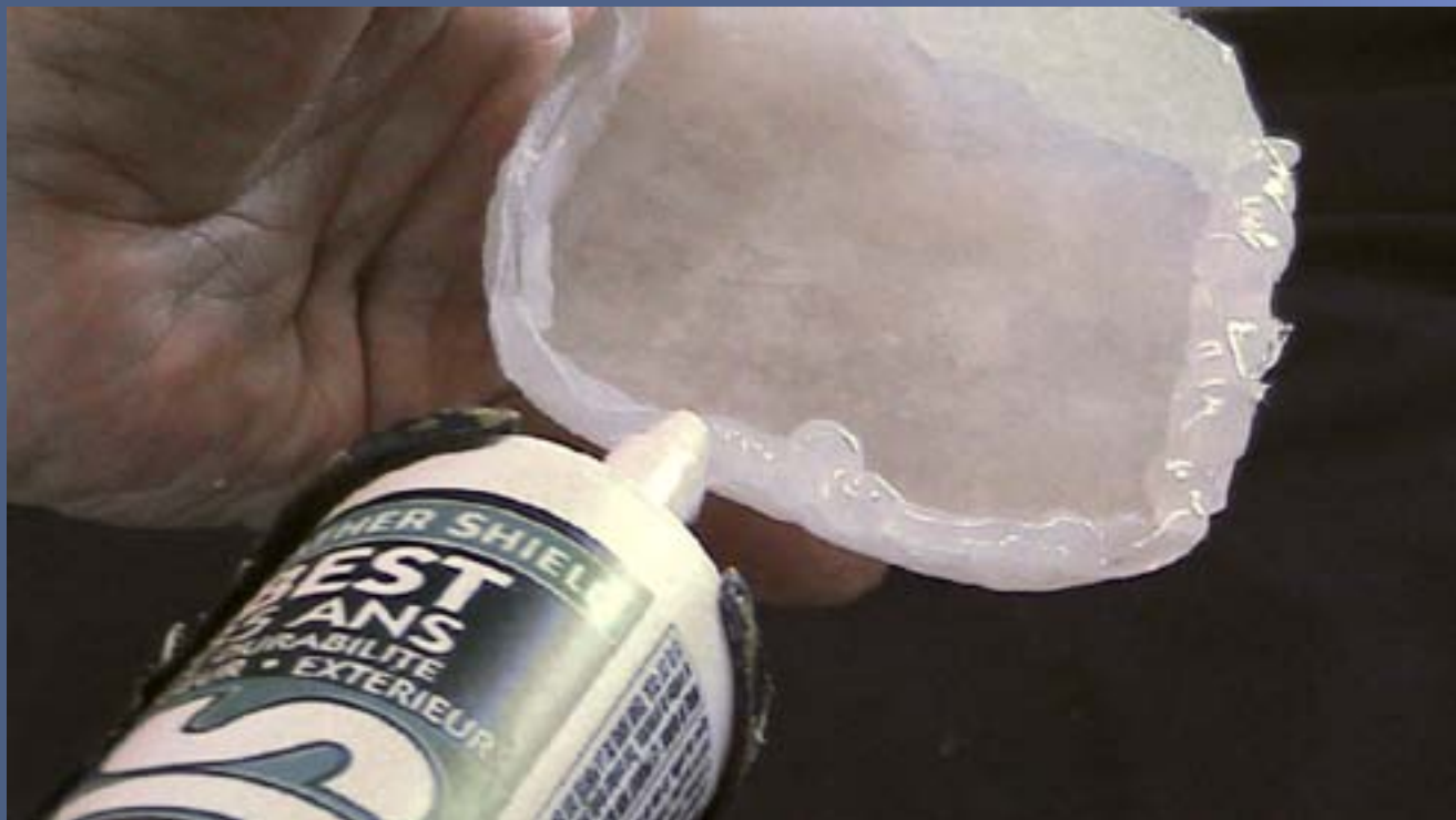
Figure 9. Applying the edge bead.
