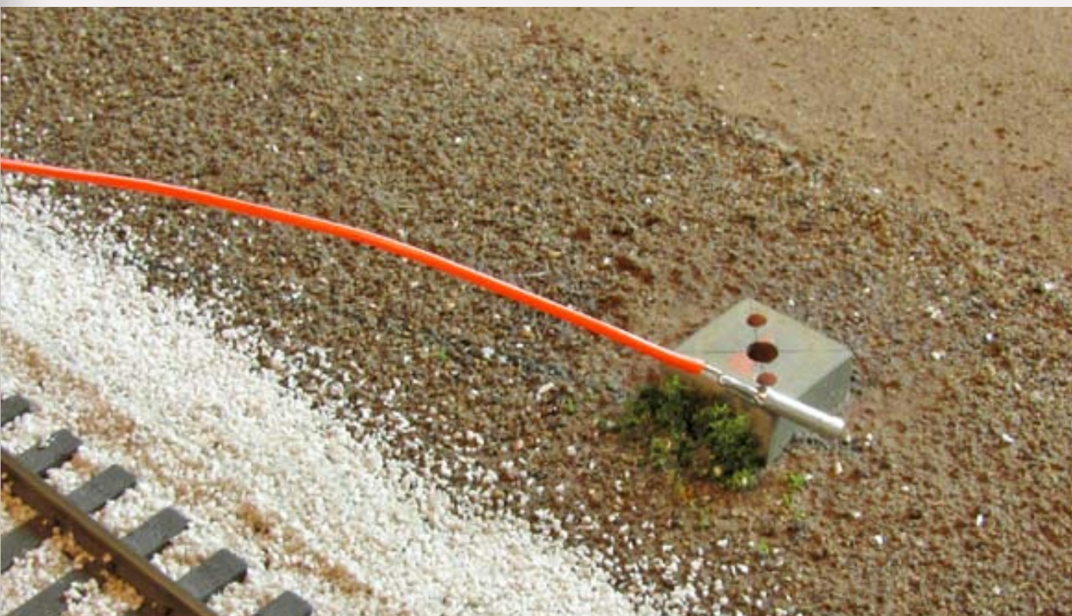
Figure 5: The header pin with a wire soldered onto it is ready to be installed.
