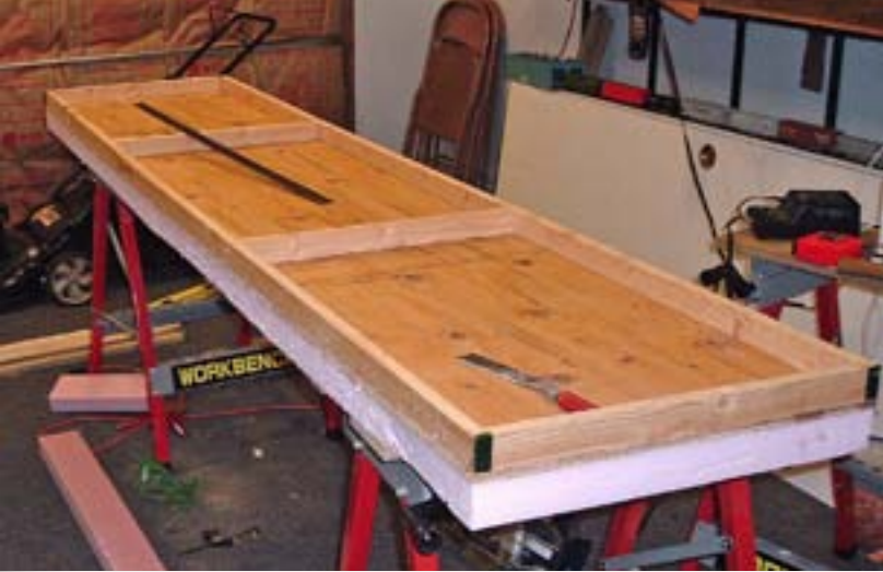
Figure 3: You can see the simplicity of domino benchwork. Here's an upside down domino (topped with 2" of pink foam). Add 2x2 legs in each corner.
