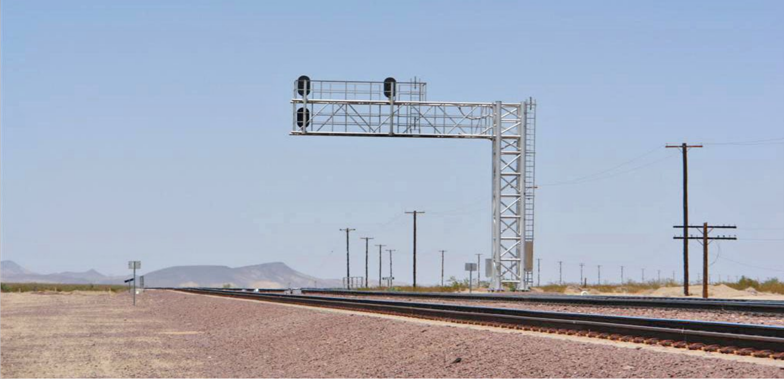
Figure 1. Eastbound train view, of the back of the cantilever signal bridge.
