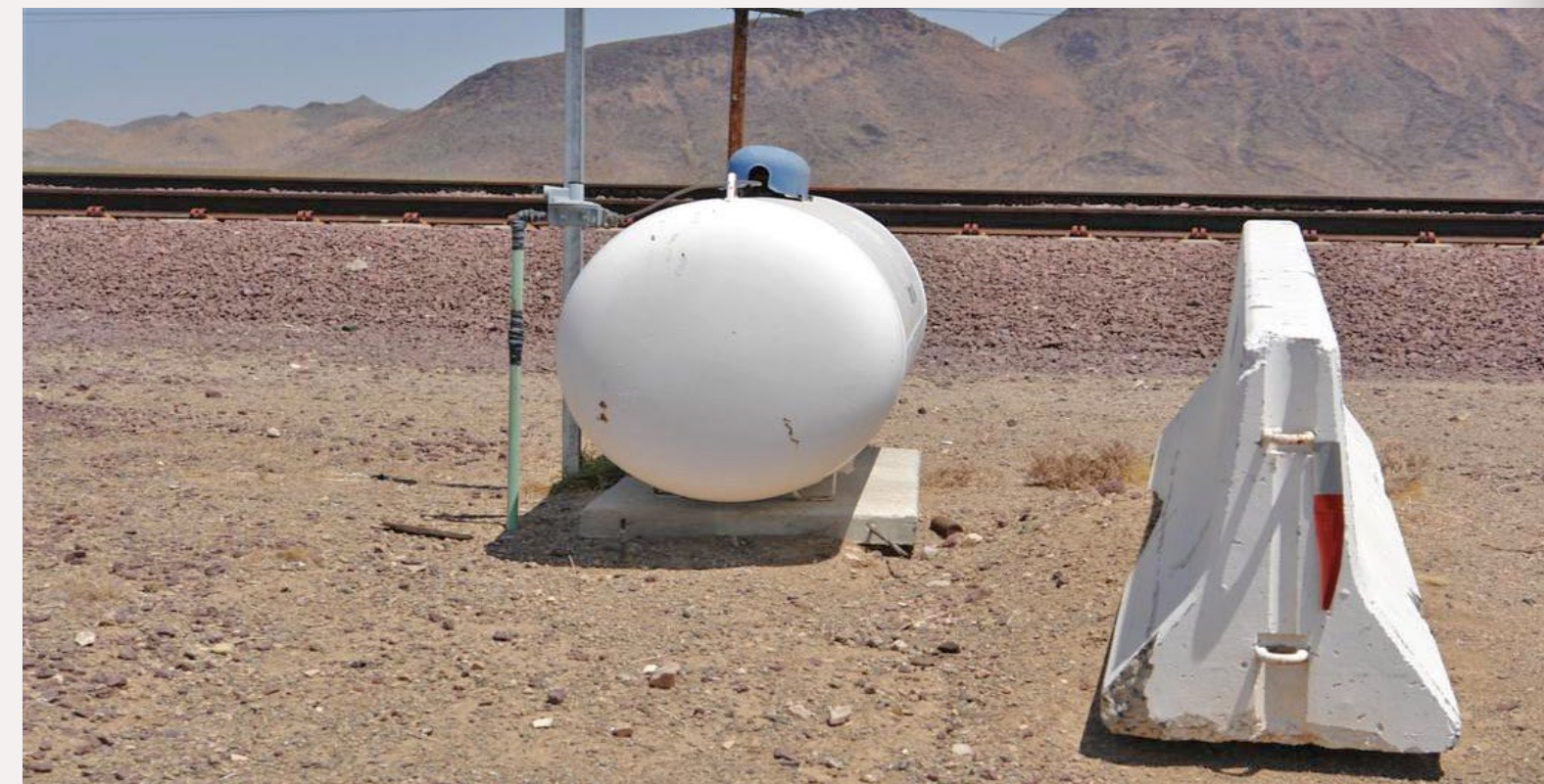
Figure 3. Propane tank and jersey barrier.
