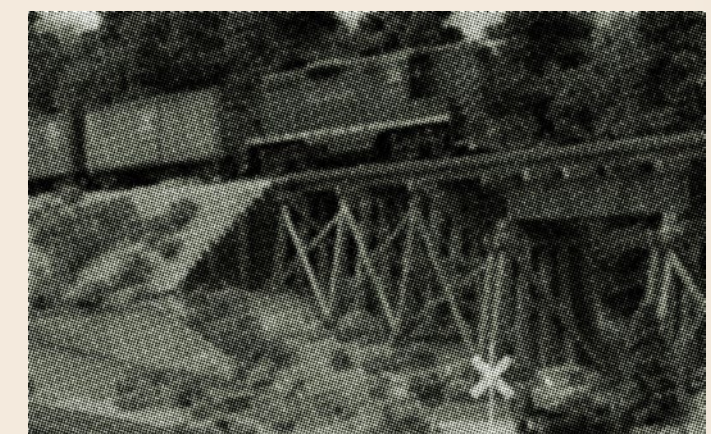
The refurbished trestle with X bracing
