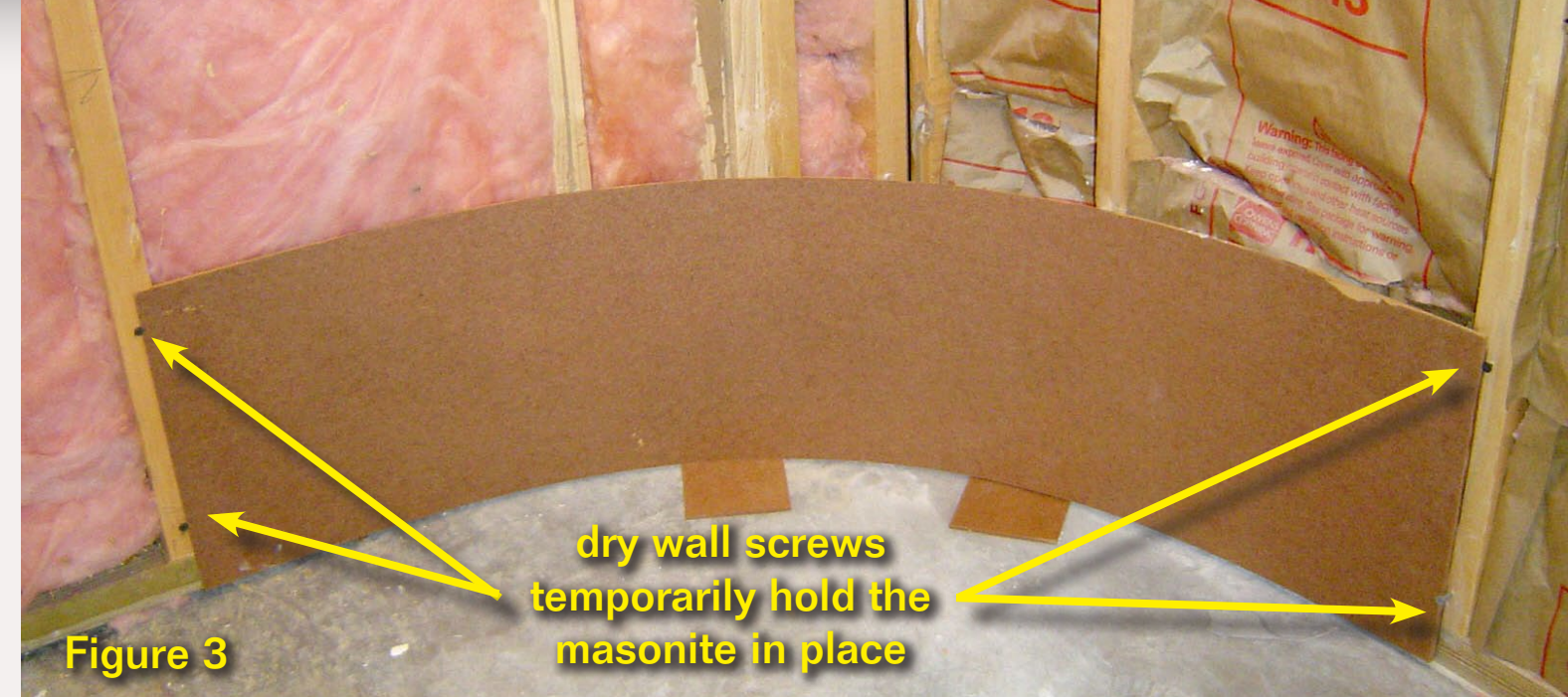
Figure 3: The first thing that I did was test-fit a piece of 2' high by 4' long by \frac{3}{16} " thick hardboard in the corner using some drywall screws screwed into the studs (not through the hardboard) to hold it in place. The stud spacing, 28\frac{1}{2} " from the corner in both directions, allowed for an attractive curve with the hardboard fitting flat against the studs. If the stud spacing wasn't acceptable, I would have added intermediate studs.
