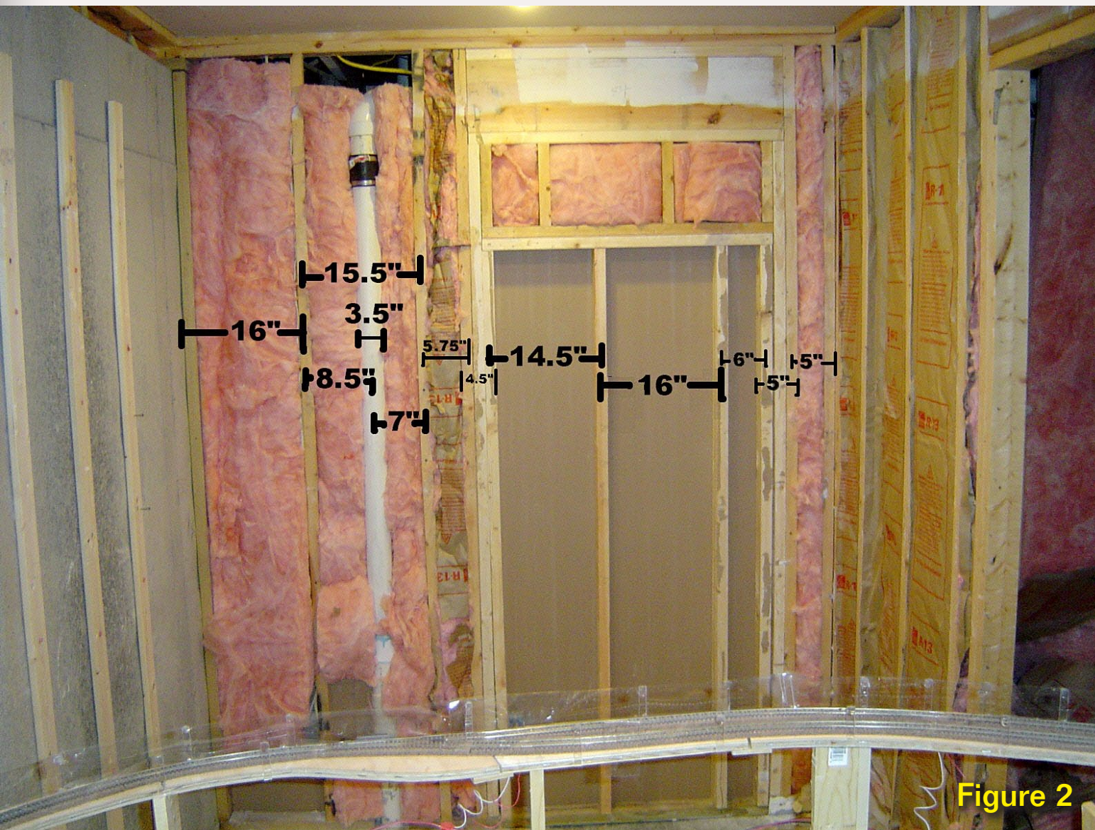
Figure 2: Here is the reclaimed 6 x 7 space looking from the existing train room. I've studded-in the old closet entrance in the back wall and will close up the entrance that already existed to the right.
