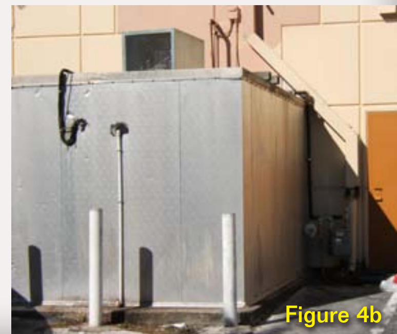
Figures 4a and 4b: A typical modern walk-in cooler added to the rear of a building.
