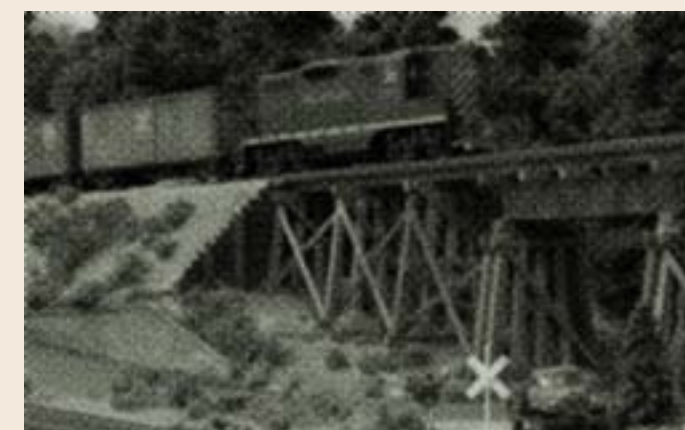
The refurbished trestle with X bracing
