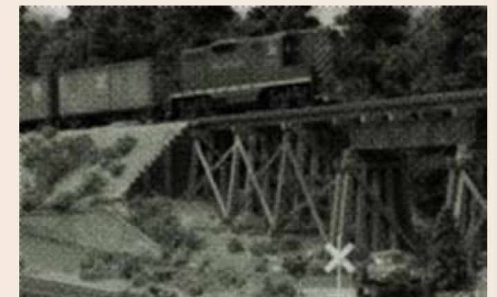
The refurbished trestle with X bracing
