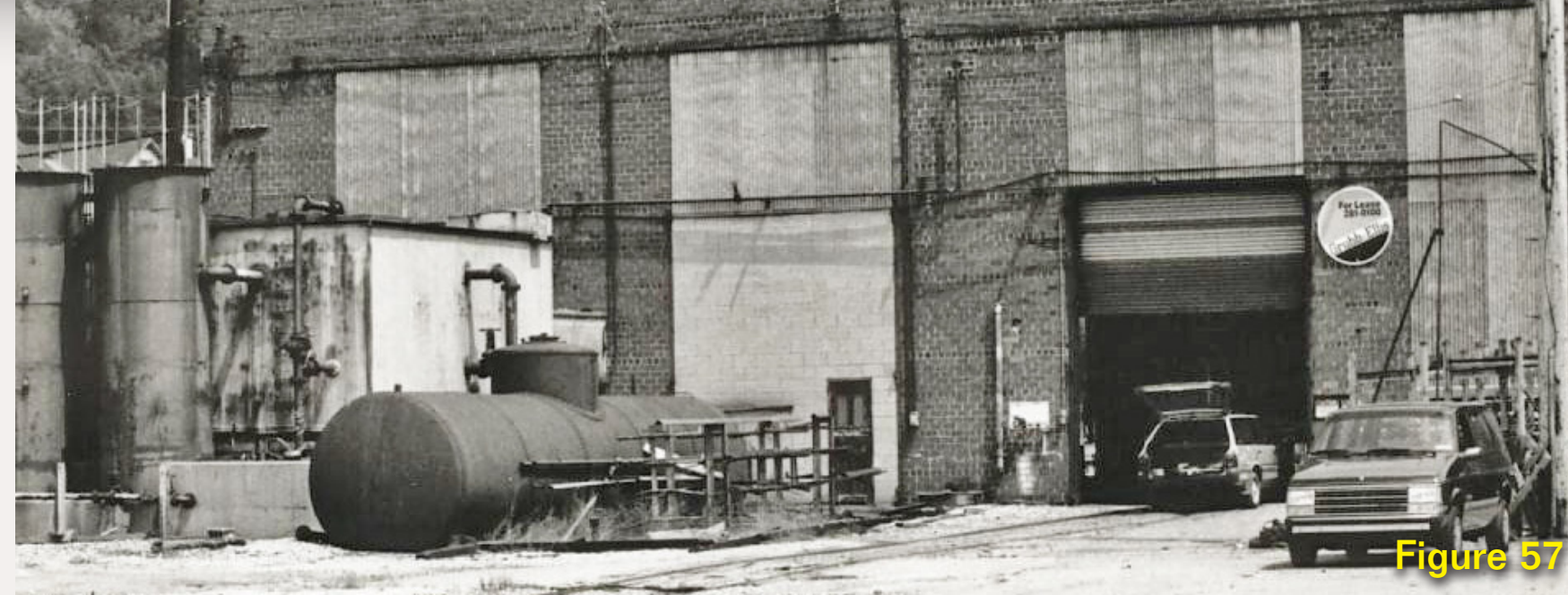
Figure 57: This is the engine house at Rook Yard circa 1992. The tank system was used to process used oil from the locomotives. This would make a great little scene on the back side of an engine house.
