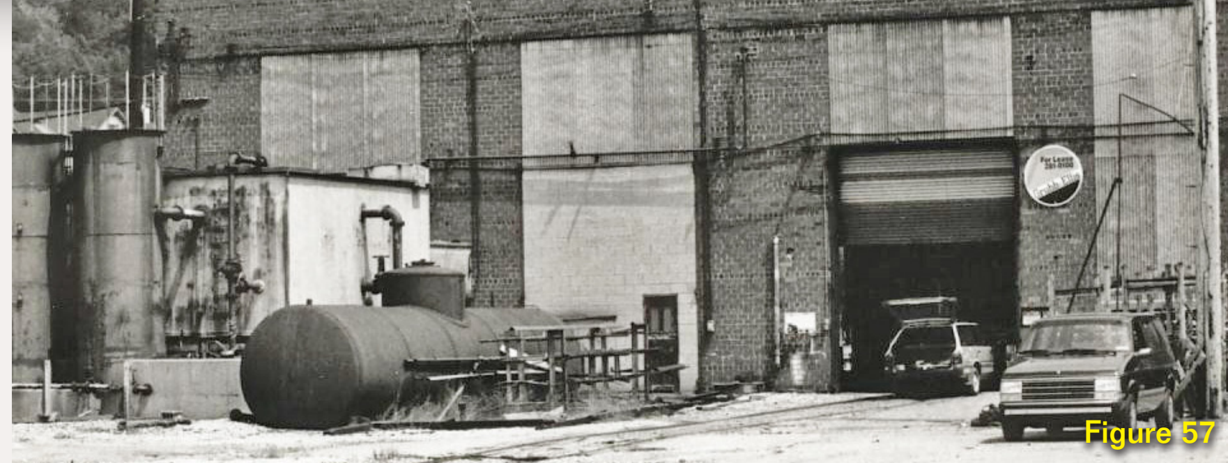
Figure 57: This is the engine house at Rook Yard circa 1992. The tank system was used to process used oil from the locomotives. This would make a great little scene on the back side of an engine house.
