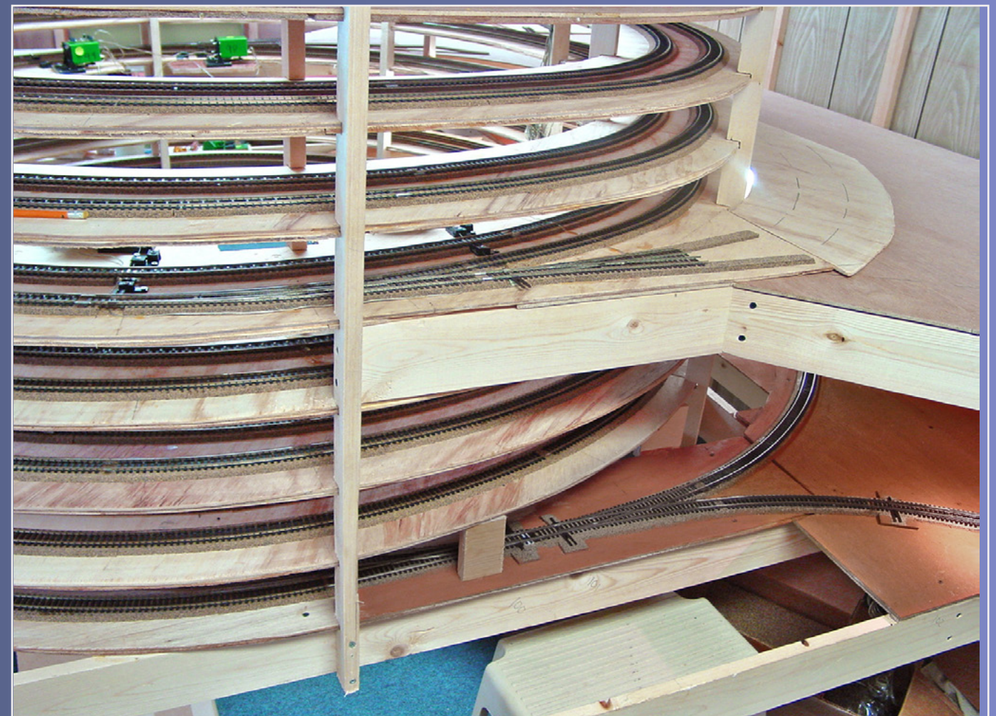
Figure 15: Tier level 4 exit to the middle deck benchwork, with the beginnings of the middle deck taking shape.
