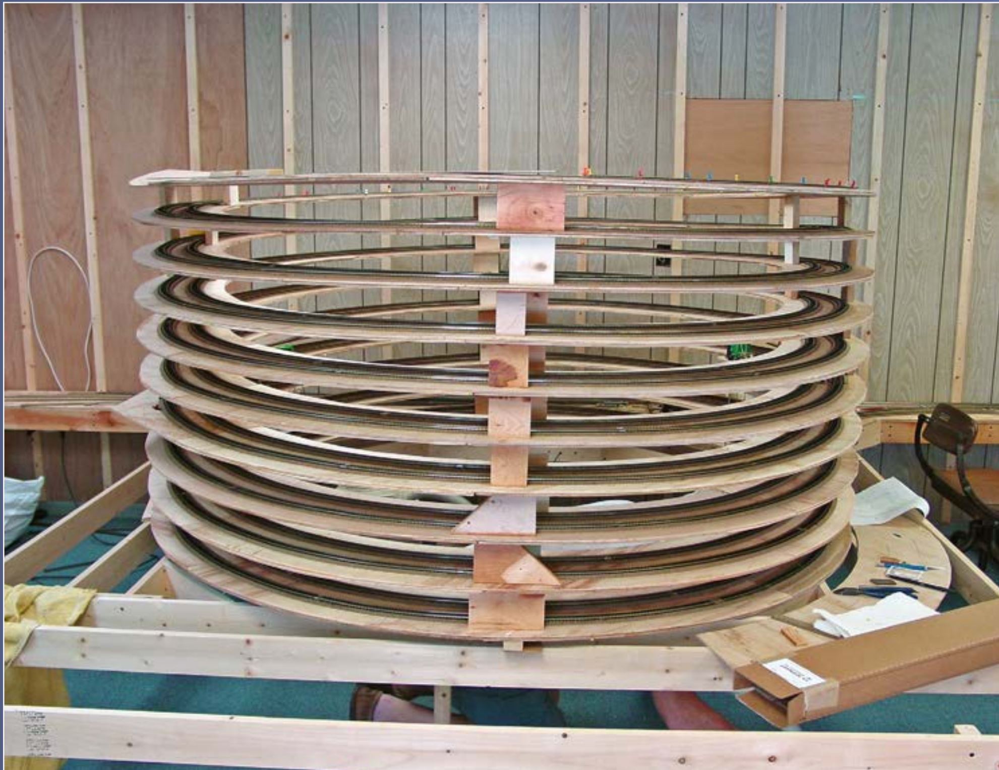
Figure 12: With all the track laid, the helix tiers were temporarily raised into place using scrap 1x4s.
