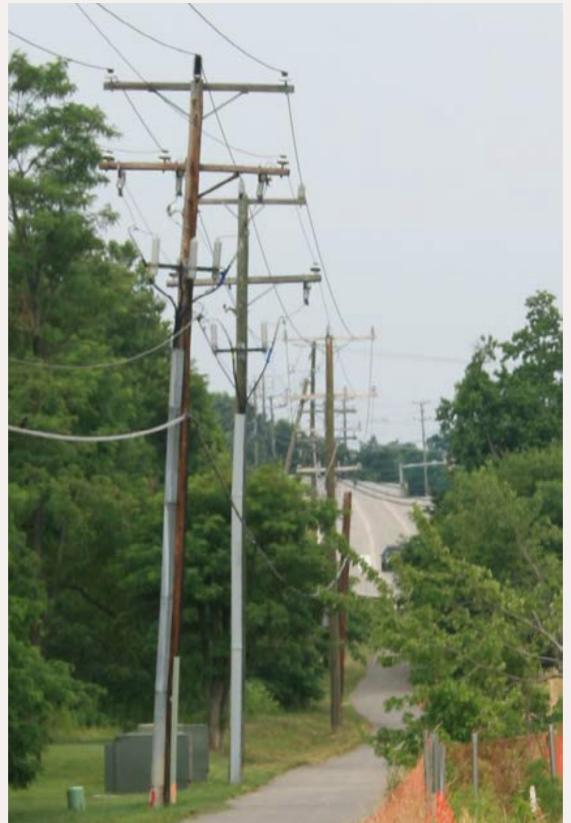
Figure 1: This line of poles shows the variety inherent even in modern utility poles.
