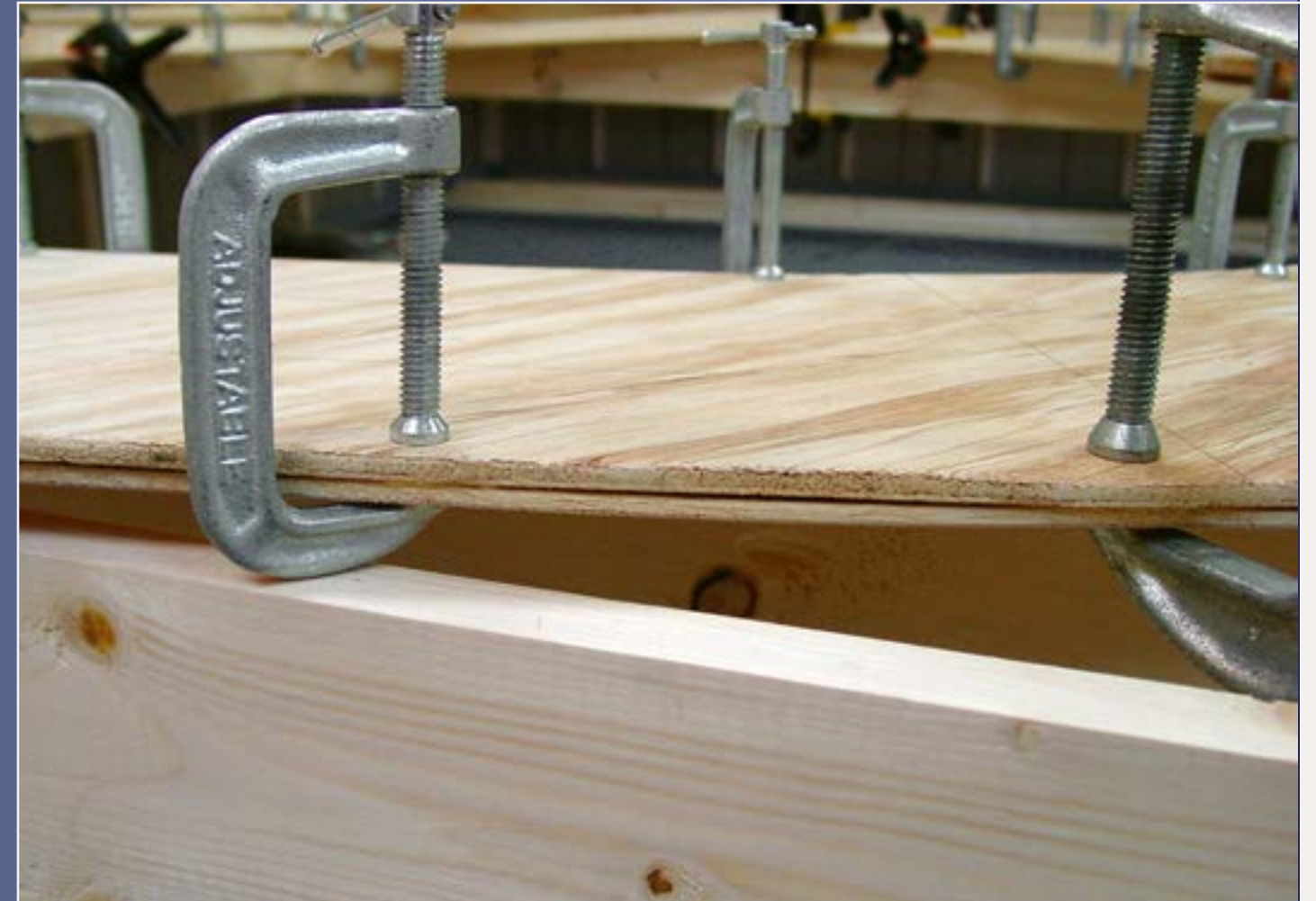
Figure 7a: We laminate two 1/4" layers of lauan plywood sub-roadbed together using carpenter's glue and clamps to get one 1/2" plywood sandwich. By staggering the joints in the layers, no joint splice plates are necessary.
