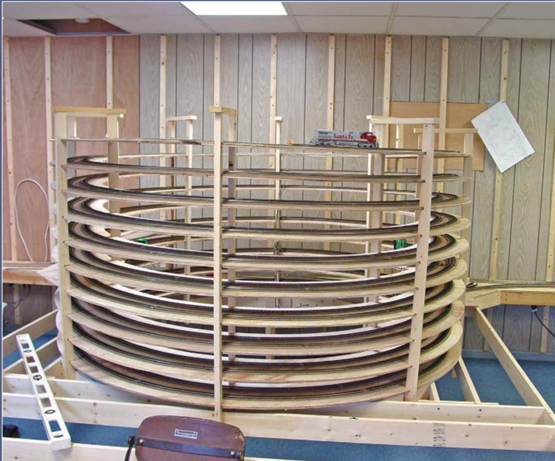
Figure 13: Helix, with all the 1x2 risers added.
