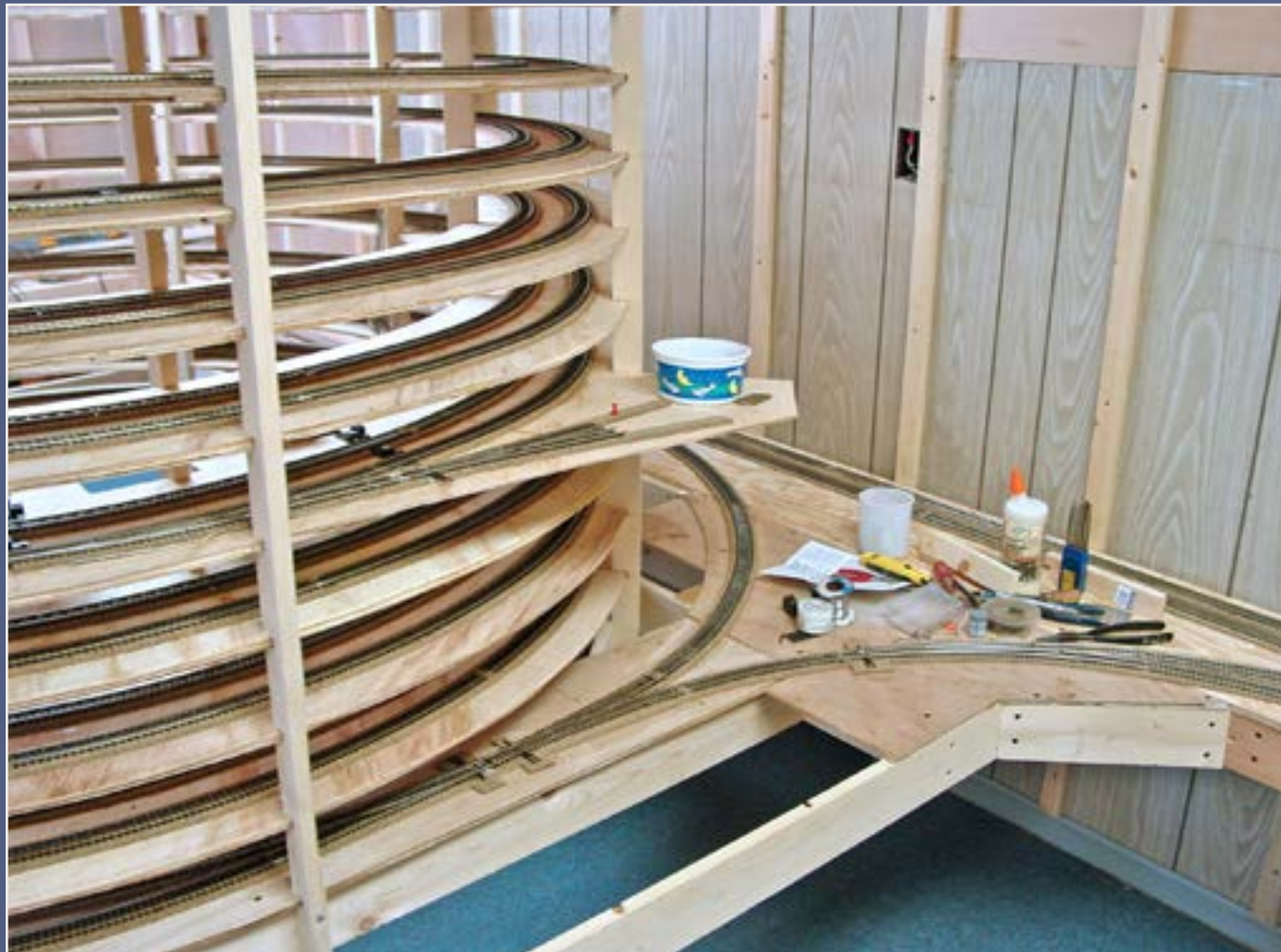
Figure 14: Entrance to the bottom of the helix, via a wye. Note the outside track helix exit turnout at tier level 4.
