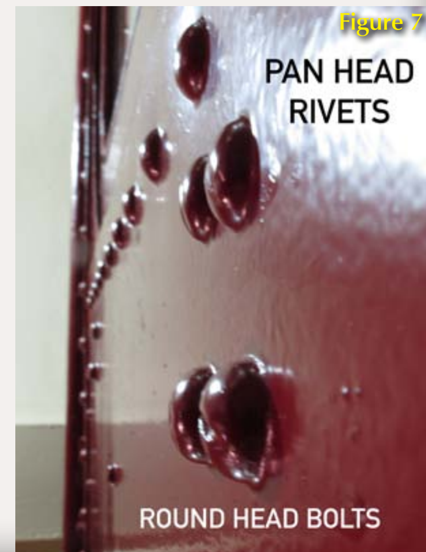
Figure 7: Bolt and rivet heads look similar but cast different size shadows.
