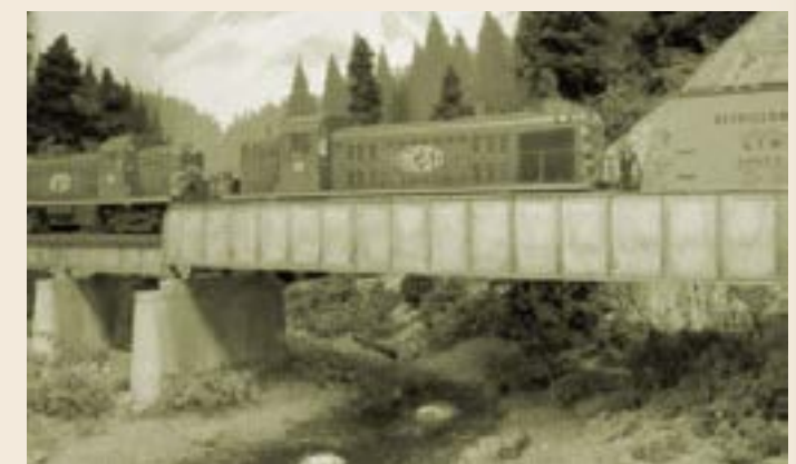
The railroad bridge across the newly wet upper Bear Creek.
