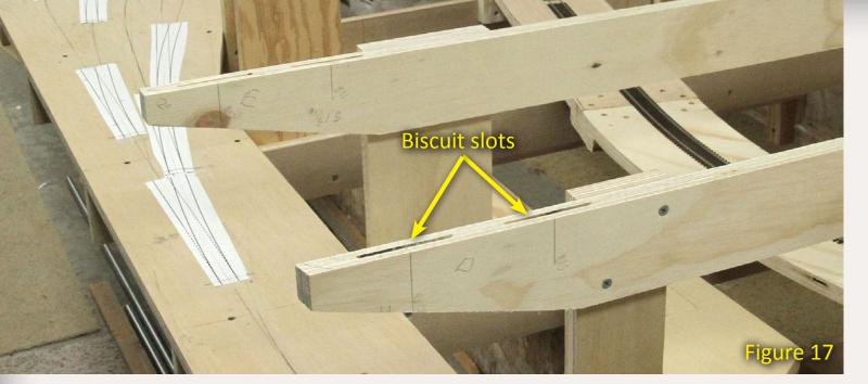
Figure 17: Biscuit slots pre-cut in the tops of joists for future installation of joist extensions to raise the height of the mainline roadbed. I discuss the use of wood working biscuits thoroughly in <u>February's Up the Creek</u>.
