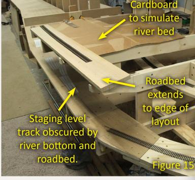
Figure 14: I clamped more joists in place temporarily to demonstrate the visibility issue. The first few joists have tapered ends improving visibility (the temporary joists beyond them are not tapered).
