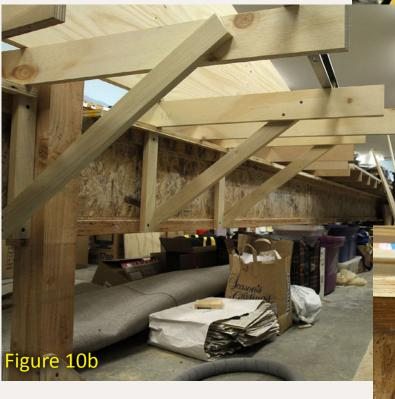
Figures 10b and 10c: The permanent joists are 3"x 3/4" plywood, and their braces are 1"x 2" poplar. Note the vertical cleats to which the braces attach at the bottom.
