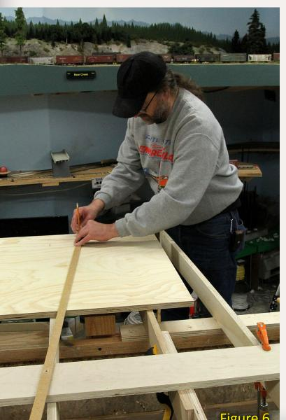
Figure 5: A trammel is the answer for plotting good arcs. But the center point was in an aisle. Not a problem – we rigged up a bit of temporary benchwork, drilled a hole at the center of the arc and stuck a nail through the trammel and into the hole.
