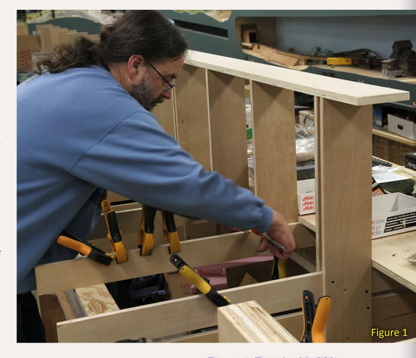
The process we used to achieve the needed riser alignment was fairly simple. I used a laser to line up a few key risers. Then used the edge of a 5" x 8' piece of 3/4" plywood to set the height of the intervening risers and keep them from leaning.
