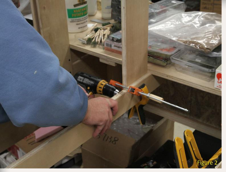
To start, we clamped a riser in approximate position. Then, using a small hammer, we micro-adjusted its height until it just kissed to bottom of the 5" x 8' plywood strip placed vertically on edge. Then we laid the plywood strip flat across the tops of the neighboring risers, tapping the new one to make it plumb with its neighbors.
