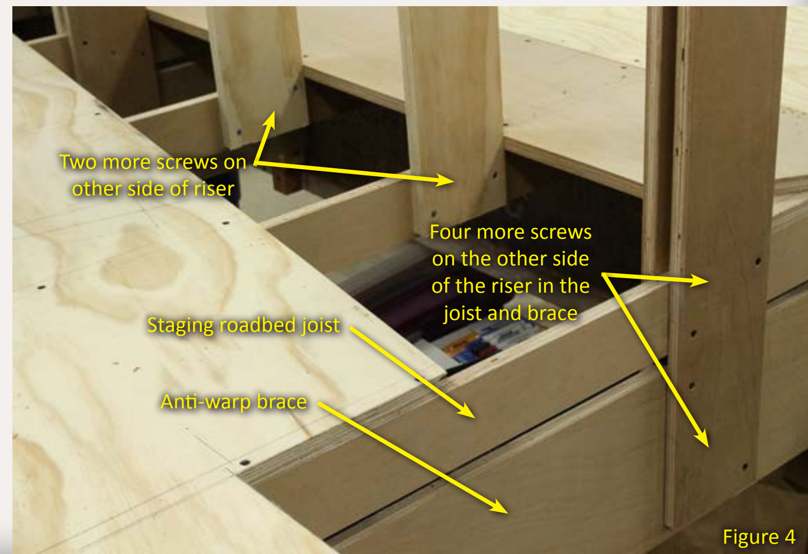
Figure 4: I put four screws in each "single" riser and eight screws in each double riser. The screws are driven half from one side, half from the other.
