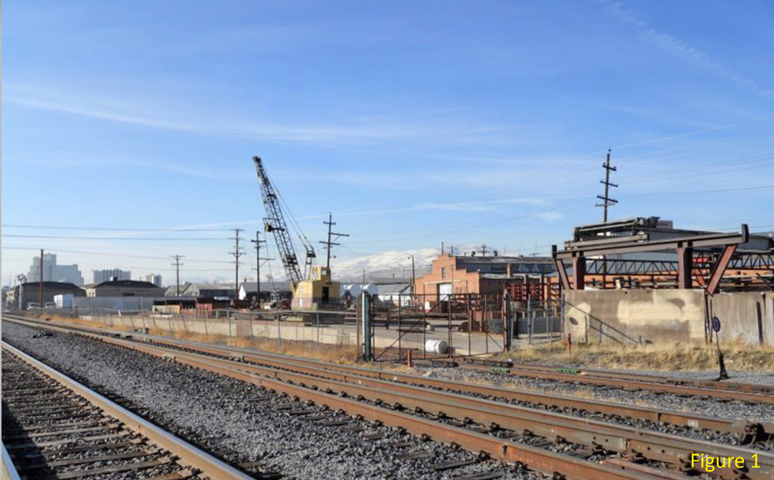
Figure 1: Reno Salvage located on the east side of Sutro Street.
