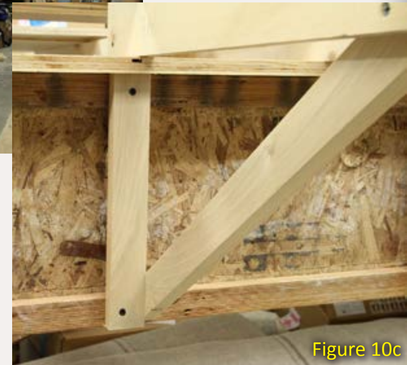
Figures 10b and 10c: The permanent joists are 3"x3/4" plywood, and their braces are 1"x2" poplar. Note the vertical cleats to which the braces attach at the bottom.
