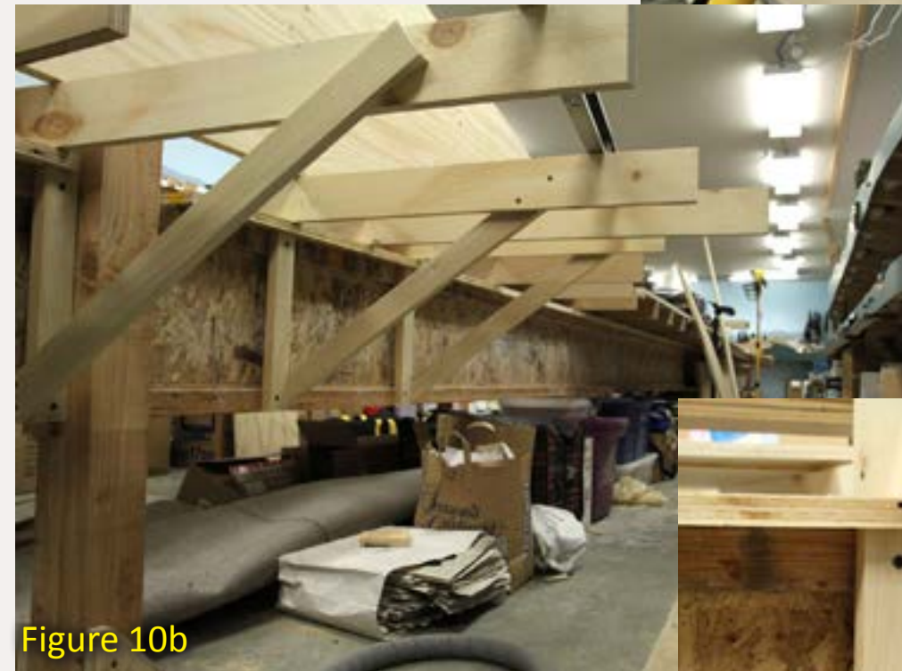
Figures 10b and 10c: The permanent joists are 3"x3/4" plywood, and their braces are 1"x2" poplar. Note the vertical cleats to which the braces attach at the bottom.
