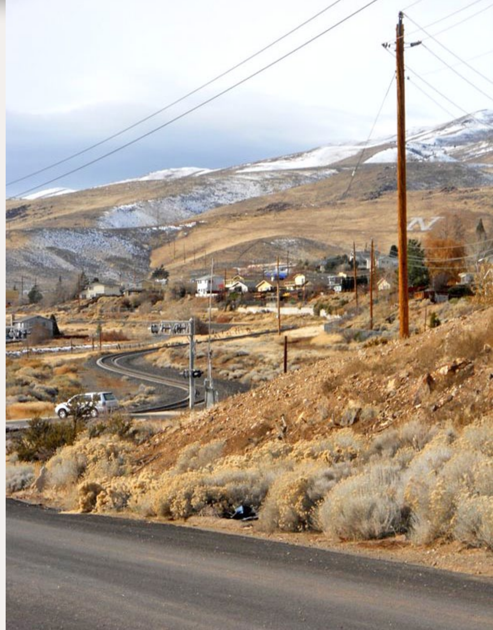
Figure 35: A good view of the serpentine nature of the line from a service road just north of McCarran Avenue. The vehicle is on Socrates Drive. This view is from the same vantage point as that in photo 34.
