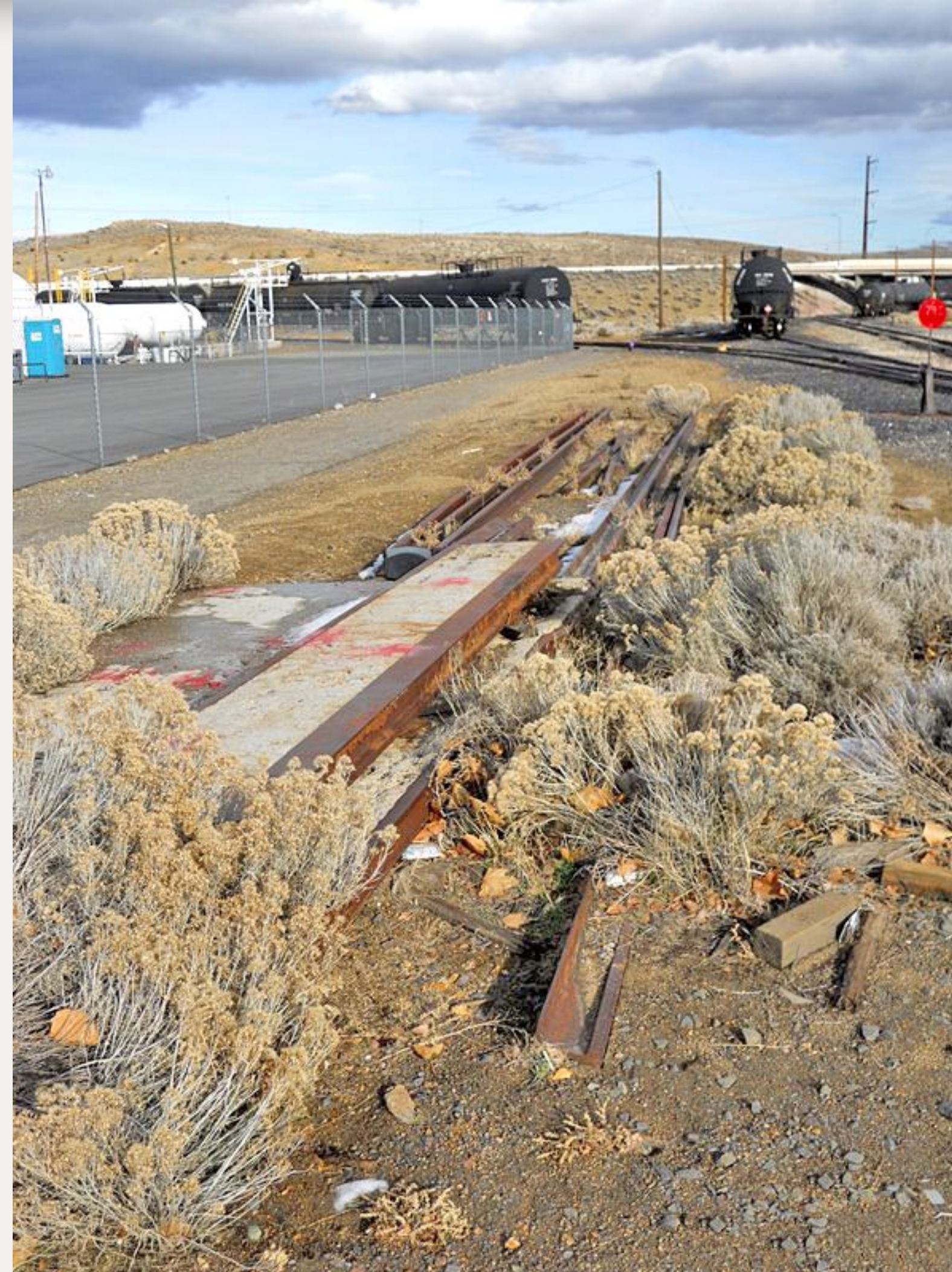
Figure 56: Remnants of the old crossing at North Virginia Street.
