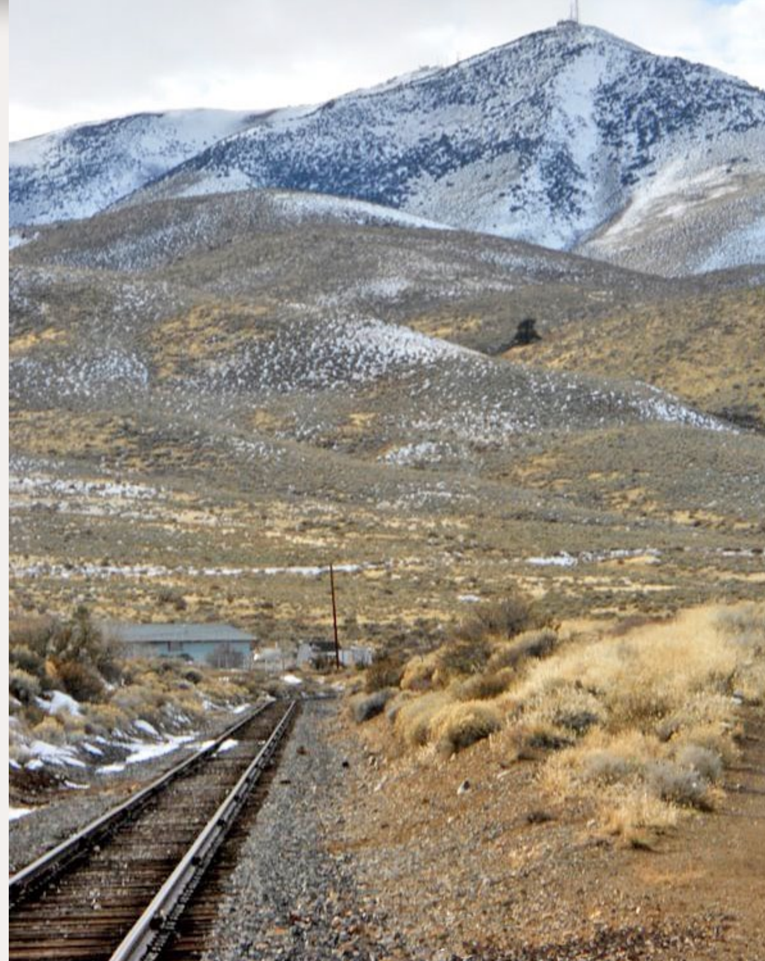
Figure 58: The line continues north to the Stead branch. At the junction there are sidings for both the line to Portola and the branch line down into Lemon Valley.
