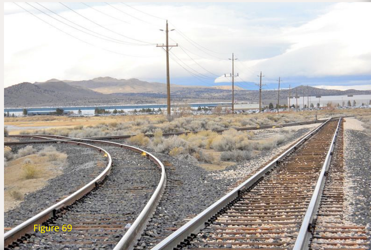
Figure 69: Some interesting track work located just east of Lear Blvd. The track in the left foreground leads to HV Manufacturing, crossing the far track, which is one leg of a “Y” that services Performance Pipe. HV Manufacturing receives tank cars. Performance Pipe receives tank cars and covered hopper cars for the manufacture of plastic pipe. The line continues on to service two large warehouses. The first is the blue and white structure seen in the background.
