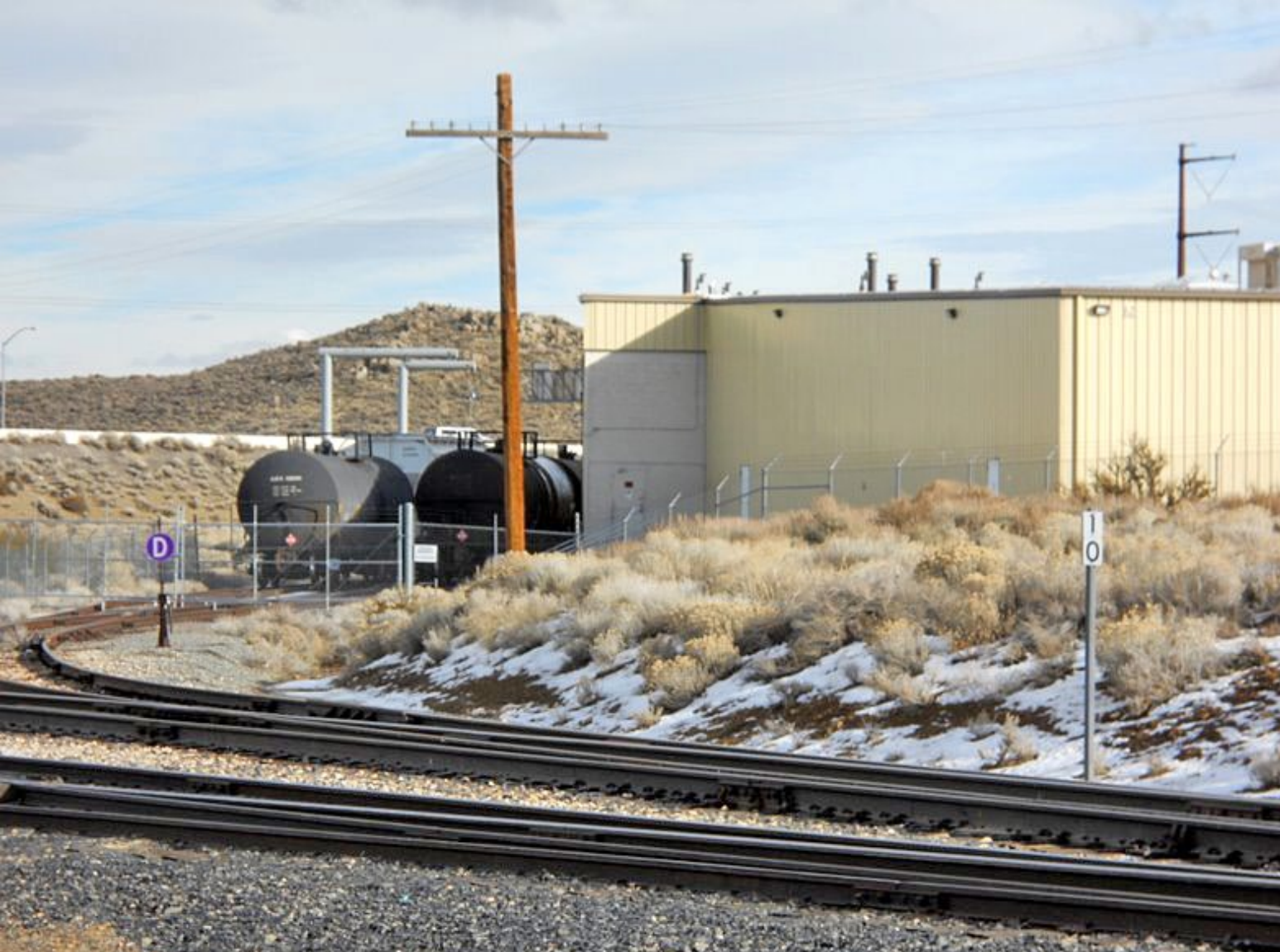
Figure 55: Cars spotted at the Sun Chemical Co. The steel supports over the car are for fall protection. A wire is strung between the supports, and workers must wear a harness that is tied off to the wire.
