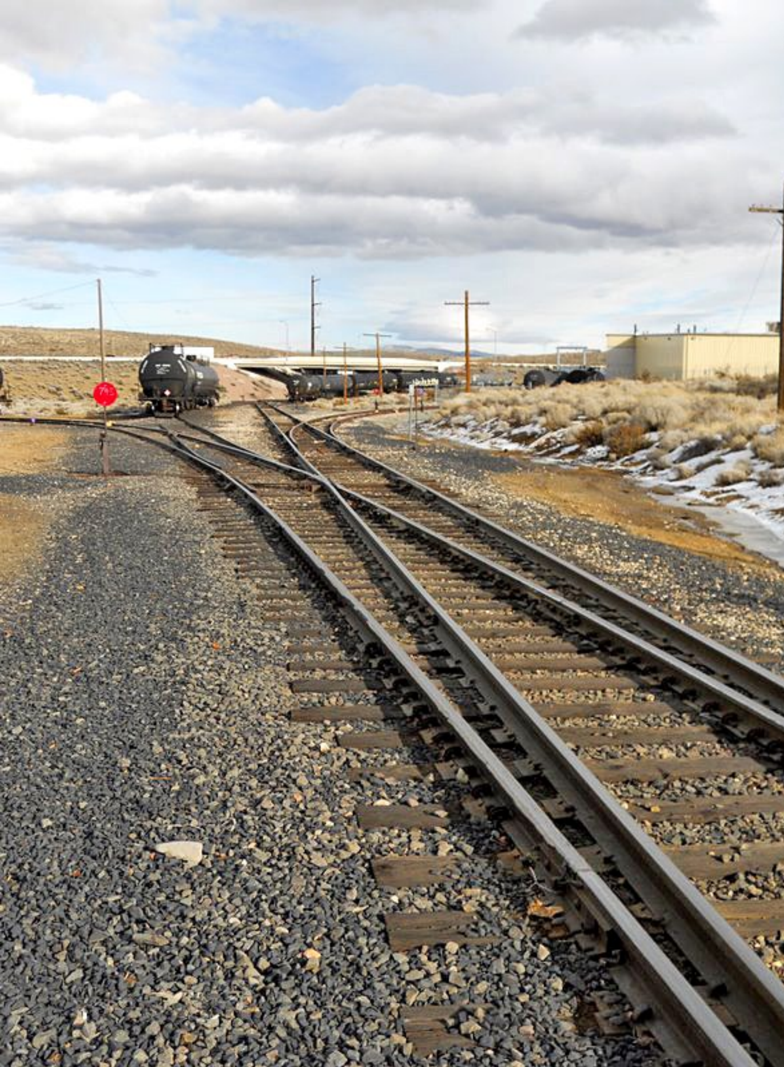
Figure 57: Looking back at the 395 overpass from Virginia.
