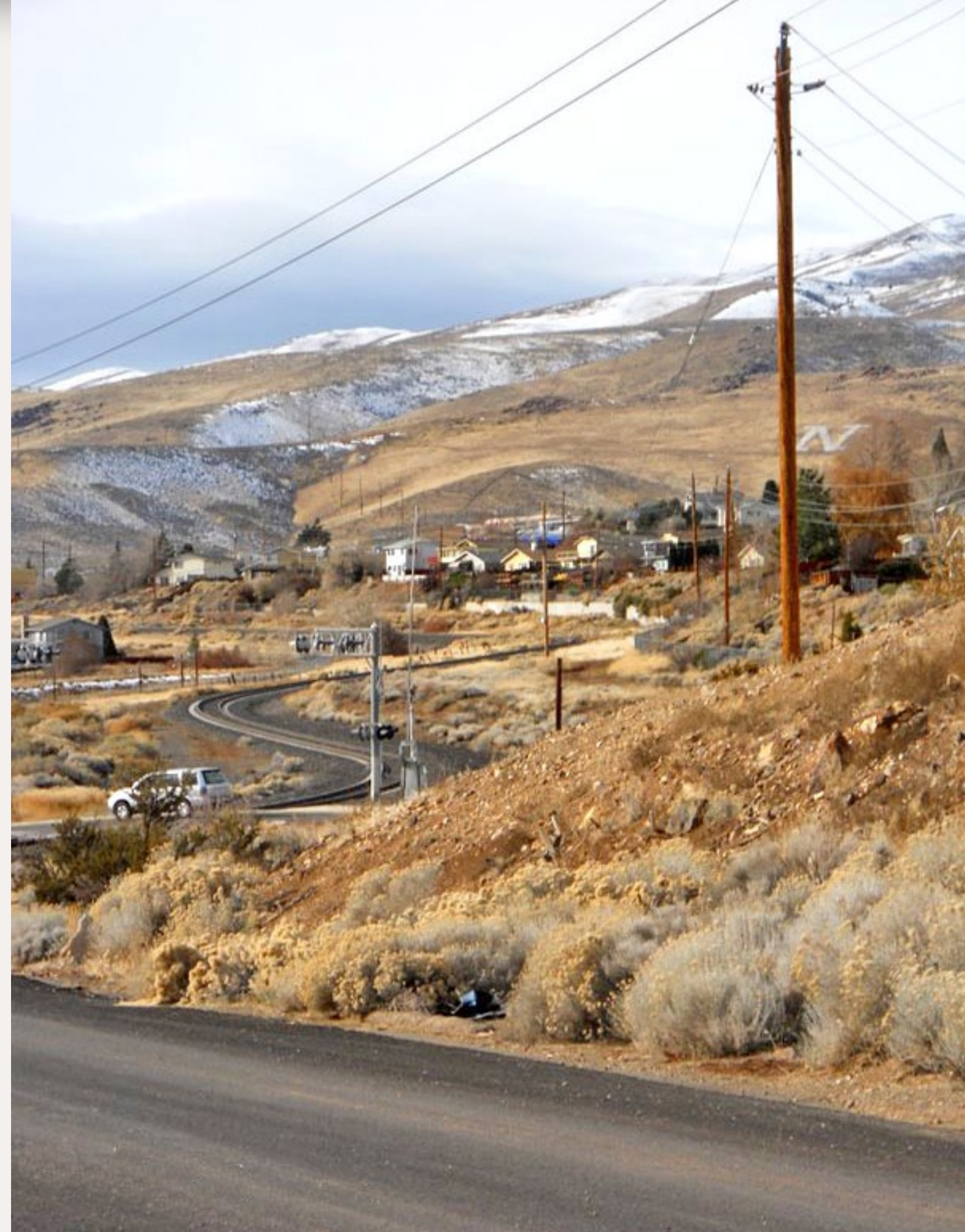
Figure 35: A good view of the serpentine nature of the line from a service road just north of McCarran Avenue. The vehicle is on Socrates Drive. This view is from the same vantage point as that in photo 34.
