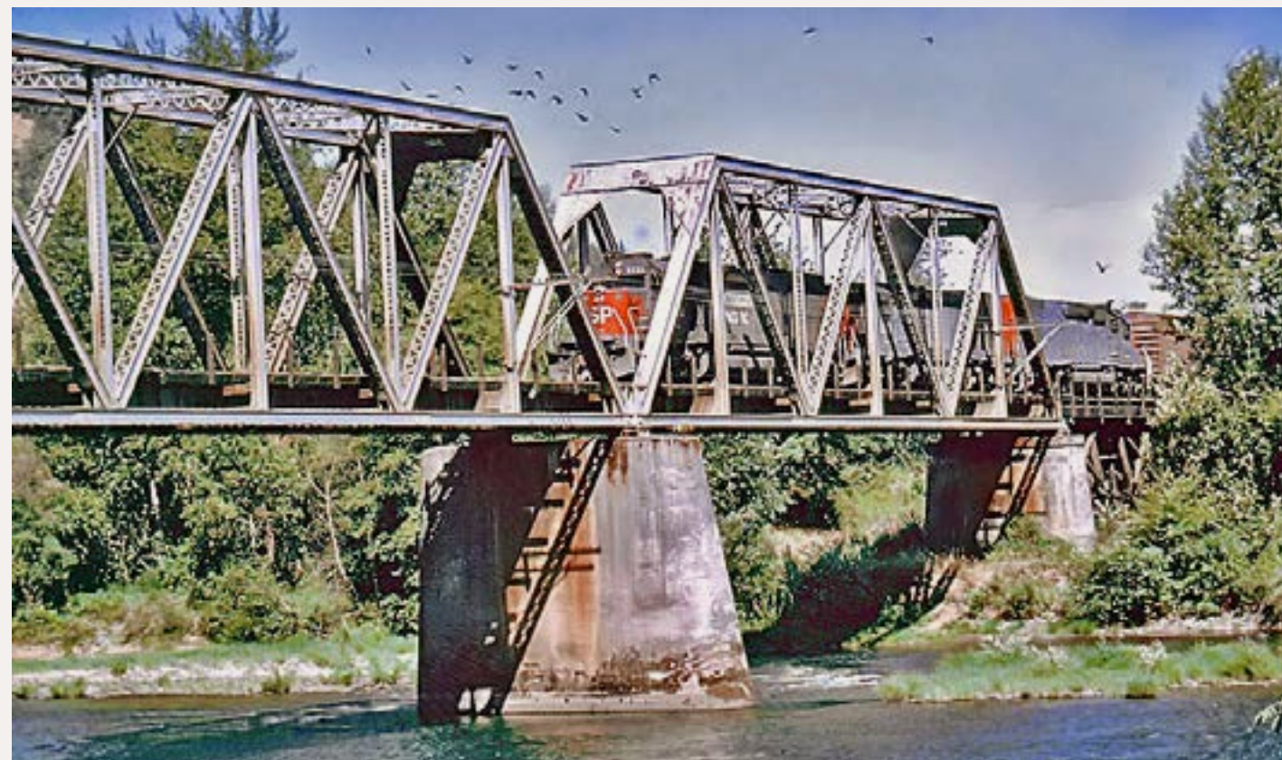
Figure 4: To carry code lines across a stream, the Southern Pacific attached crossarms to the sides of this bridge over the Umpqua River in southern Oregon. Joe Fugate photo.
