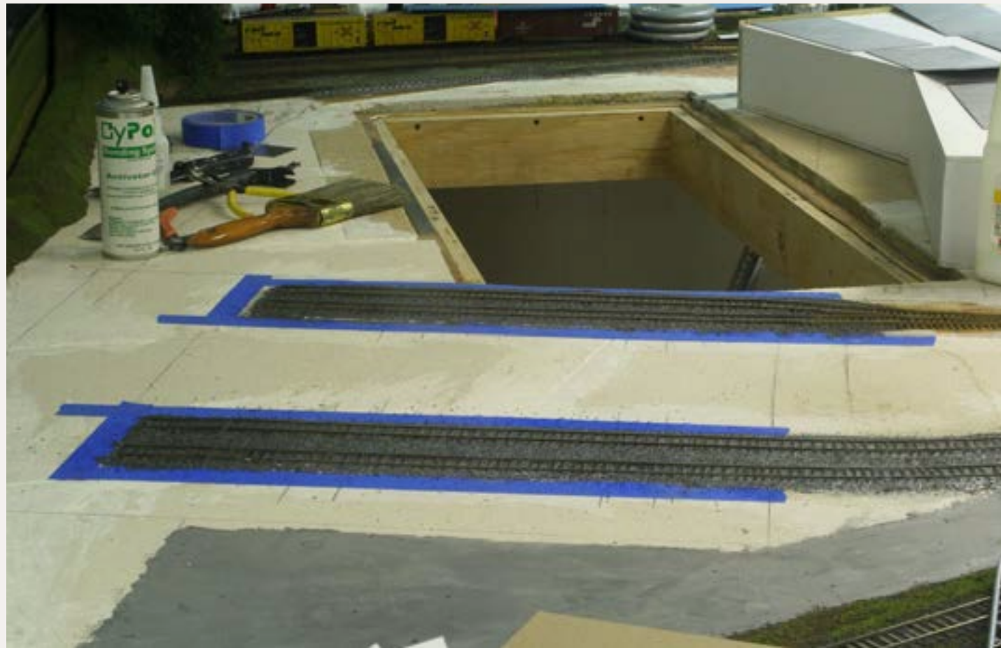
Figure 3A: Prior to installation of the building itself, it was necessary to ballast the tracks. I used blue painters tape to keep the ballast only to the areas inside the cement block walls and not under the building itself. Note also that the track on the first pair of sidings has been extended.
