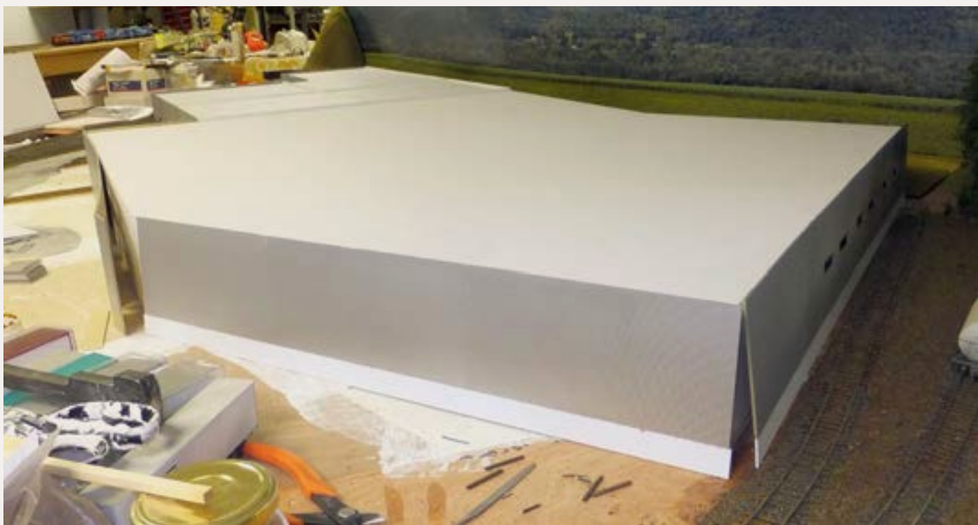
Figure 1X: The manufacturing building is in the process of having its siding bonded to the building core, in this case constructed from Gatorfoam Foam Board.
