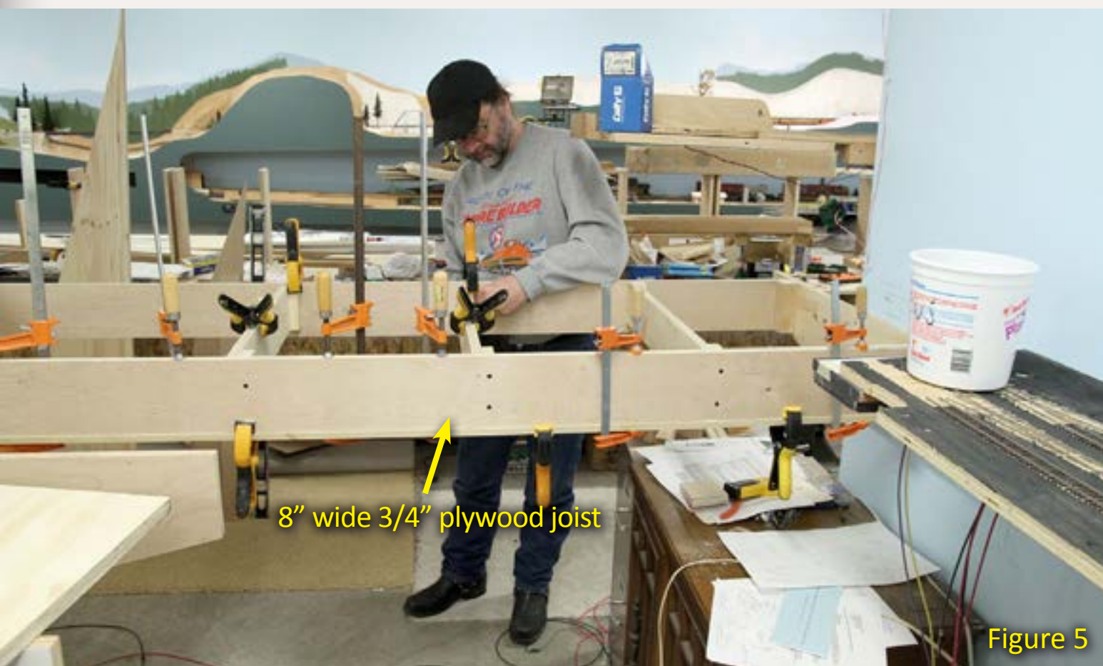
Figure 5: Two joists with cross members span the gap between the peninsula's helix table and the around-the-walls portion of the layout. Mike is gluing, clamping, and screwing it all together.
