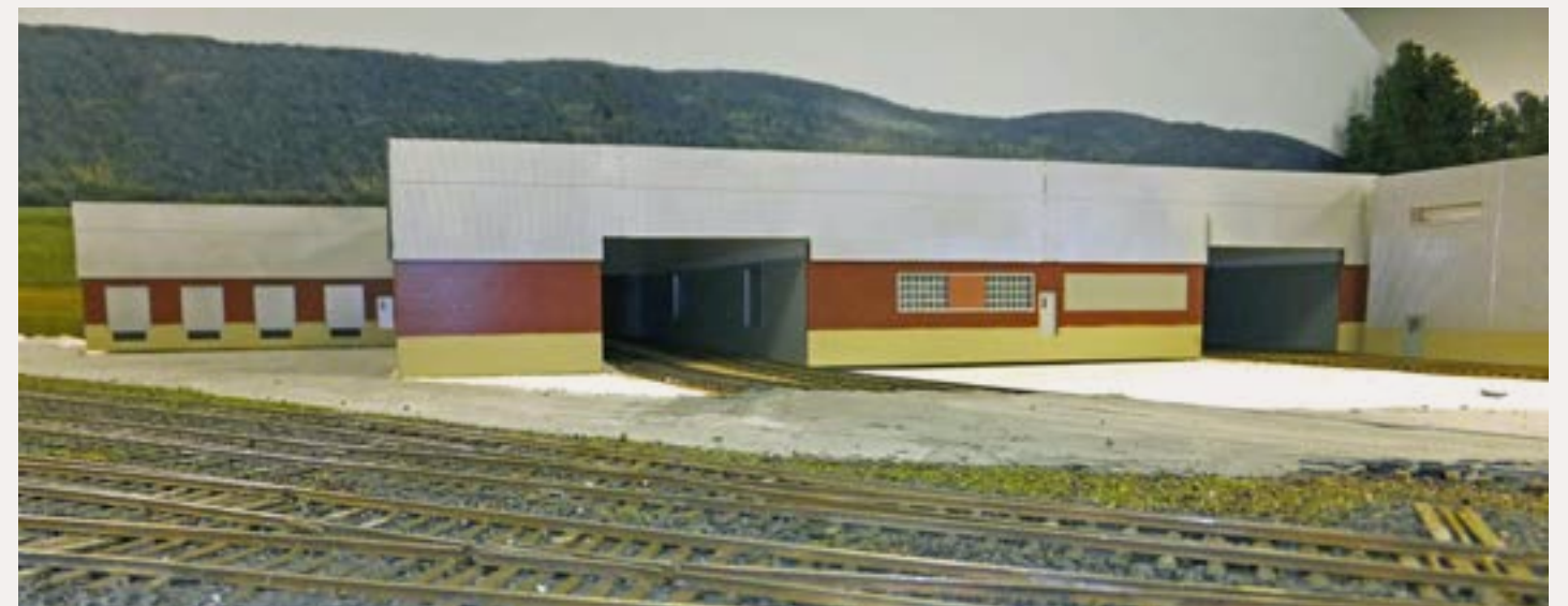
Figure 1V: The warehouse complex in a low angle shot from the front, taken with the camera in West Yard.
