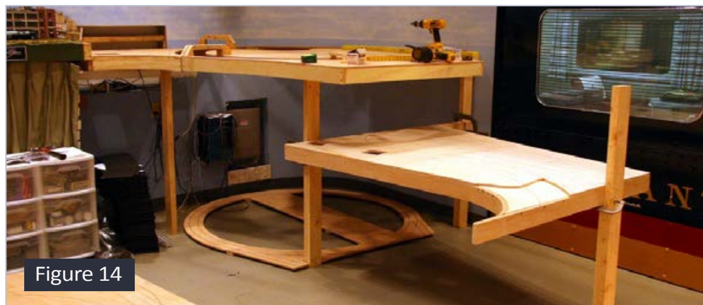
Figures 13-14: Placing the 2x4 legs, and the second level underneath.
