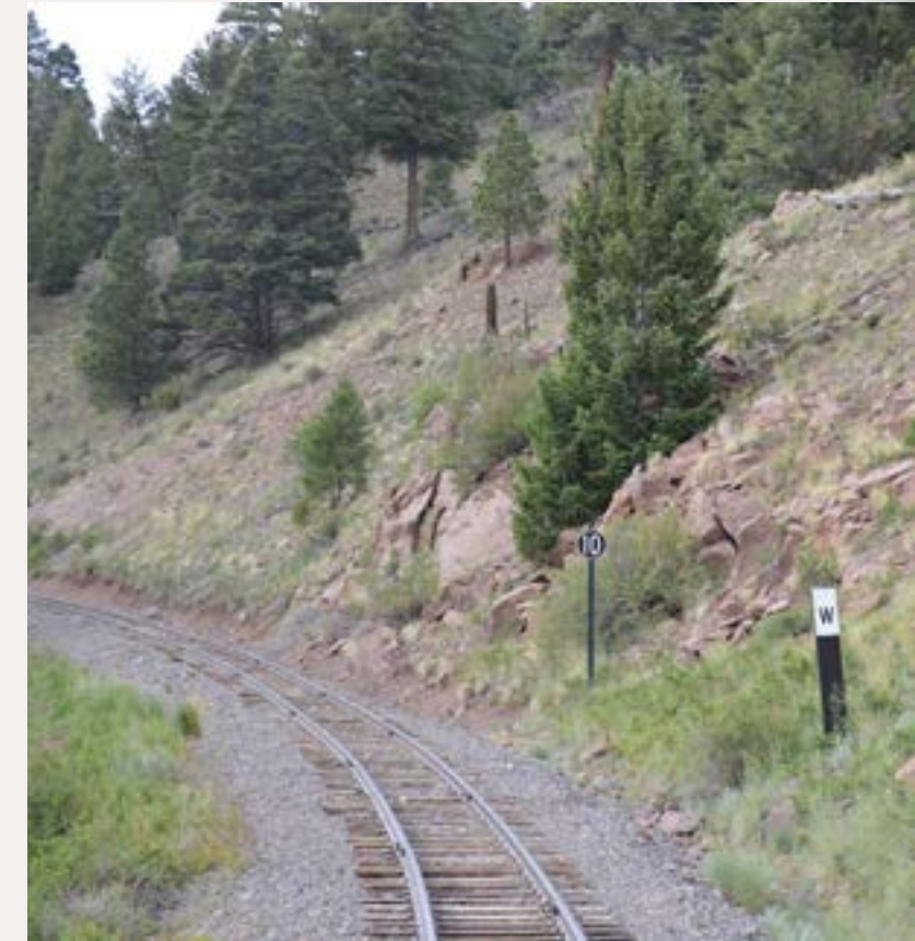
2: The “W” post on the Cumbres and Toltec Scenic Railroad [link: cumbrestoltec.com ] tells the engine crew they are approaching Mud Tunnel. The circular “10” sign is a speed restriction. Photo by Sharon Evans.
