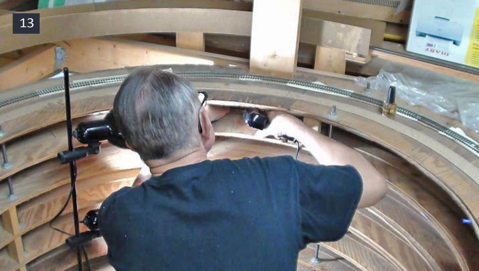
13: Phil solders new feeders into the Pineland helix.
