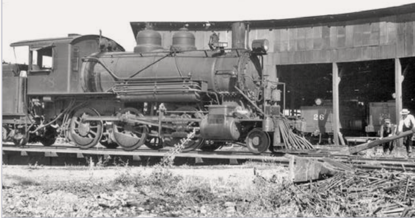
18: In this photo, the crew is turning the No. 28 on the turntable at Merced, probably around 1944 or so. But, what was also of interest to me is the pile of “junk” in the bottom right corner of the photo. The large wooden object is a sawhorse, not your typical carpenter sawhorse but a heavy-duty one. There are also some springs, most likely from freight car trucks, and a lot of scrap material. This pile of “stuff” shows up in some other prototype photos of the area. – Photo by Stanley Snook
