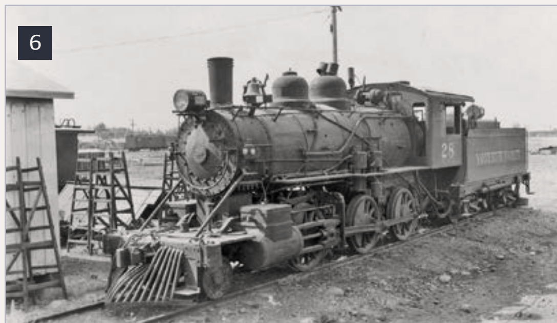
6: Another prototype photo provides a closer view of these details. While they might appear to be ladders, I finally realized that they were actually part of an early-day scaffolding system. These “ladders” were set up alongside a freight car with 2x8 or 2x10 boards inserted between the “steps” of the “ladders” to form the scaffolding needed to work on the upper portion of the car. They thus worked similar to current-day scaffolding systems.
