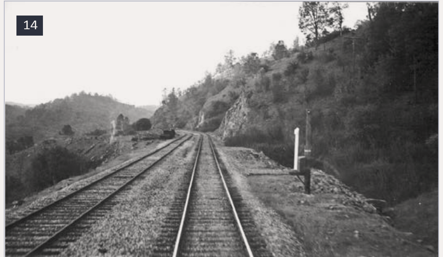
14: The YV switched from using telegraphs to telephones for transmitting Train Orders as of January 1, 1931. A few years later, the railroad began installing telephone jacks at a number of non-station sidings for the convenience of trainmen and other employees using portable phones. This photo shows the box sheltering the telephone jacks at a siding known as Starr on the YV. One of the Bulletins issued by the railroad noted that telephone jacks had been installed at a number of locations including Moss Canyon. Employee Timetables also indicated where telephones were available.
