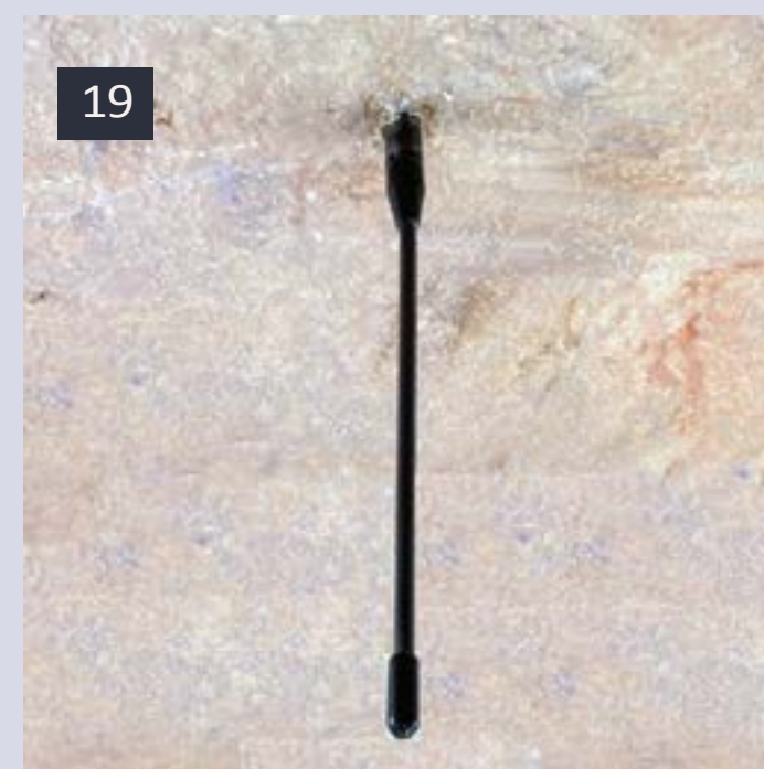
19: NCE RB02 through ceiling from below.
