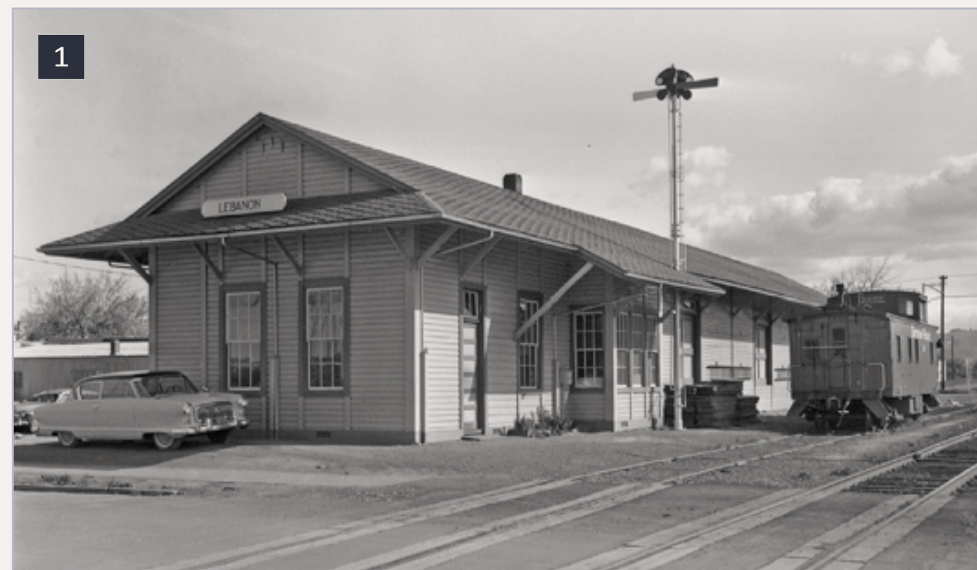
1: This is the Southern Pacific depot at Lebanon, Oregon, with an SP caboose standing on the house track (probably during a switching move). This depot shows the classic SP look, with its rectangular operator's bay, white window sashes, four-panel freight doors, and shingle roof. The depot was located on the East Side Line in Oregon, considered part of the Woodburn-Springfield Branch. (Shasta Division Archives.)
