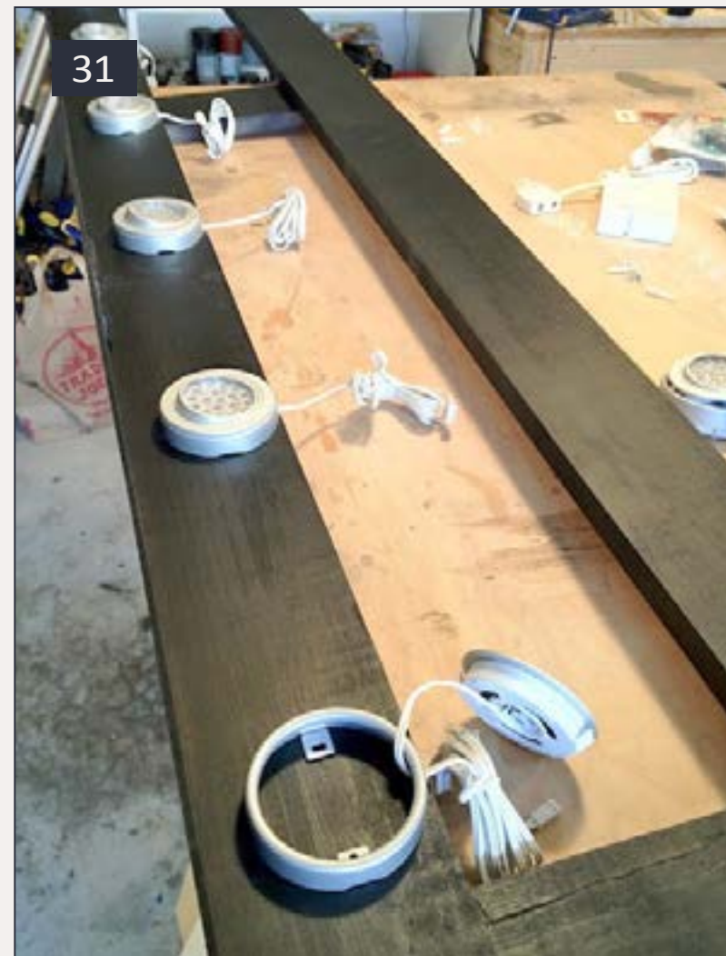
31: I installed two packs of Ikea "Inreda" LED pucks along the underside of the valence framework. They put out no heat whatsoever (which is good, since my garage already gets over 100 degrees F in the summer) and can rotate / adjust some to direct the light.
