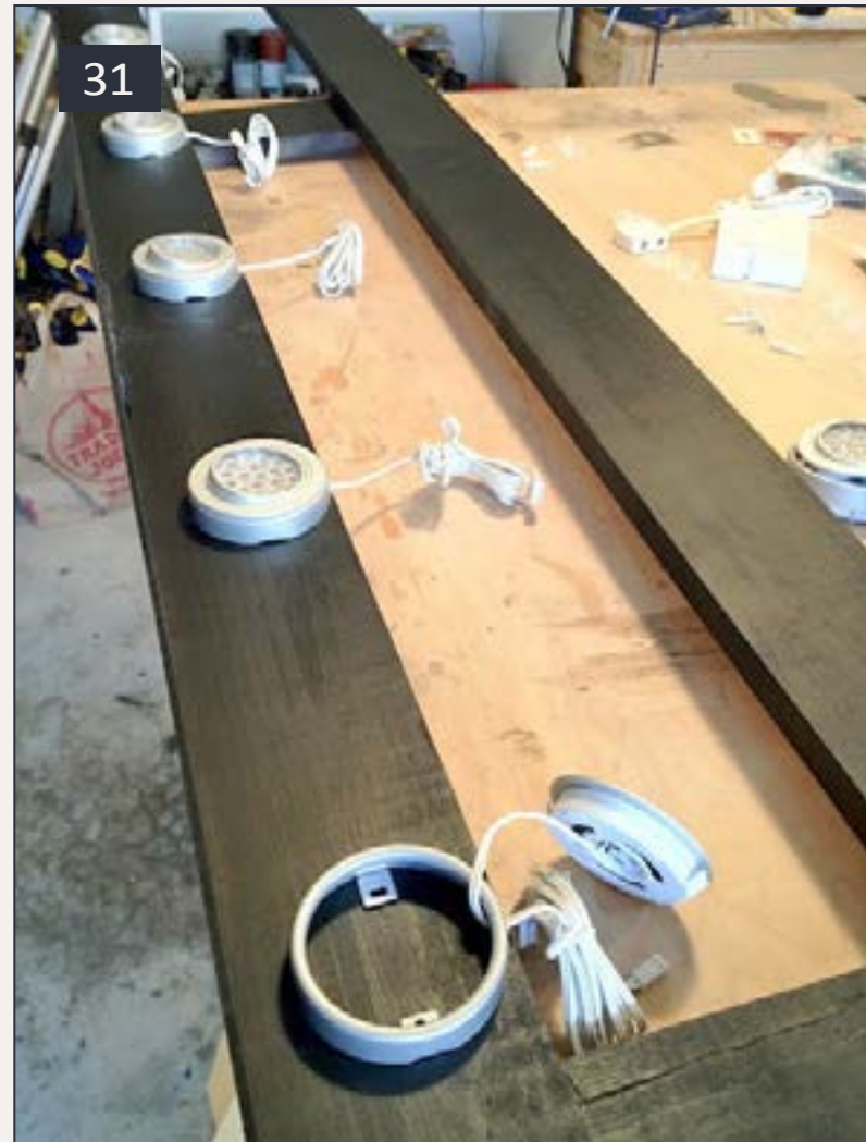
31: I installed two packs of Ikea "Inreda" LED pucks along the underside of the valence framework. They put out no heat whatsoever (which is good, since my garage already gets over 100 degrees F in the summer) and can rotate / adjust some to direct the light.
