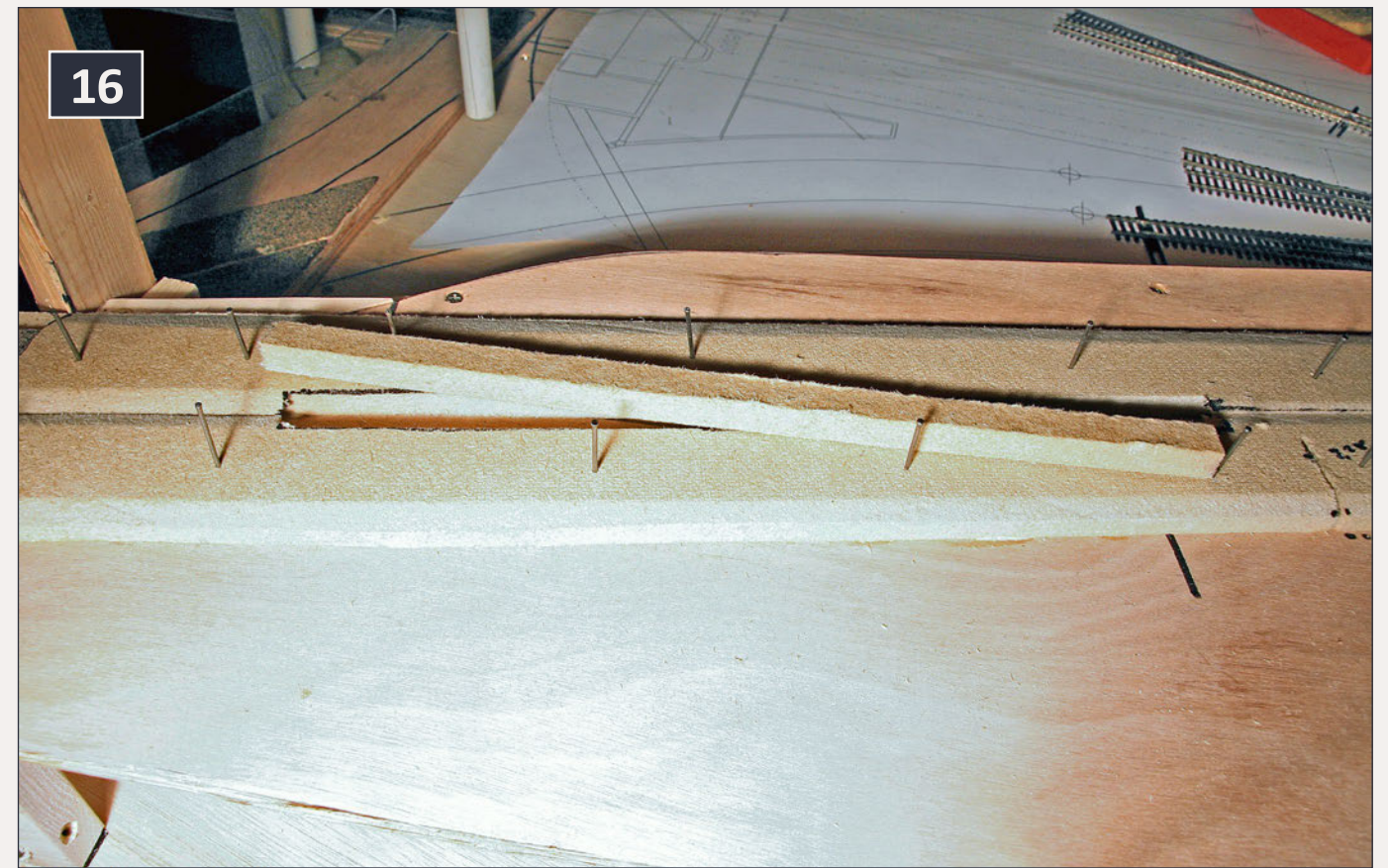
16: Special switch work.
