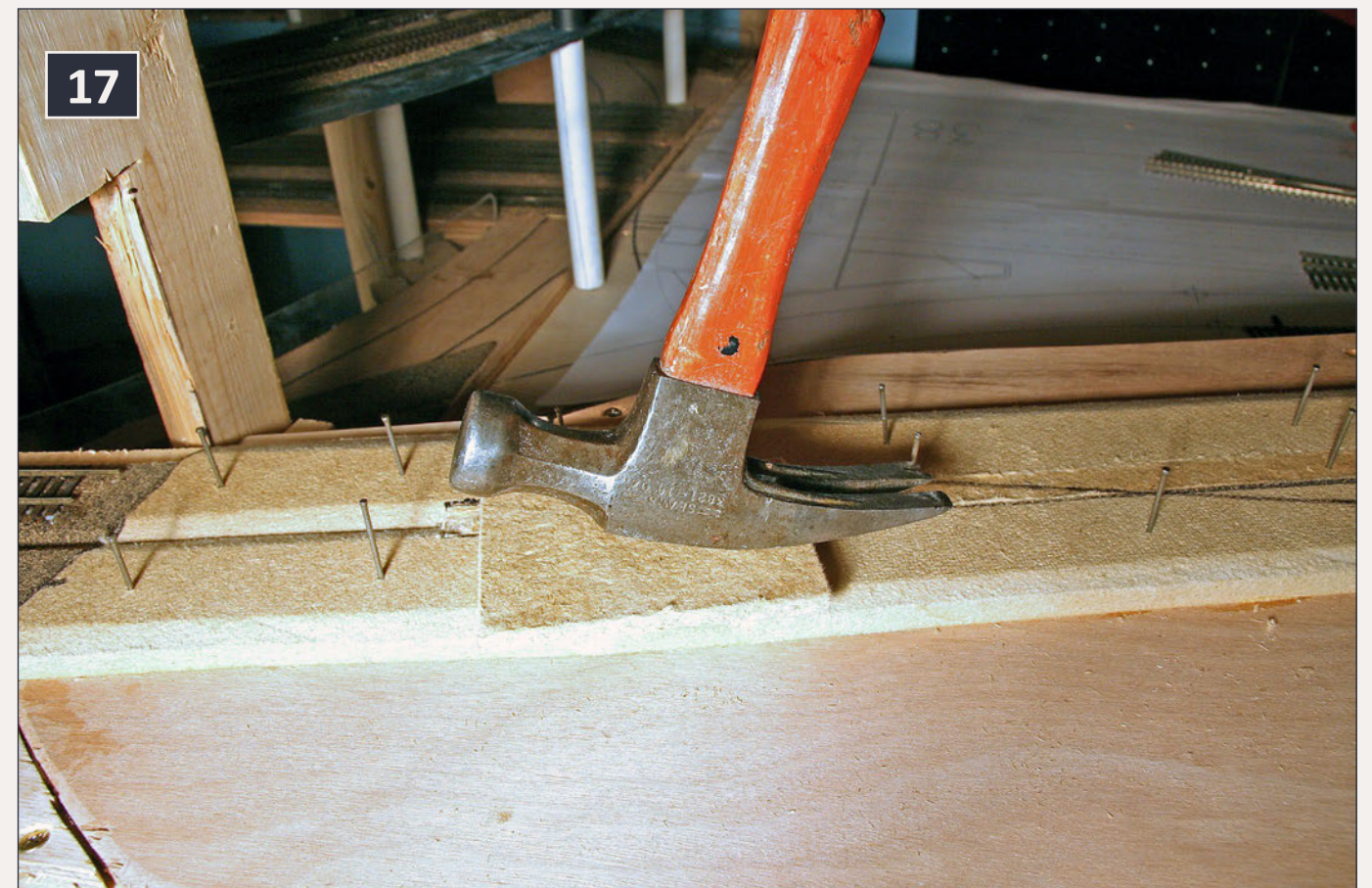
17: Removing the nails.
