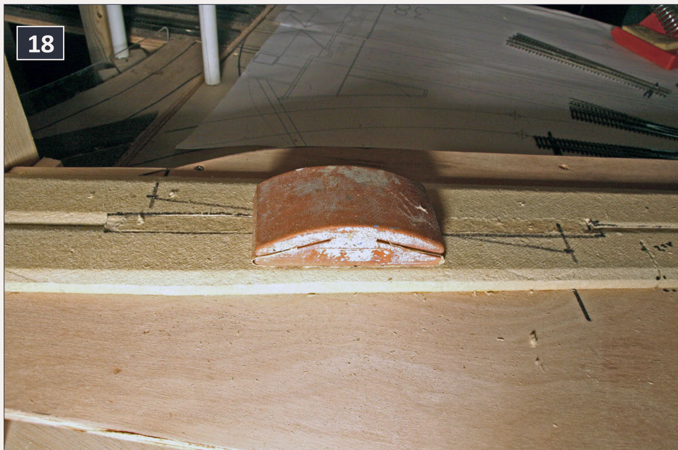
18: Sand the roadbed top smooth.
