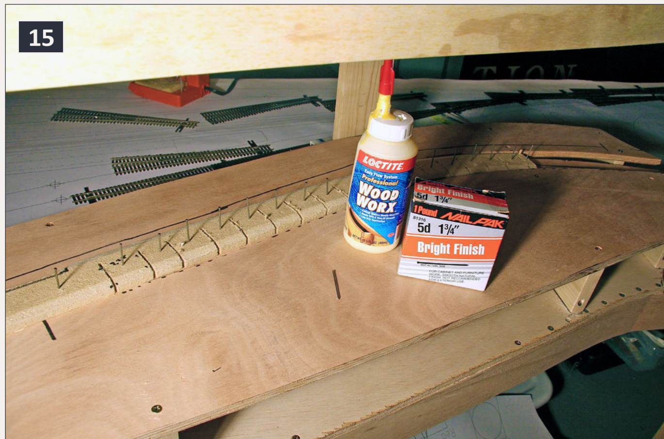
15: Laying the roadbed.
