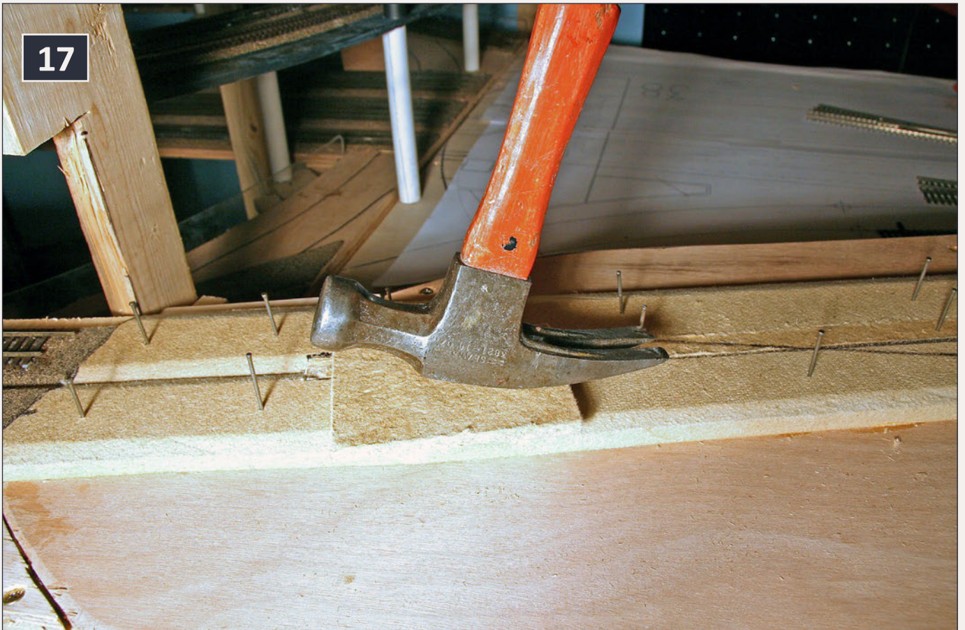
17: Removing the nails.
