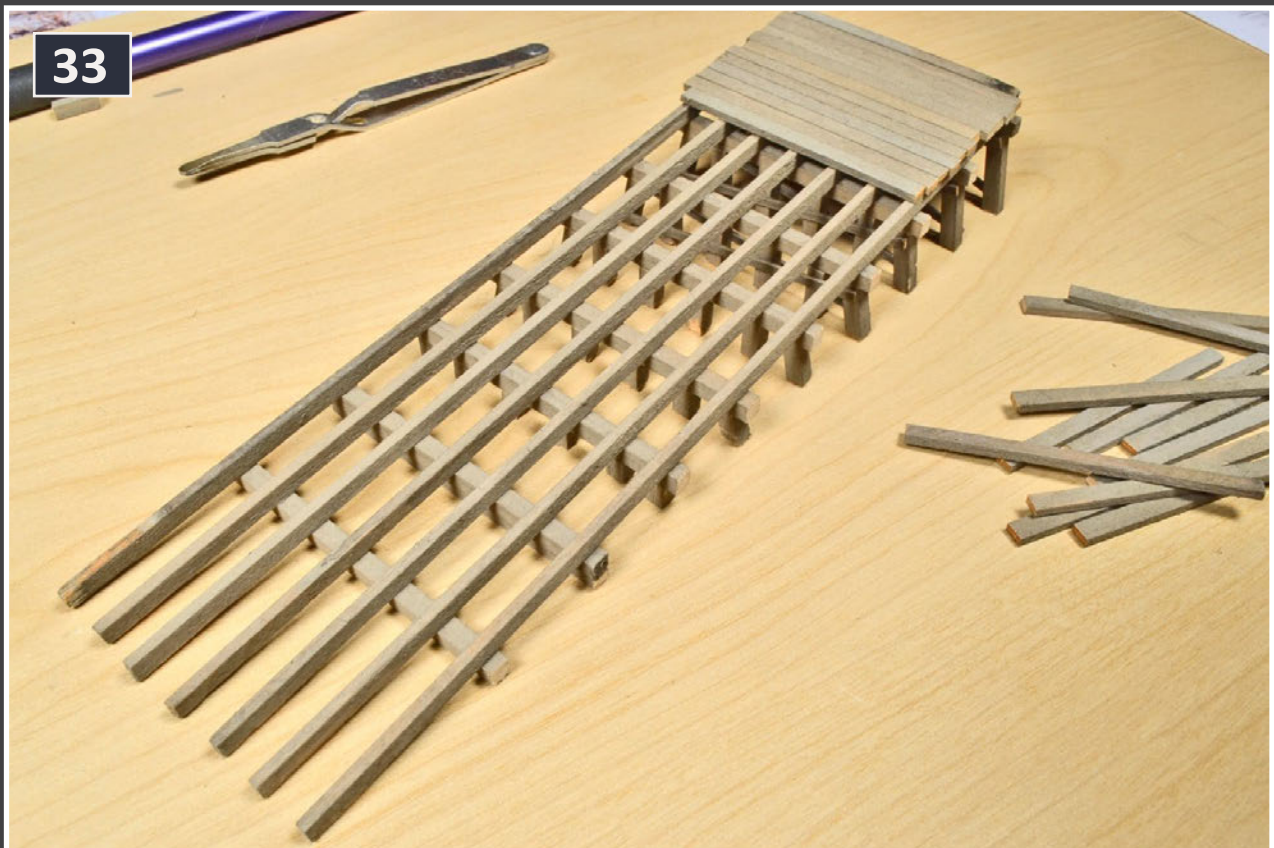
33: Installing the flooring on the ramp.
