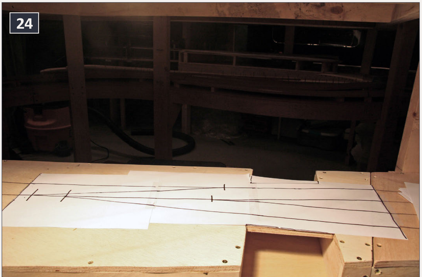
24: Paper pattern for complex roadbed section.
