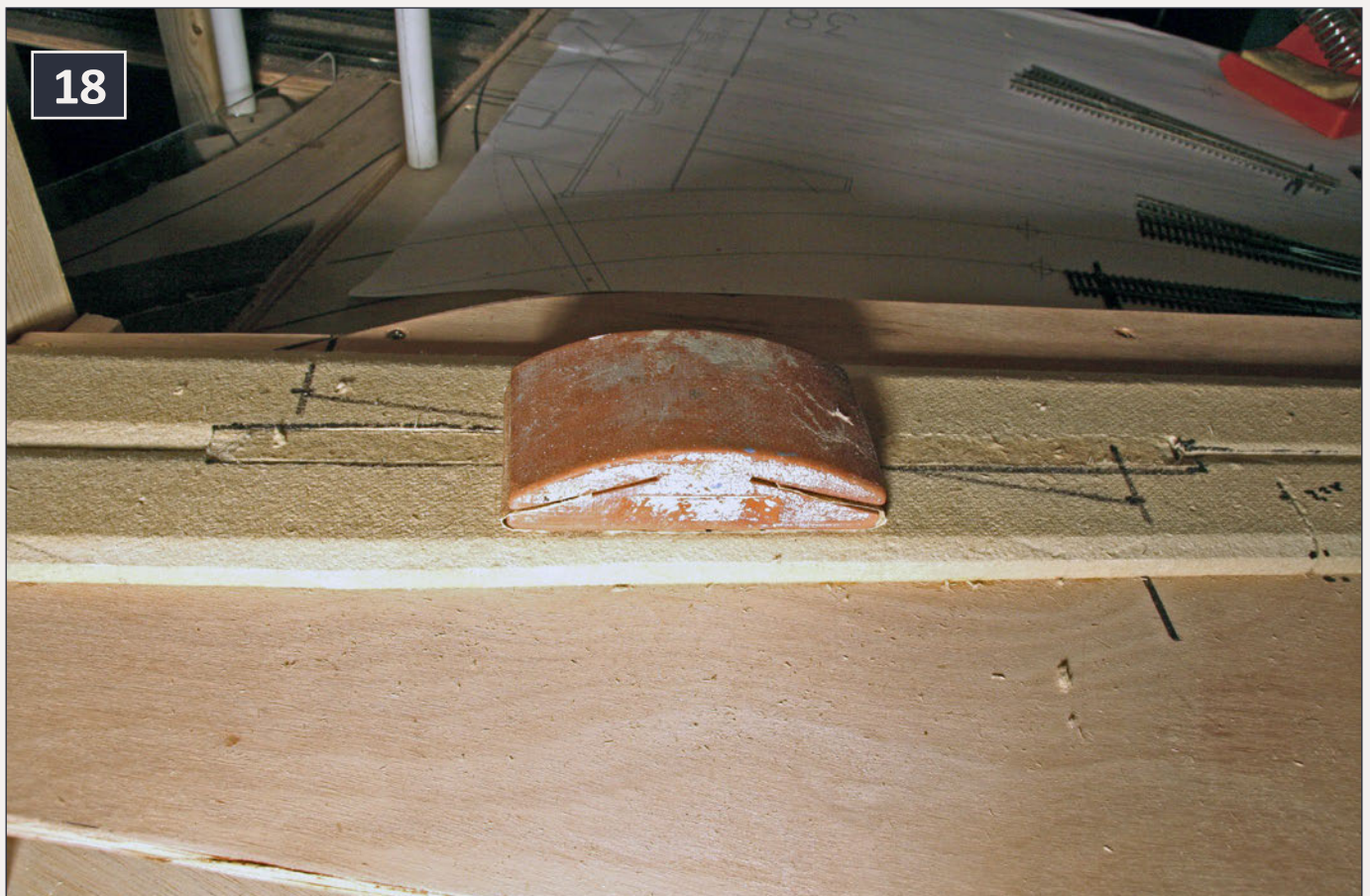
18: Sand the roadbed top smooth.
