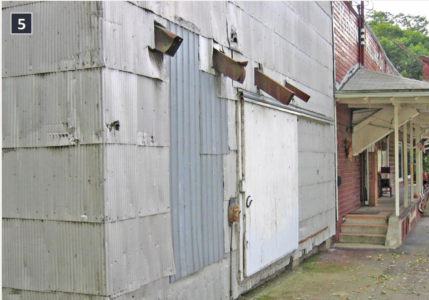
5: When you are scratchbuilding something like this, detail photos such as this (showing a close up of the siding, a patch job, the old sliding door, and the loading chutes) are invaluable.
