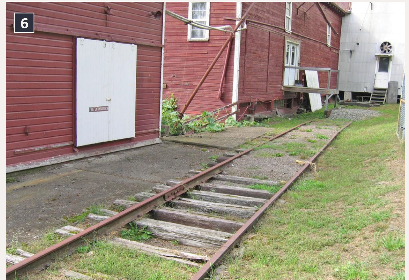
6: Here you can see the concrete that was part of the loading pit, now filled-in. It also looks like a truck dock has been built where rail cars once stood.
