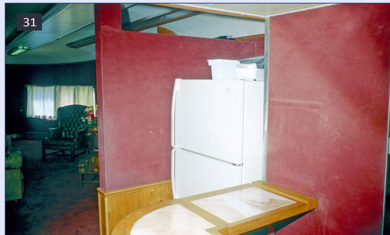
31: Where the wall was ripped out.
