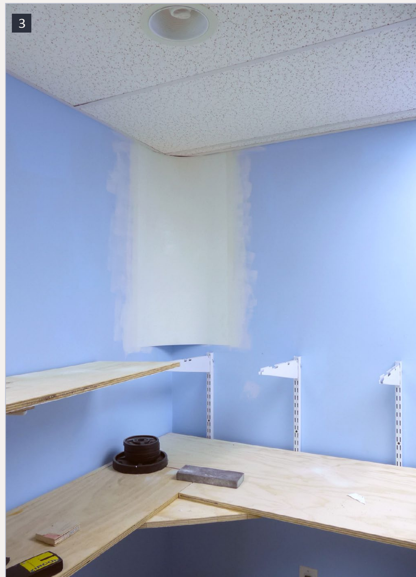
3. Hide the edges of the vinyl with two light coats of ready-mixed joint compound. Prime and paint.
