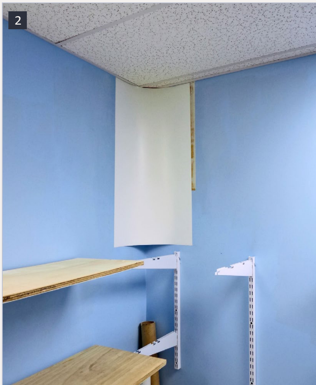
2. Cove base adhesive immediately holds the vinyl in place. Clean-up with soap and water.
