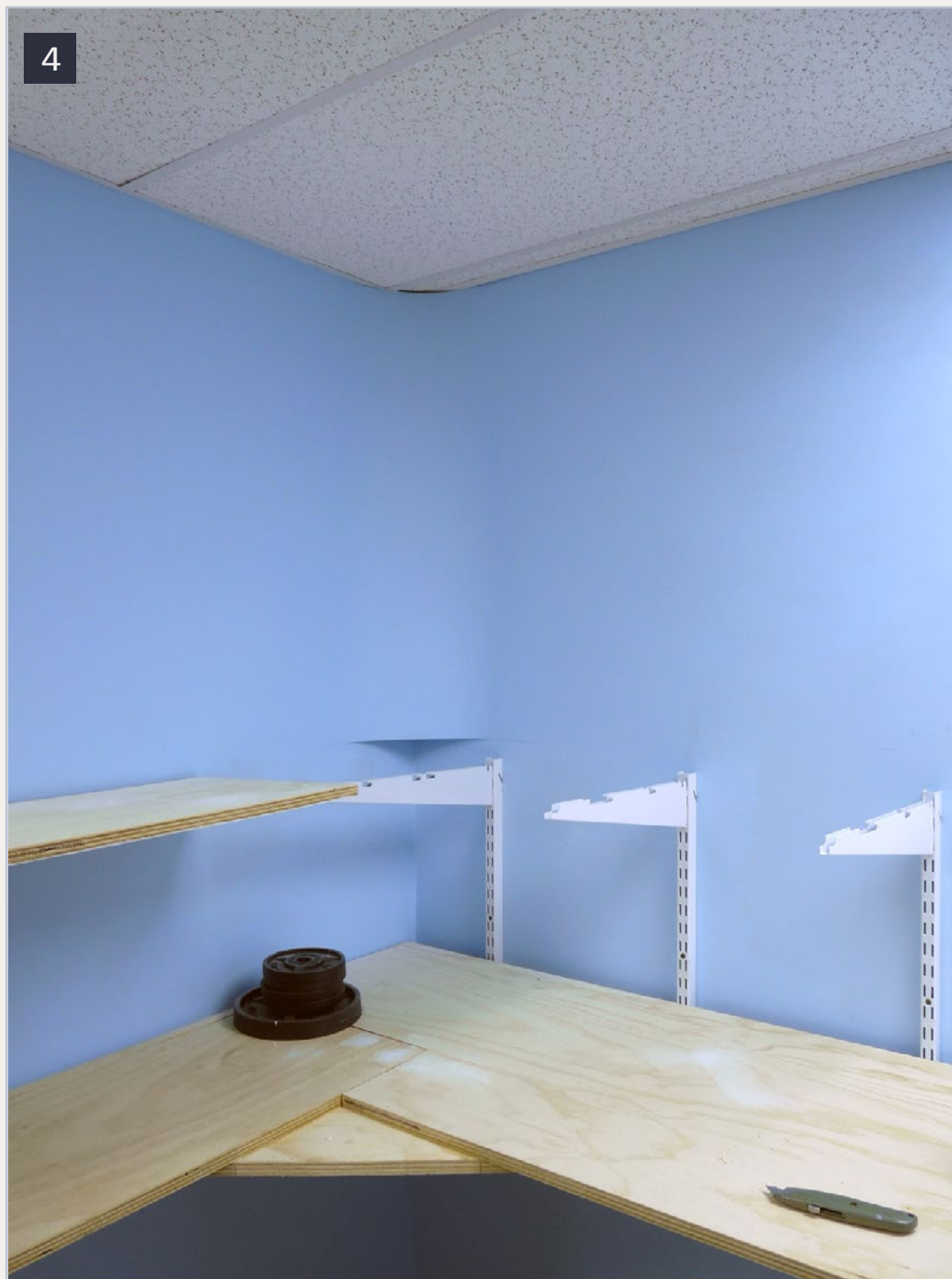
4. Notice where the wall and ceiling join: the radius is between 4 and 5 inches.
