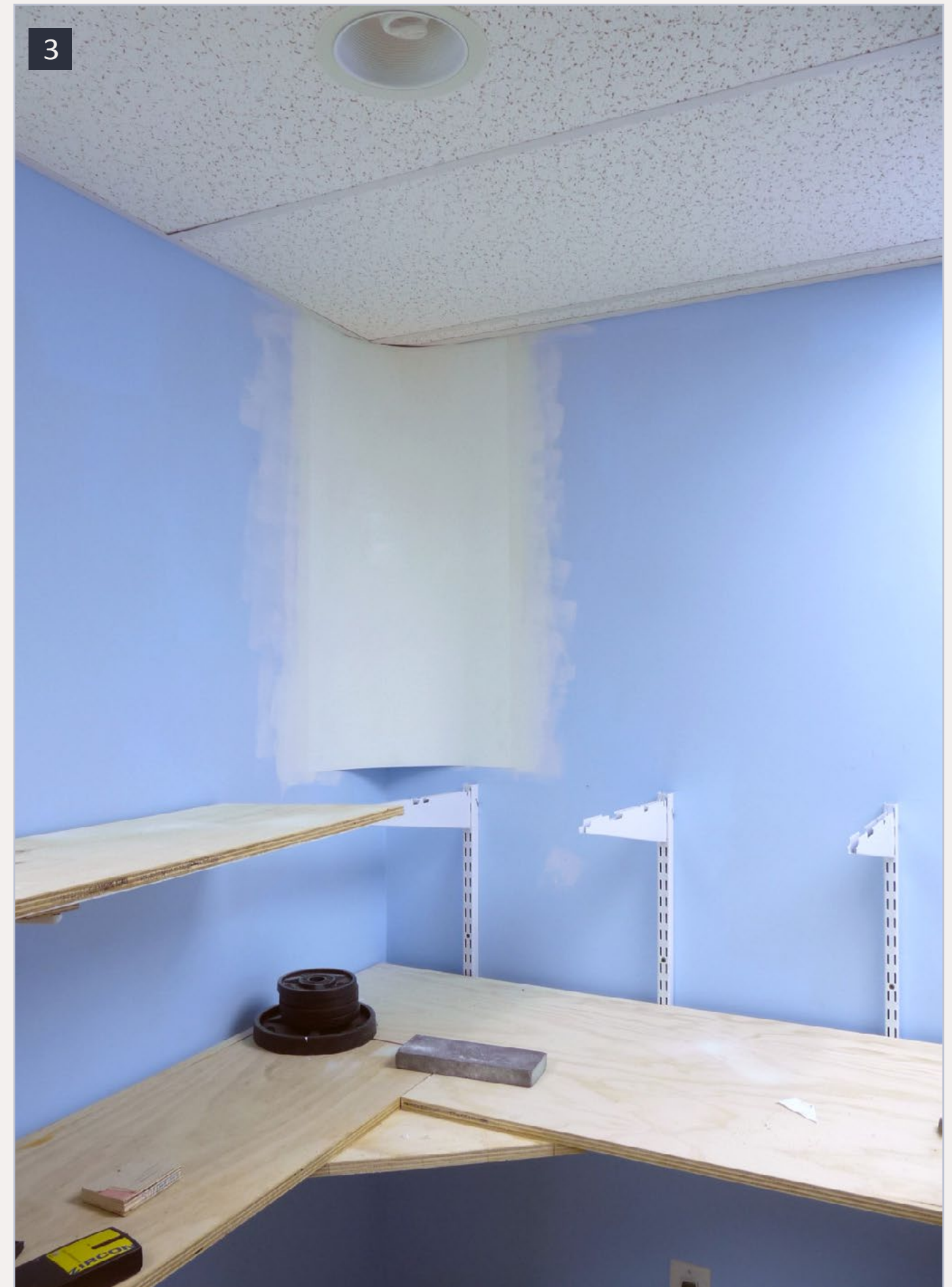
3. Hide the edges of the vinyl with two light coats of ready-mixed joint compound. Prime and paint.
