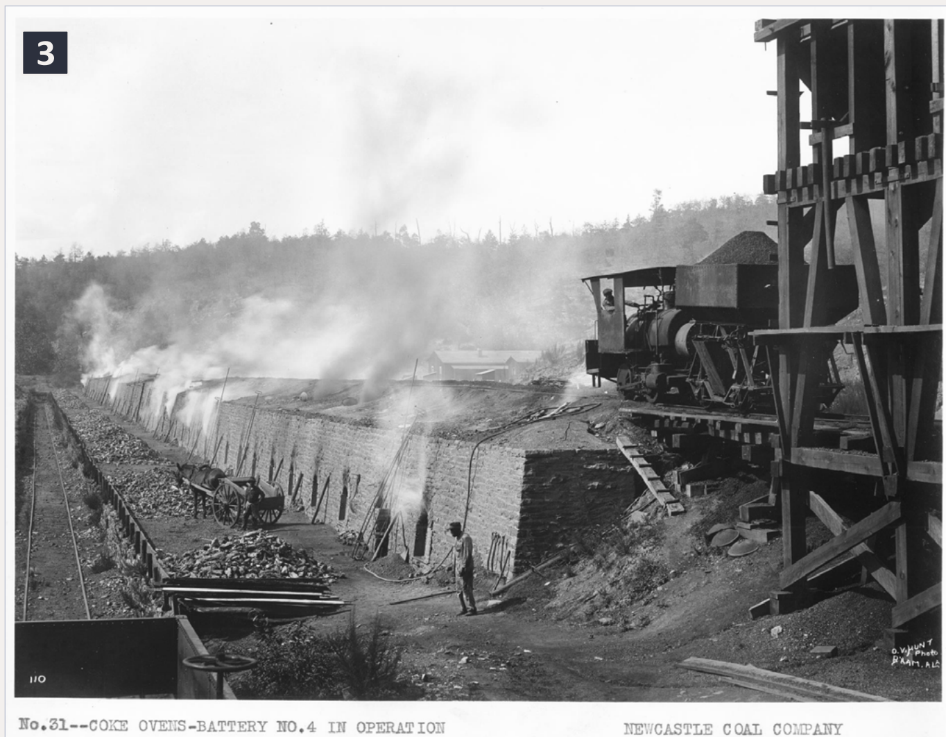
3: Coke Ovens Battery No. 4 of the Newcastle Coal Co. in operation at Newcastle, AL Courtesy of bham-rails.info from Ted McCormack Collection
