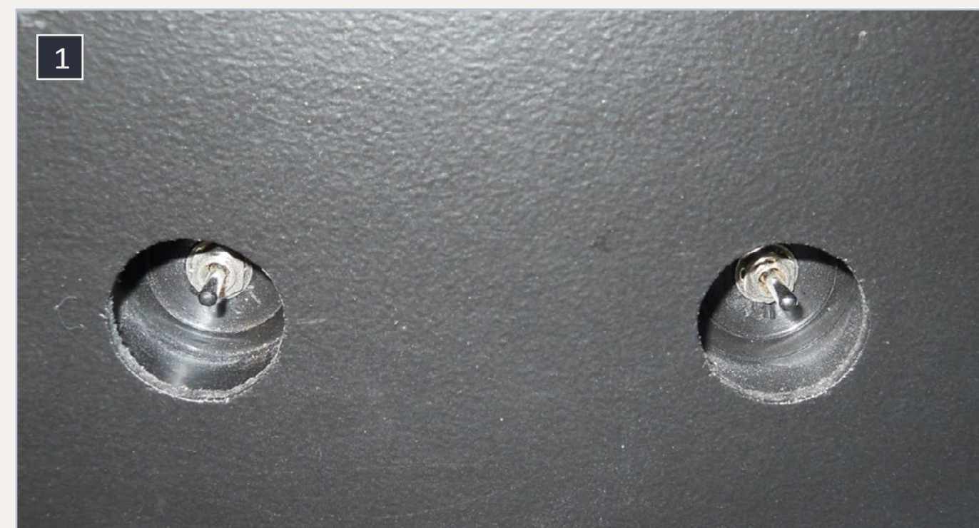
1: Recessed toggle switches are protected from damage and accidental use.
