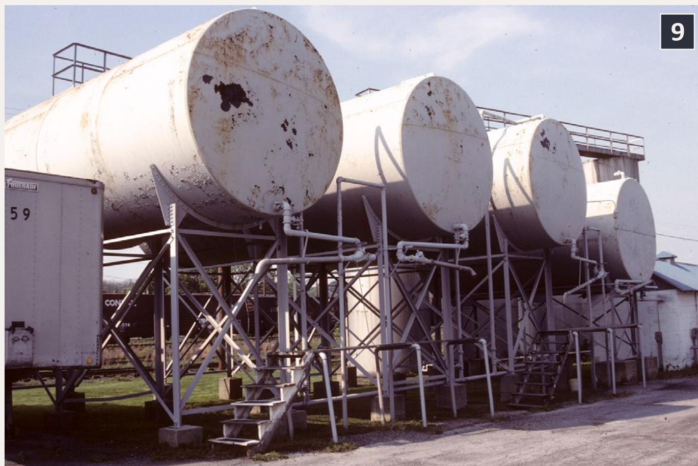
9: This oil dealer, in New Cumberland, Pennsylvania, was photographed in May 1985. The stairway leads to a minimal platform, and loading pipes come directly from tanks. In the background can be seen the top walkway on a four-tank set of vertical tanks. – Author photo.
