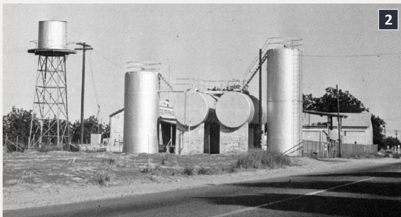
2: A Standard Oil of California bulk oil dealer in Waterford, California (east of Modesto). Here there are two vertical tanks, with two horizontal tanks between them, all painted silver. Barely visible behind the right-hand tank is a truck loading platform, and in the distance is the warehouse. This 1973 photo was included in the April 1996 Railmodel Journal article listed in the Bibliography. – Robert Schleicher photo.
