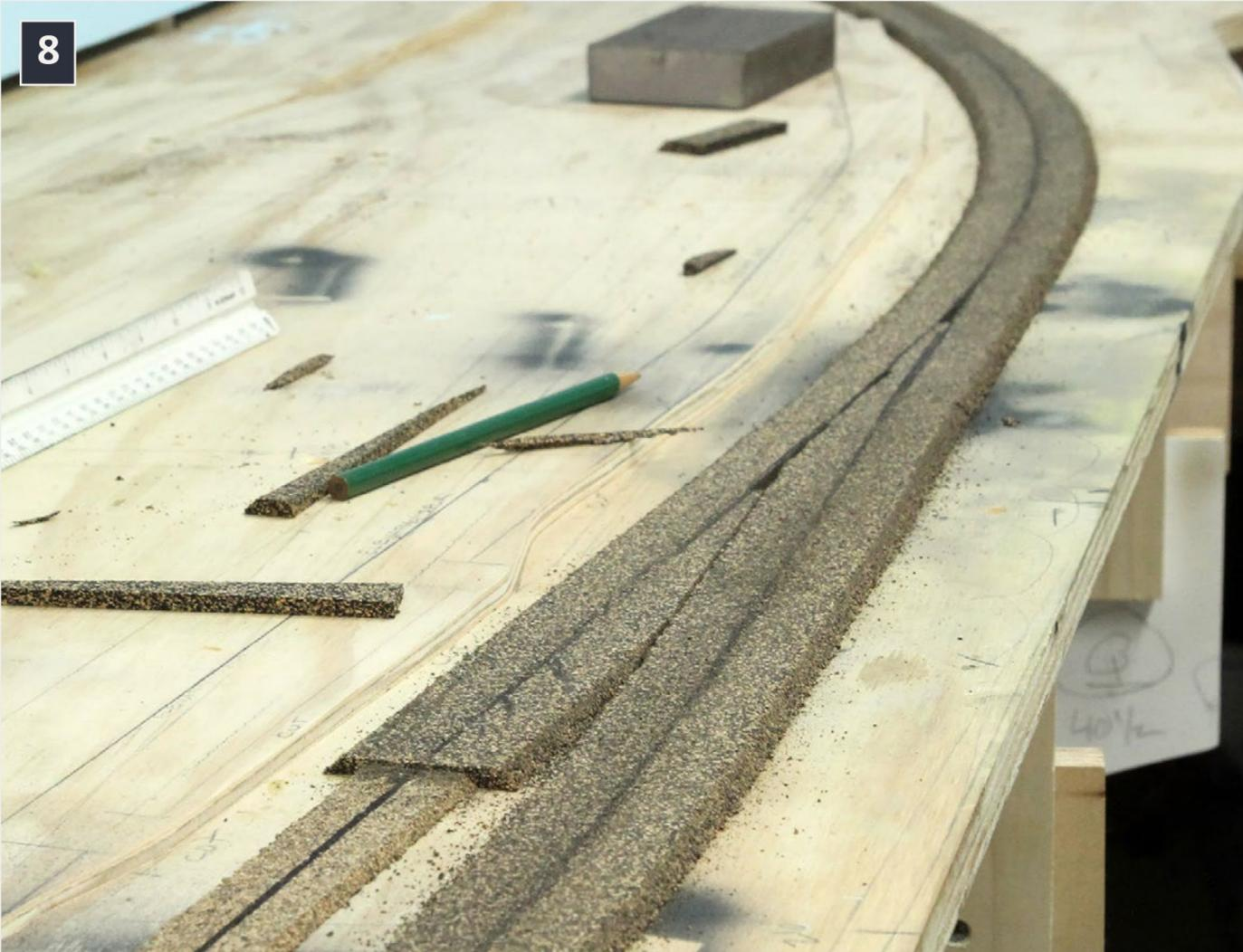
**8. The center seam in the cork roadbed is clearly visible even after the cork has been sanded.**
