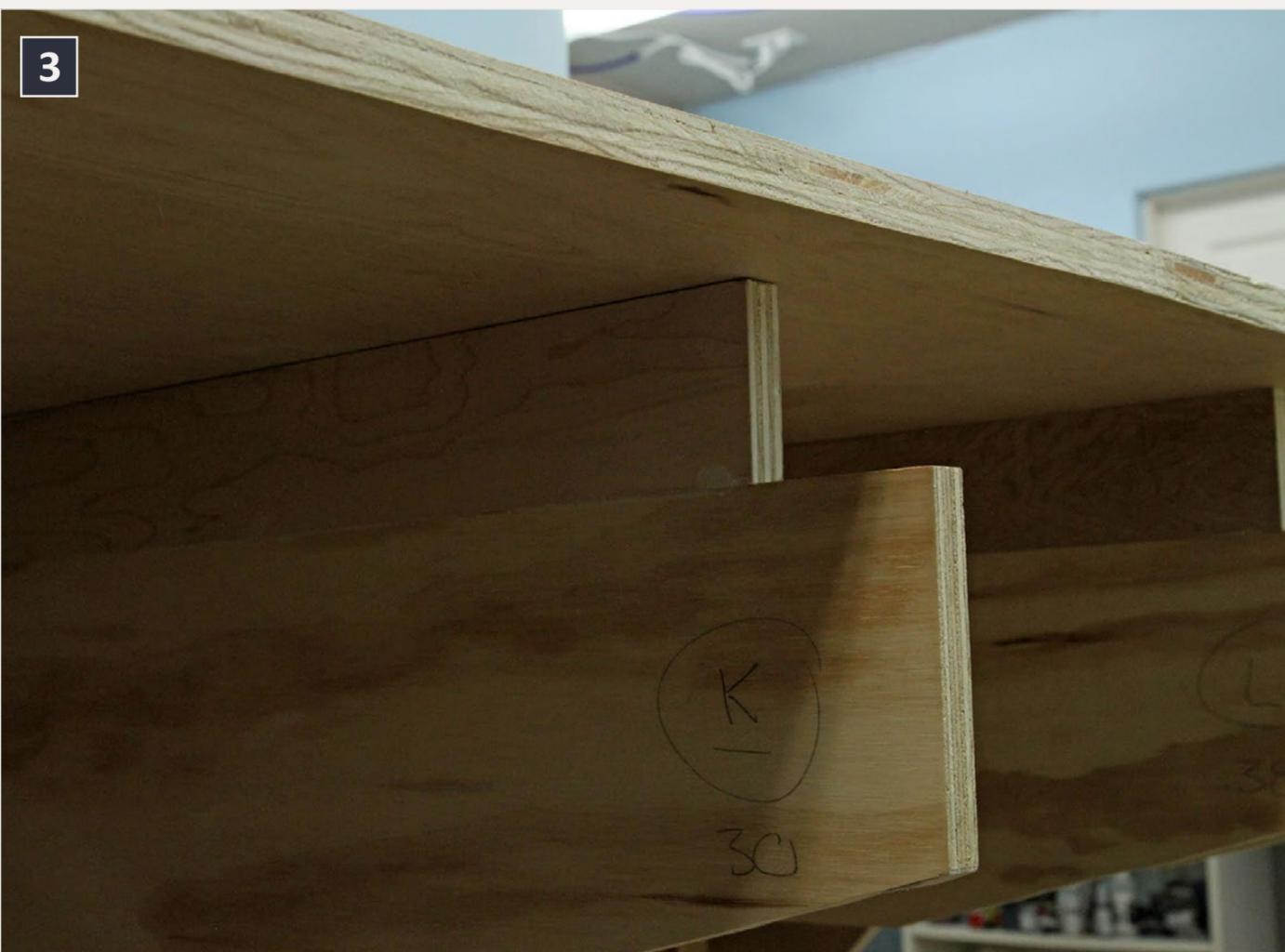
**3. 2-3/4" auxiliary joists riding on top of the Browning supports raise the plywood sub-roadbed to the correct height. They're attached with Liquid Nails. I set the auxiliary joists back from the edge to make room for a creek which will border the fascia in places.**
