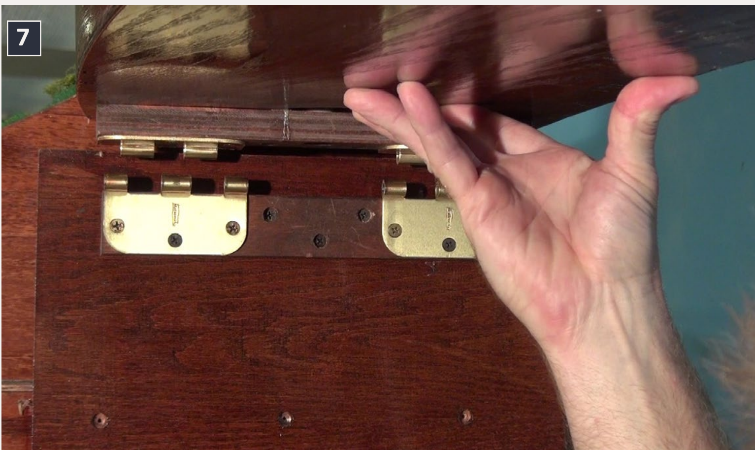
7. Remove the hinge pins and lift the section to separate the hinge parts. See how the hinge mounts fit together.
