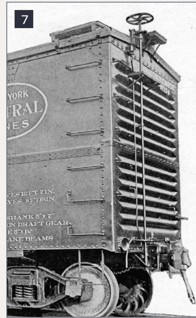
7. ACF builder's photo of 36' steel car built in 1912 with 7-7 Murphy end. Note lack of end ladder.
