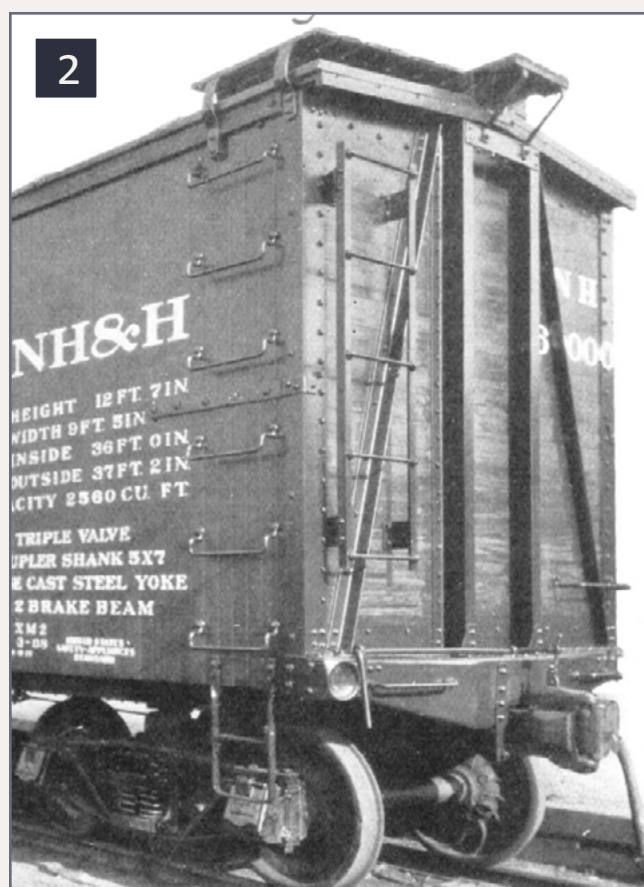
2. 1908 car rebuilt in late 1920s with heavy vertical steel bracing augmented with lighter L-sections angled inward from the lower corners. Note overhanging roof.
